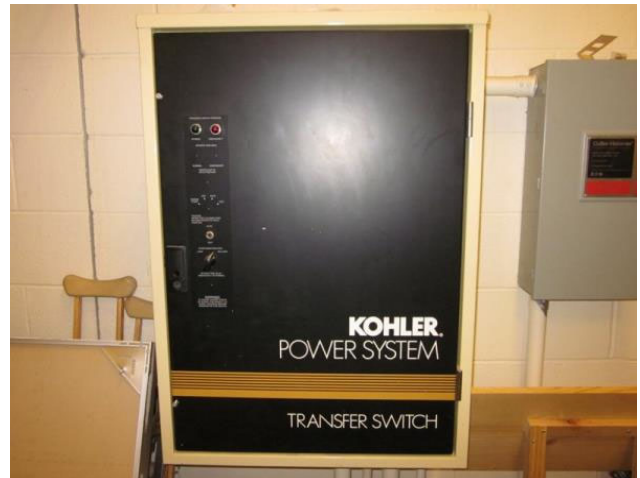
28 - EMERGENCY GENERATOR AUTOMATIC TRANSFER
