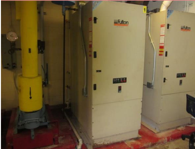
19 - BOILER NUMBER 1, FULTON PULSE BOILER 6/23/14
