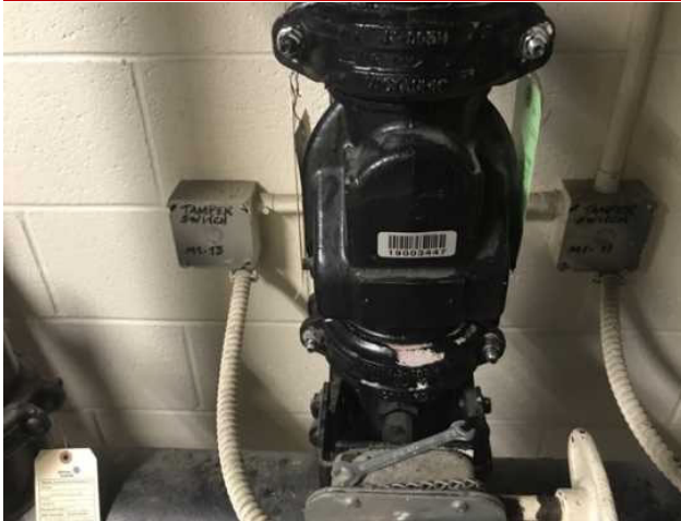
25 - FIRE RISER, WET STANDPIPE
