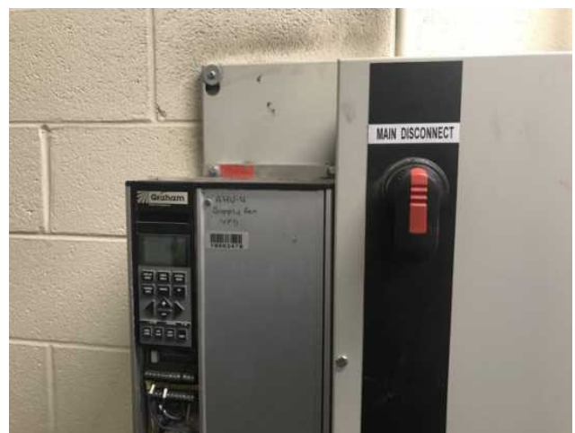
30 - VARIABLE FREQUENCY DRIVE, VFD
