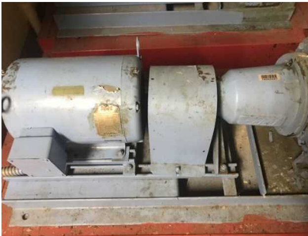
21 - PUMP, DISTRIBUTION, HVAC HEATING WATER
