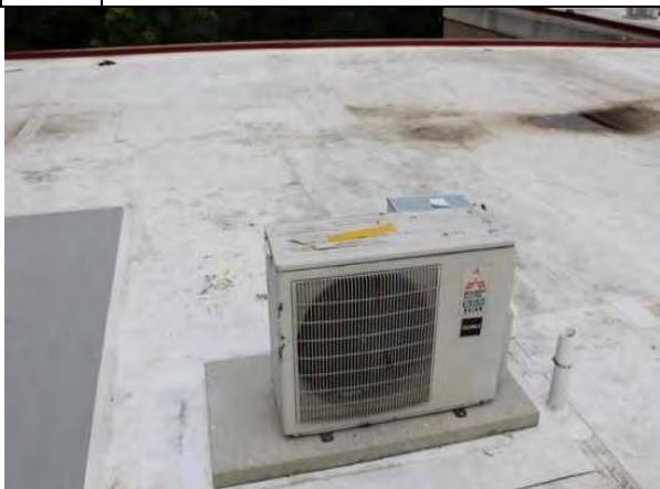
#29: SPLIT SYSTEM DUCTLESS
