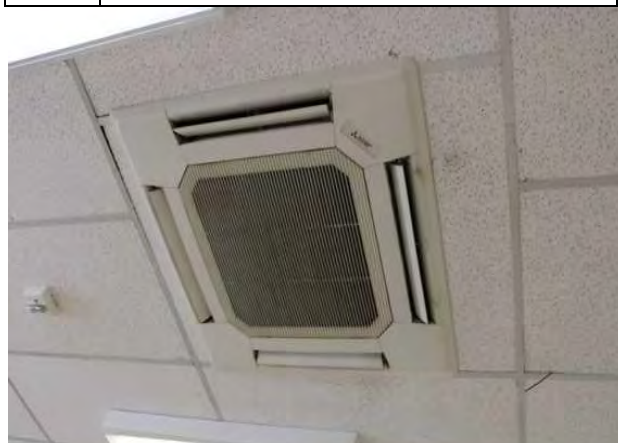
#30: SPLIT SYSTEM DUCTLESS
