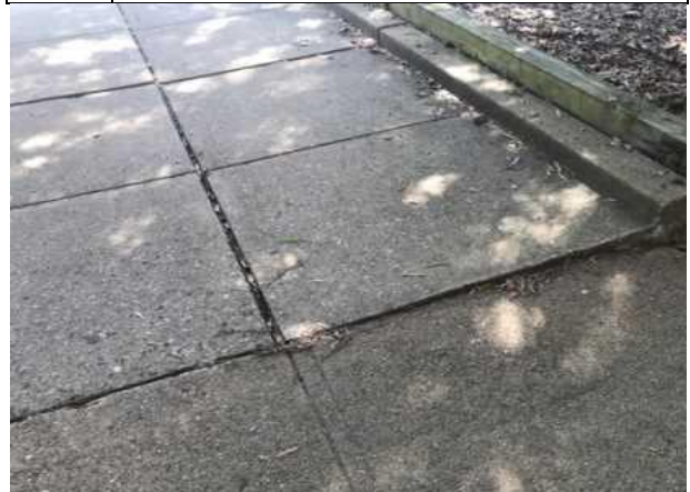
#22: TRIP HAZARD ON SIDEWALK
