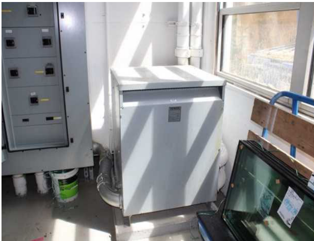
39 - SECONDARY TRANSFORMER
