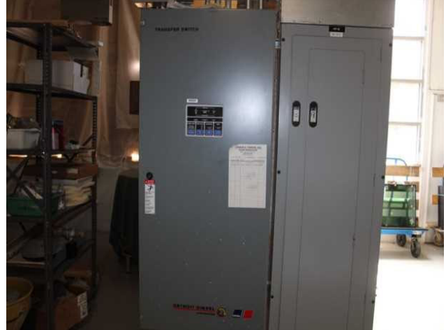
38 - AUTOMATIC TRANSFER SWITCH
