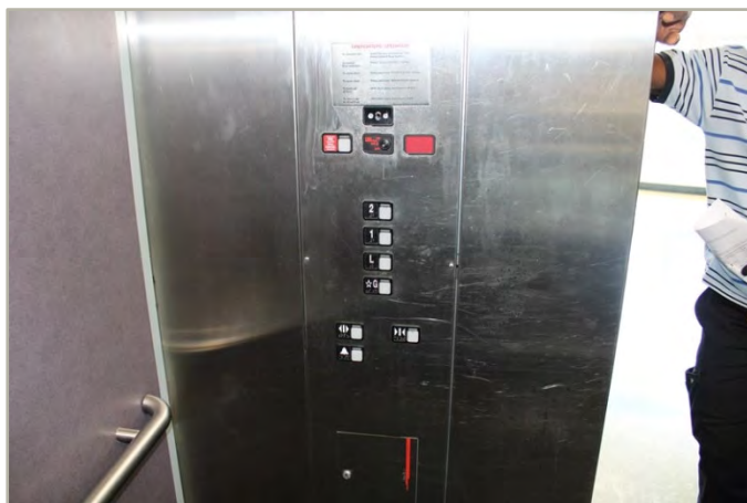
10 - IN-CAB CONTROLS/EMERGENCY CALL PANEL
