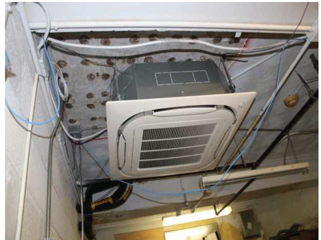
28 - SPLIT SYSTEM DUCTLESS
