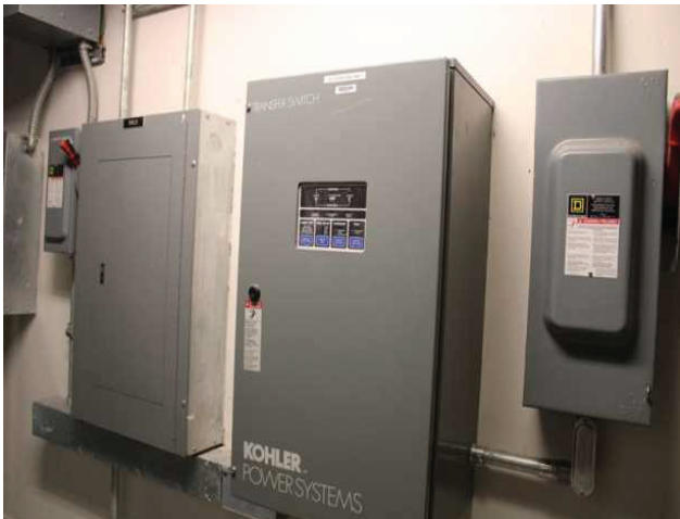
33 - AUTOMATIC TRANSFER SWITCH
