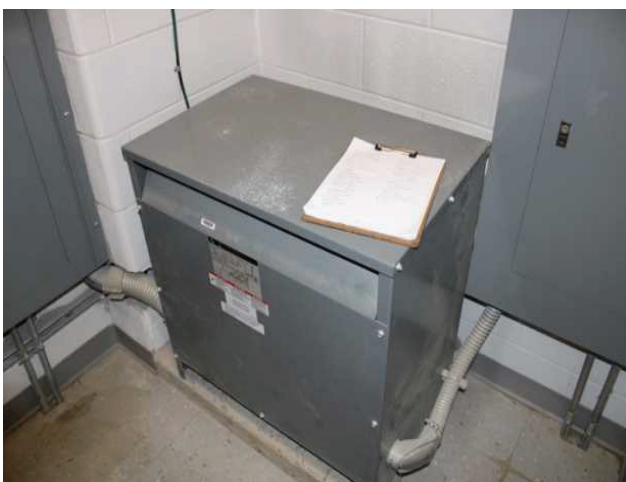
35 - SECONDARY TRANSFORMER
