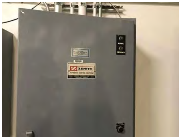
28 - AUTOMATIC TRANSFER SWITCH - ATS
