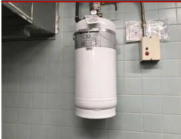
31 - FIRE SUPPRESSION SYSTEM, COMMERCIAL KIT
