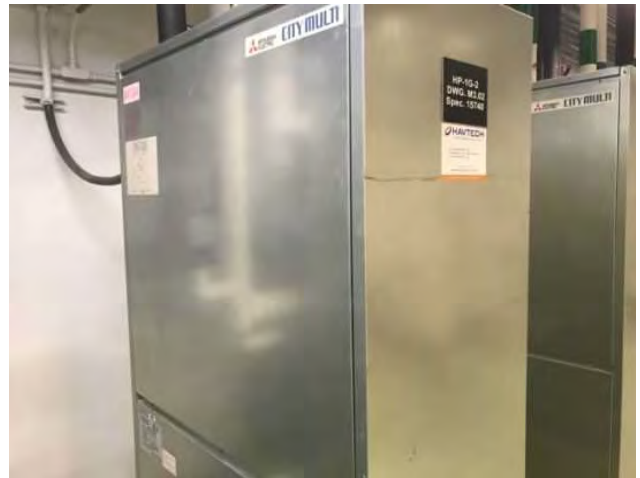
16 - WATER SOURCE HEAT PUMP
