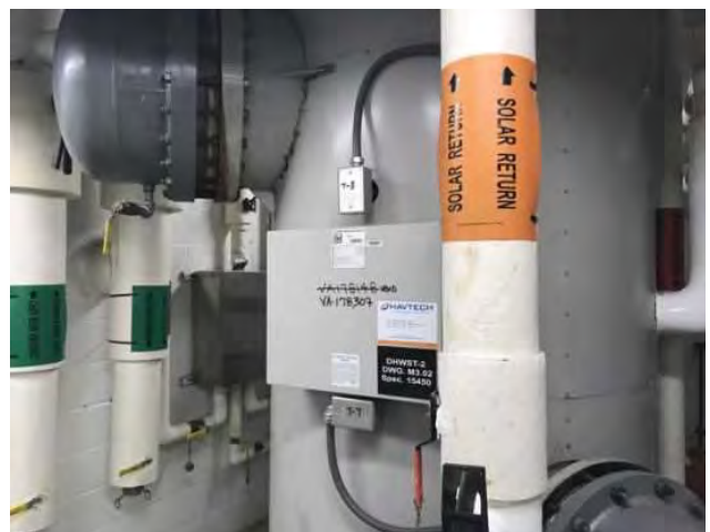
18 - STORAGE TANK, DOMESTIC WATER
