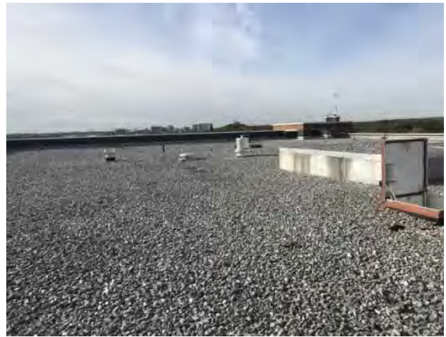
4 - ROOFING, BUILT-UP
