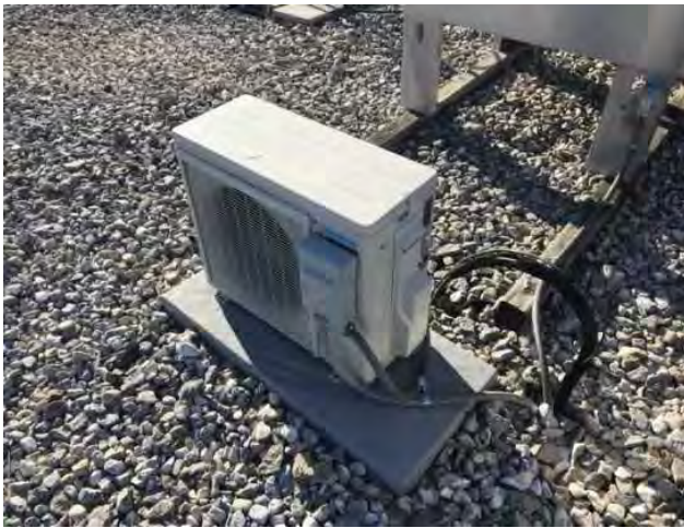
21 - SPLIT SYSTEM DUCTLESS
