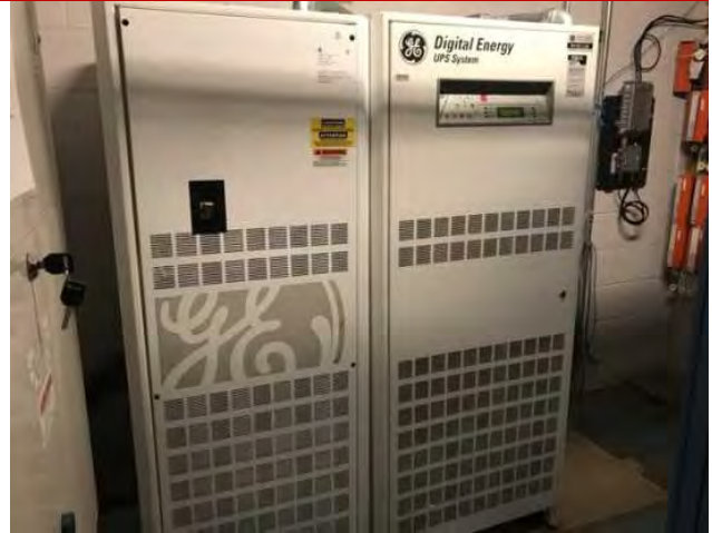
32 - UNINTERRUPTIBLE POWER SUPPLY, UPS
