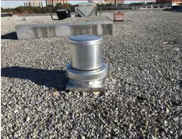
25 - EXHAUST FAN, CENTRIFUGAL
