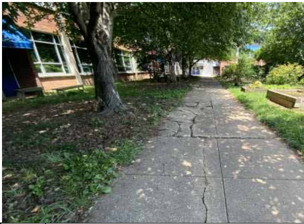
#13: DAMAGED SIDEWALKS
