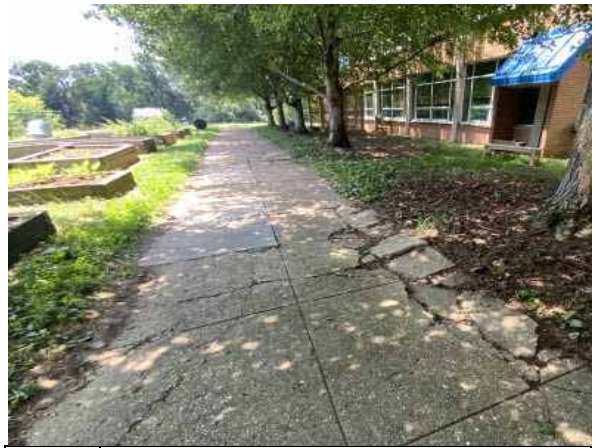
#14: DAMAGED SIDEWALKS
