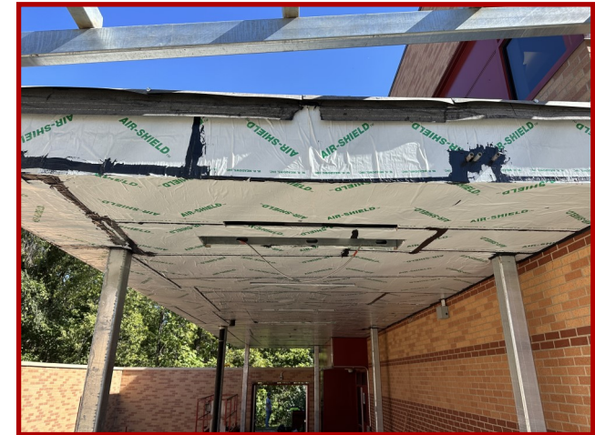
Waterproofing at Addition Canopy
