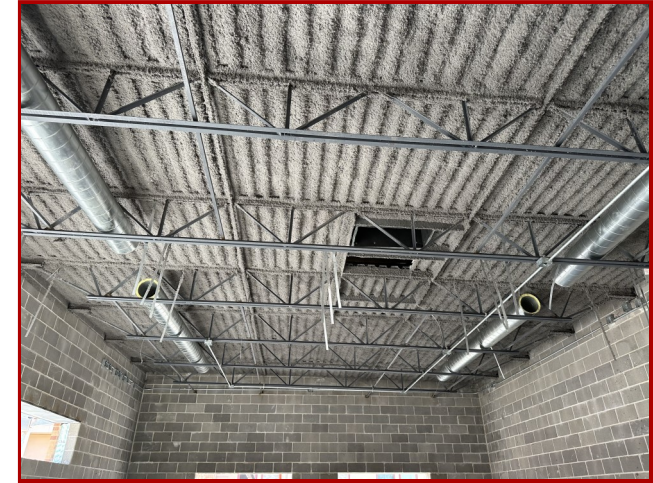
MEP Rough-In at Addition Ceiling
