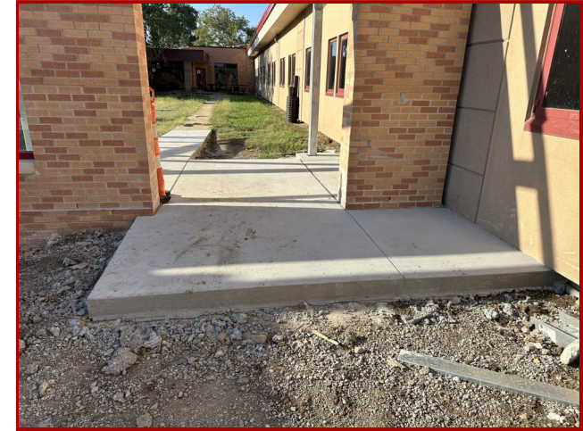
Concrete Sidewalk at Addition
