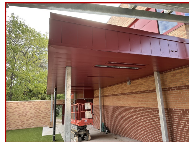
Metal Panels at Addition Canopy
