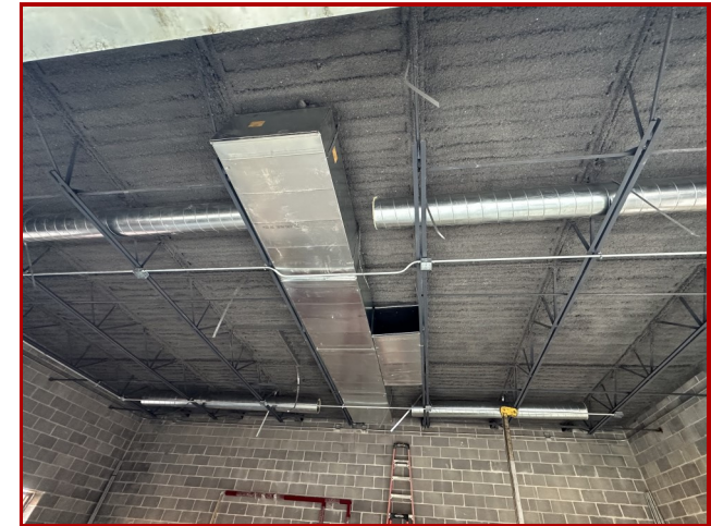
MEP Rough-In at Addition Ceiling
