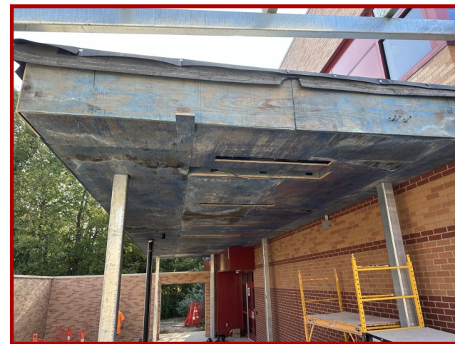
Plywood Sheathing at Addition Canopy
