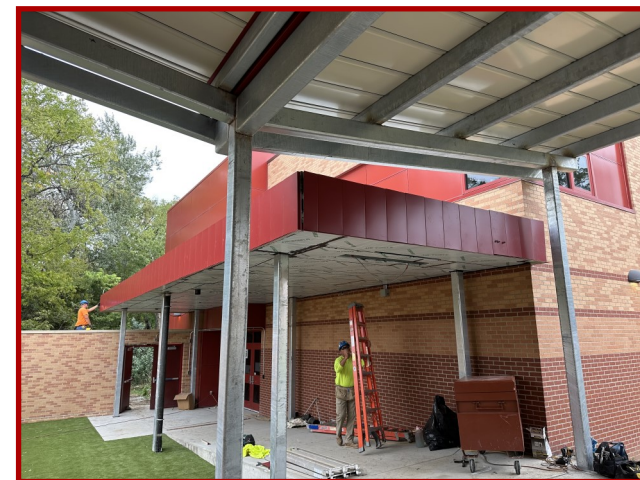
Metal Panels at Addition Canopy
