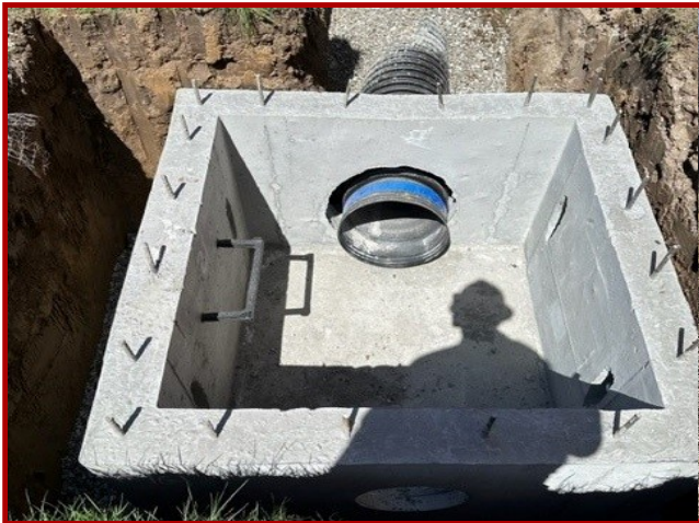
Installed Storm Structure
