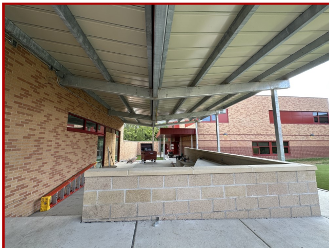
Metal Panels at Addition Canopy
