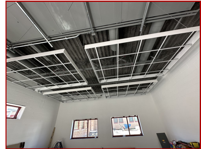
Acoustical Panel Ceiling Clouds
