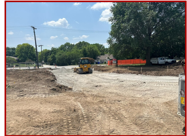
Existing Bus Loop Grading
