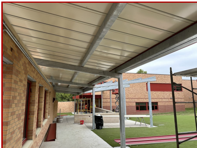
Metal Panels at Addition Canopy
