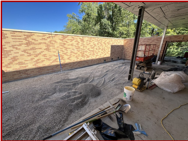
Prep for Turf at Addition
