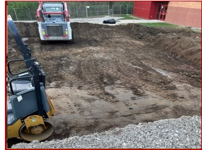
Grading for Foundations
