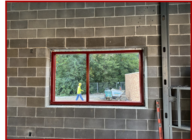
Addition Storefront Window Framing
