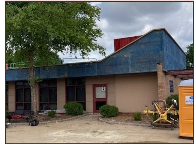
Exterior Framing & Sheathing at Front Office
