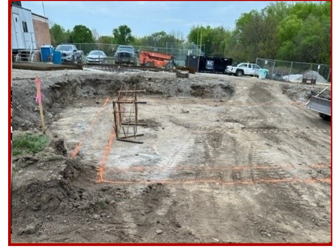
West Footing Layout at Addition
