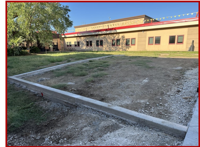
Concrete Curb in Courtyard
