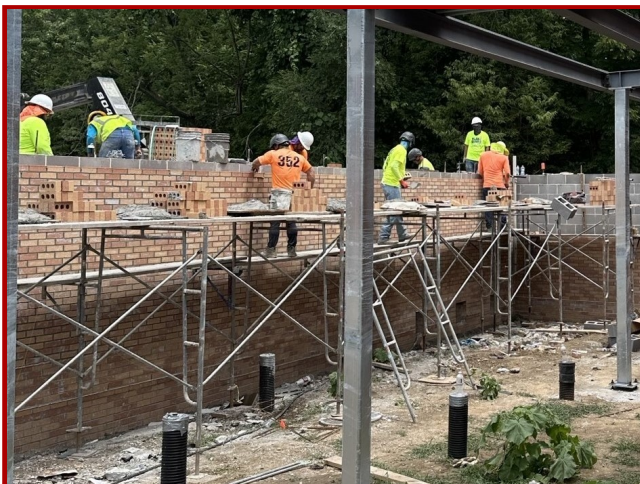
Masonry on Courtyard Walls
