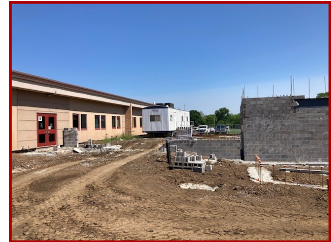
Leave-out Section to Finish Courtyard
