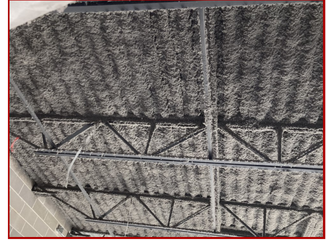
Spray Insulation at Addition Ceiling
