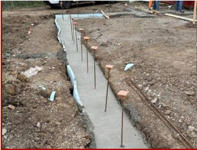
Poured A Line Footing
