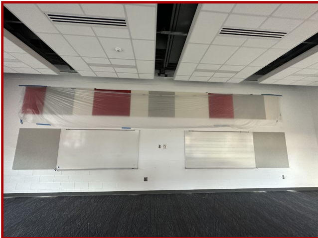
Acoustical Wall Panels in Auxiliary Classroom
