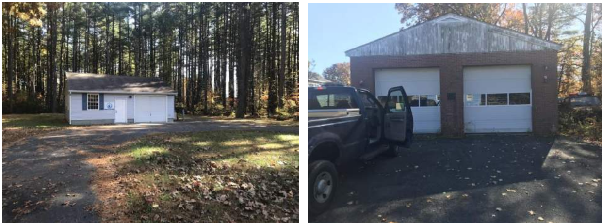
Figure 1. Water supply interconnection building and driveway on Pequot Road (left) and old Fire Department building and driveway on Bluemer Road (right) (October 2019).
