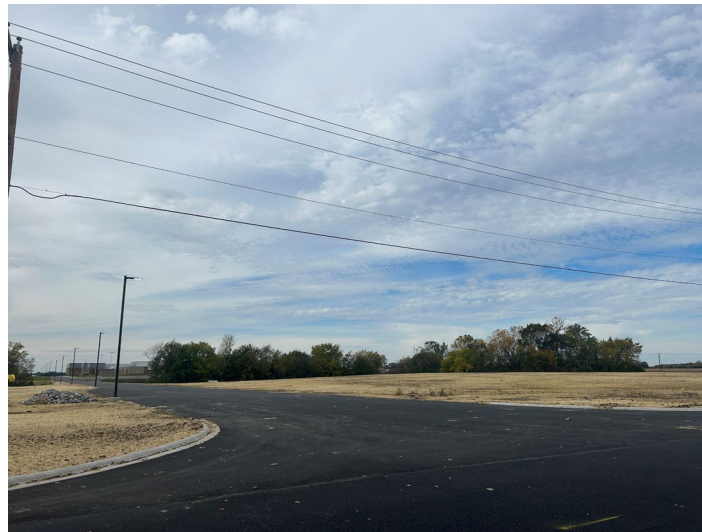
South Entrance Road
