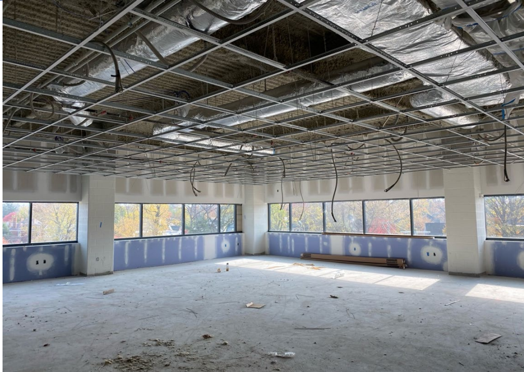
Ceiling Grid Being Installed on the 4th Floor
