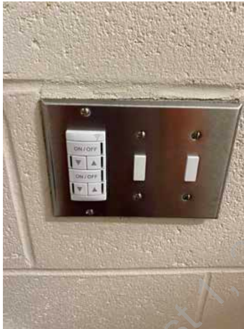
● D2. 5: Electrical Lighting Control Station
