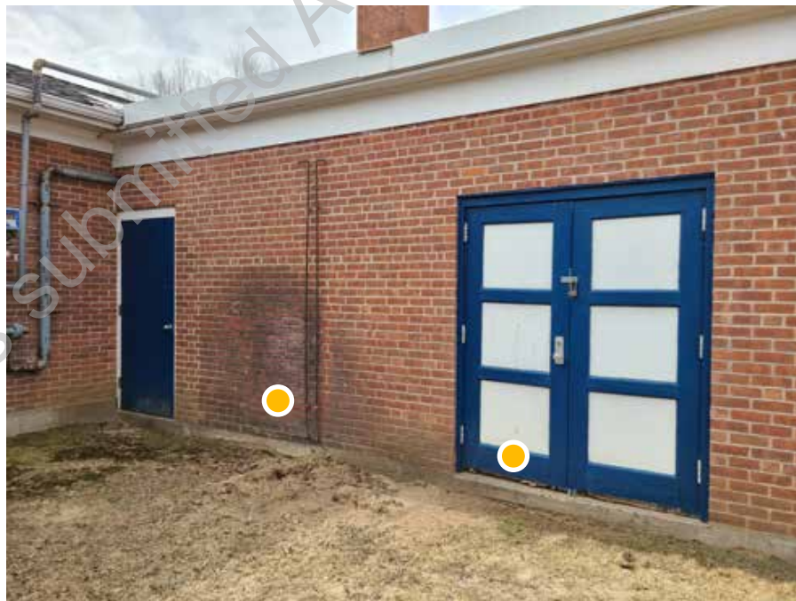
● D1. 8: Detail view of access doors into lower level mechanical room space. Note deterioration at based of wall and doors.
