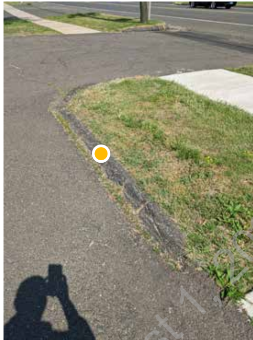
● D3. 7: Damaged bituminous curbs along parking and drive aisles
