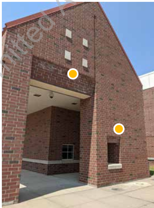
● D1. 22: Signs of efflorescence at entry canopy possible due to moisture infiltration into the masonry cavity.
