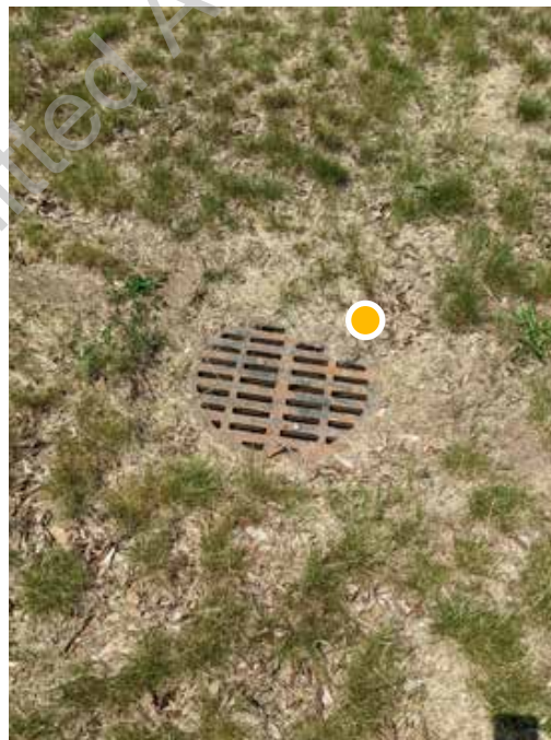
● D3. 18: Detail view of partially obstructed yard drain.
