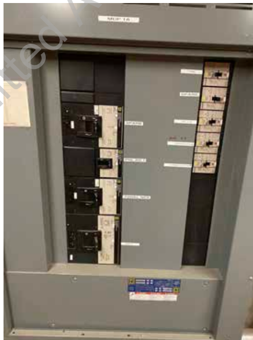
● D2. 6: Electrical Main Distribution Panel #1.
