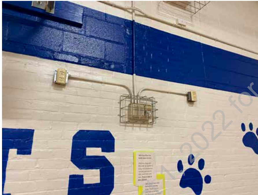
● D2. 13: Fire Alarm Speaker Strobe with RTU Test Switches.
