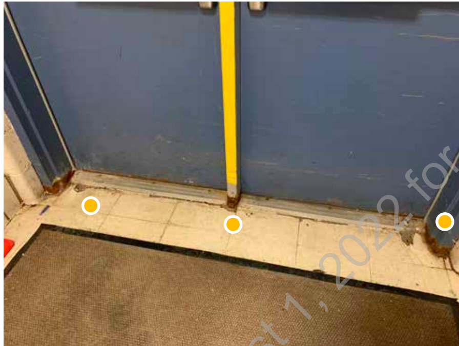
D1. 39: Detail view of exterior door, frame, and sill - all in fairly poor condition overall, signs of deterioration possibly due to moisture
