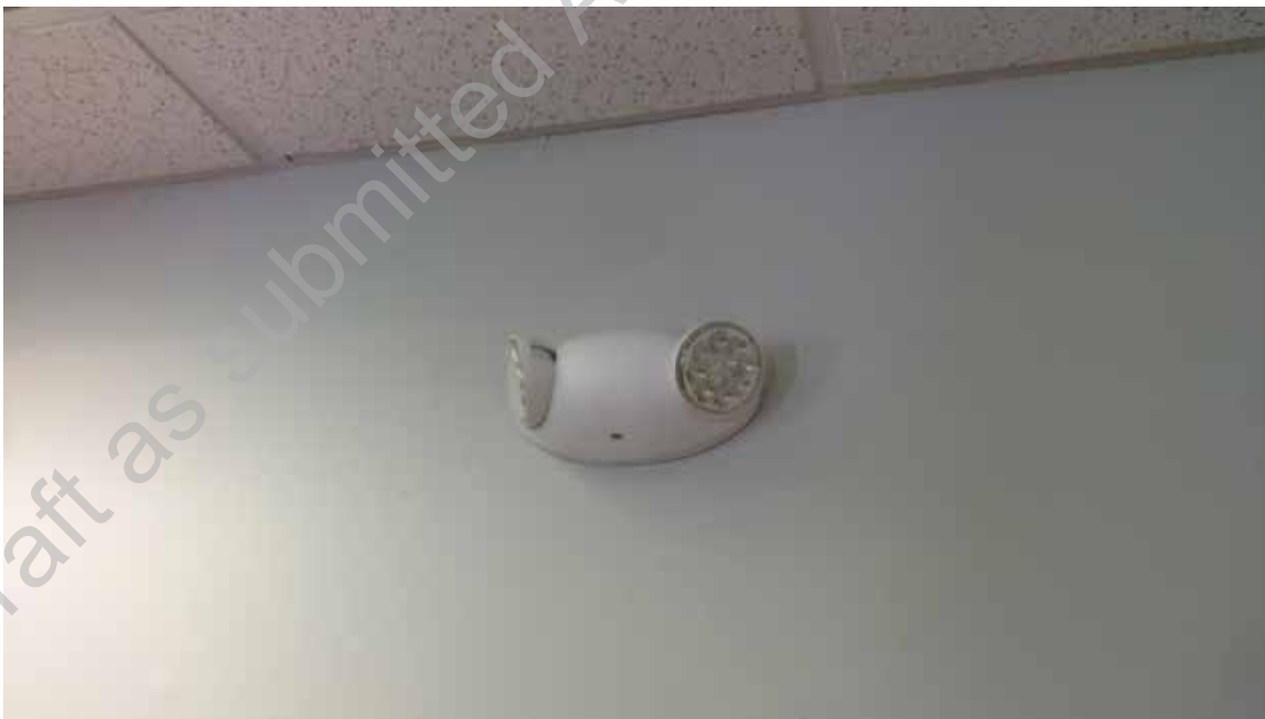
● D2. 22: Interior Egress Lighting Fixture
