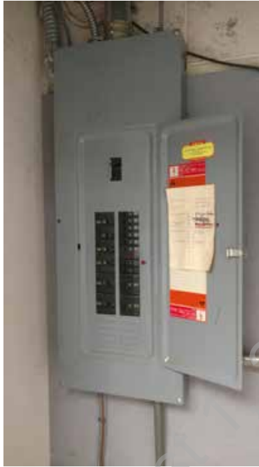
● D2. 11: Electrical Main Service Panel
