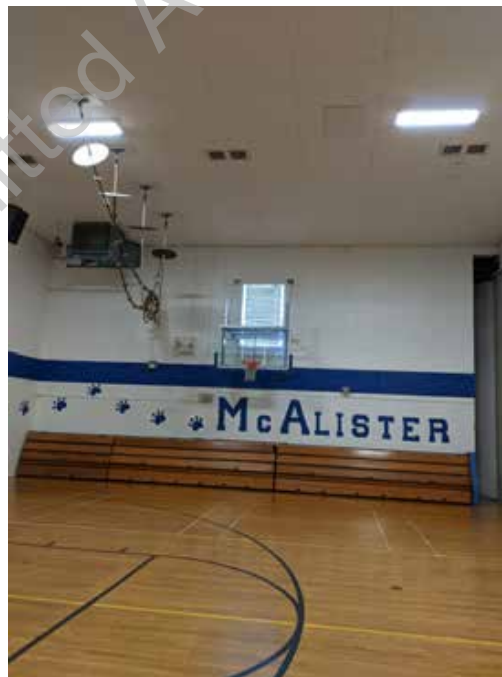
● D1. 28: Overall view of gymnasium in original 1939 building, space has seen limited improvements over the years, note ceiling mounted heating unit and original ACM ceiling tiles.
