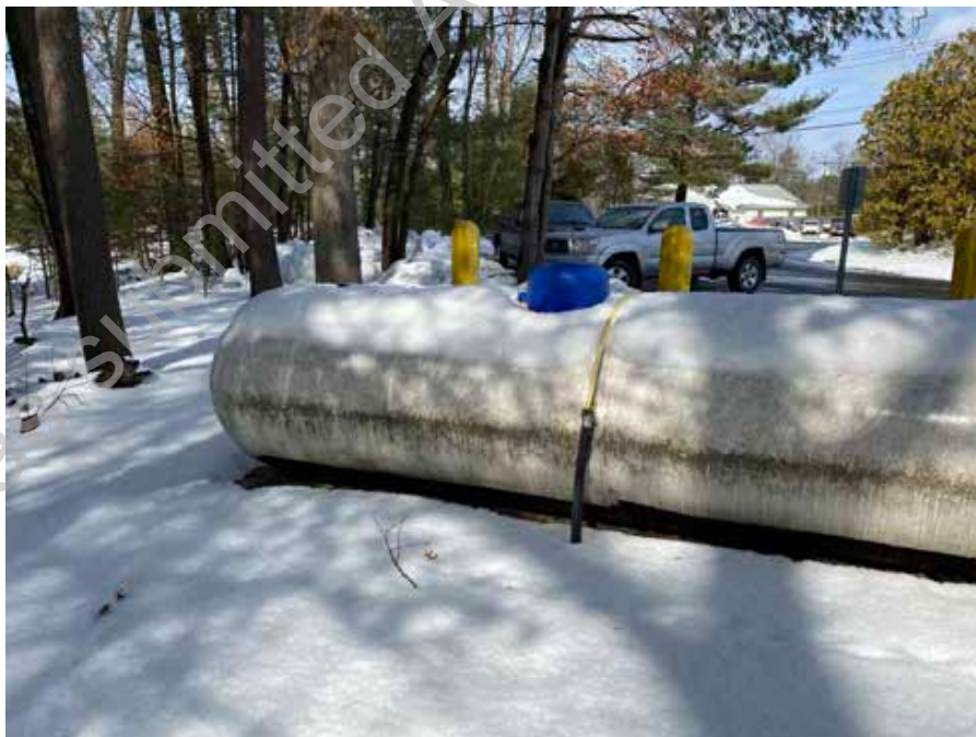
● D2. 24: Propane Tank Located Outside
