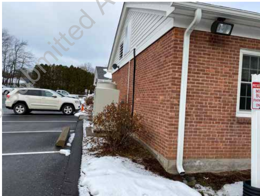
● D2. 26: Gutter Roof Drain System
