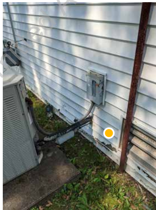
● D1. 22: Vinyl siding damaged at base
