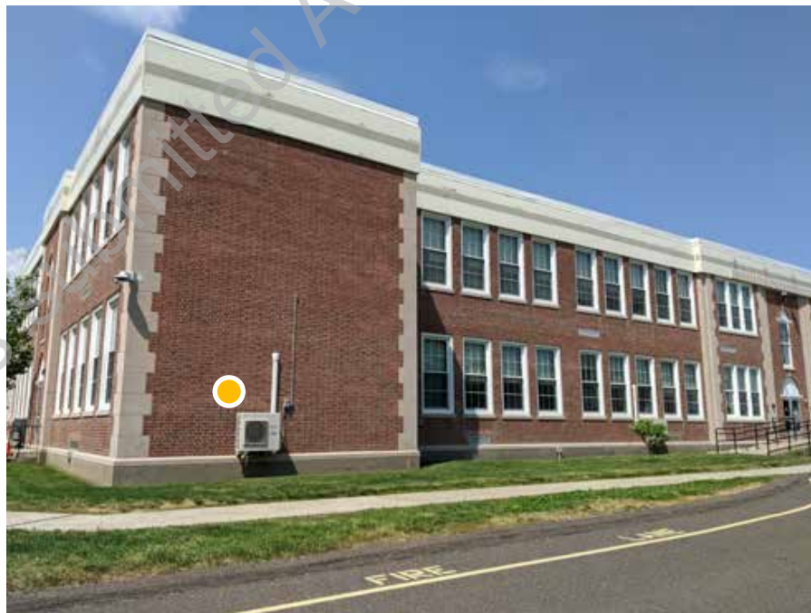
● D1. 4: View of south façade of original 1939 building, note modifications for wall mounted air conditioning unit.
