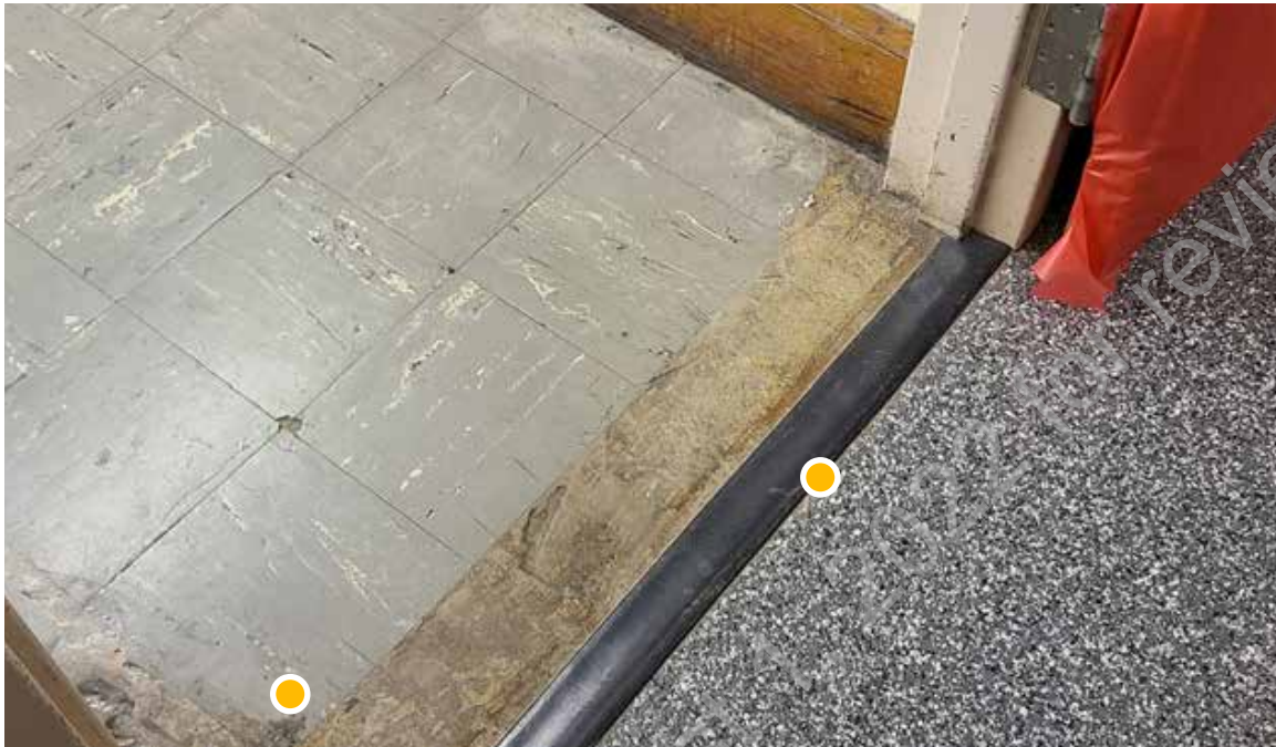
● D1. 35: Typical flooring transition between Kindergarten classrooms and corridor. Note: Possible VAT (vinyl asbestos tile).
