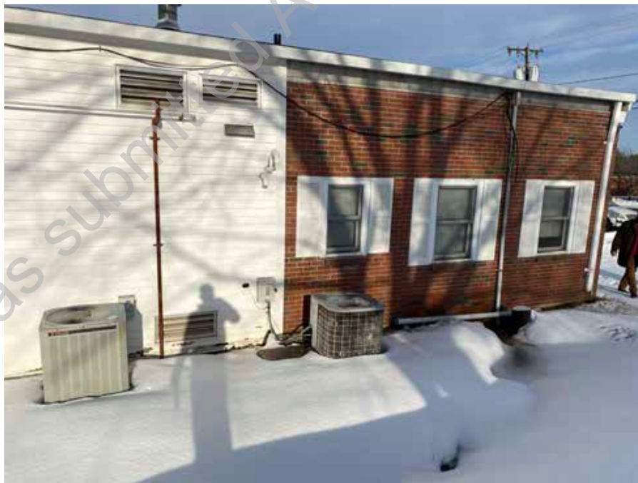
● D2. 34: Trane Condensing Unit Serving the Furnace and Old Abandoned Condensing Unit
