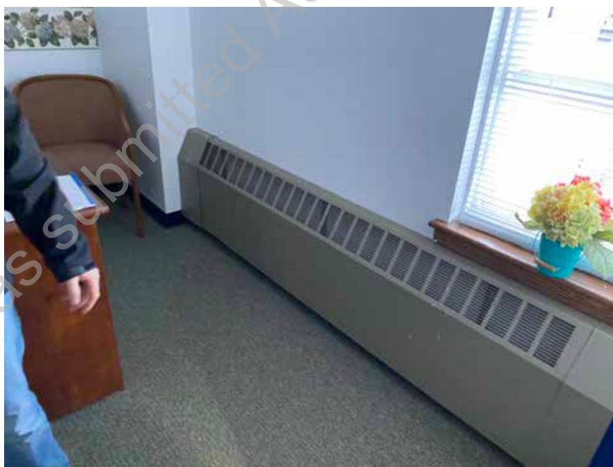
● D2. 36: Old Hot Water Baseboard Radiation
