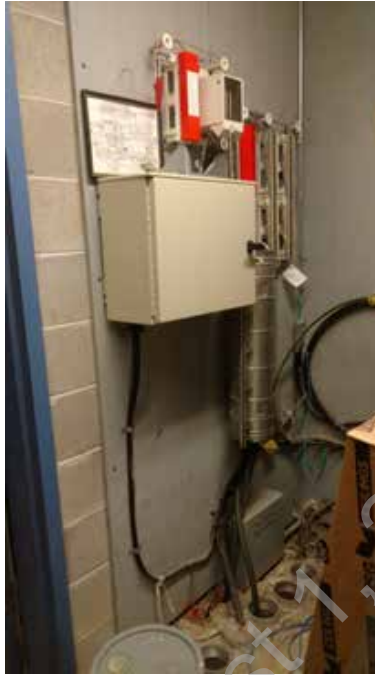
● D2. 3: Communications Service Entrance Backboard
