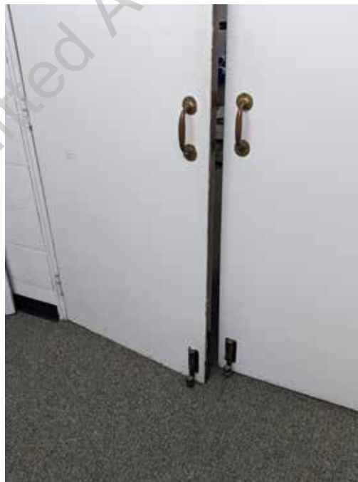
● D1. 40: Door between Lecture Hall and vestibule does not properly seal
