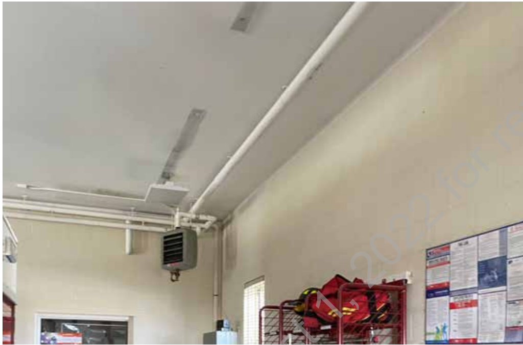
● D2. 17: Hot Water Unit Heater in App Bay
