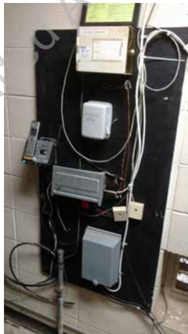
● D2. 22: Telecommunications Service Backboard
