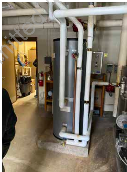
● D2. 12: Indirect Domestic Hot Water Tank and Piping
