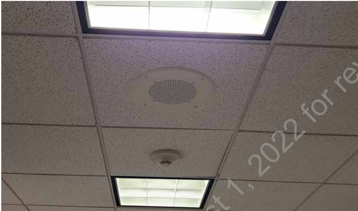
● D1. 29: Fluorescent Light, Smoke Detector and Speaker within Ceiling.
