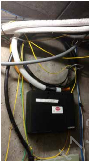
● D2. 15: Fiber Optic Service Equipment
