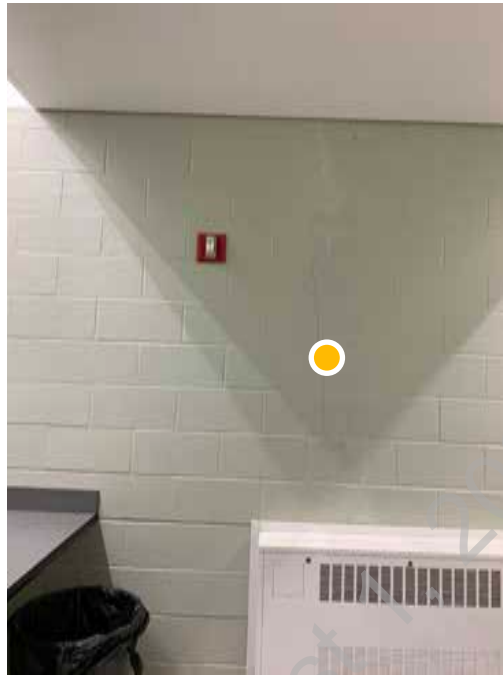
● D1. 43: Detail view of hairline stress fracture in CMU block wall construction, likely due to settlement.
