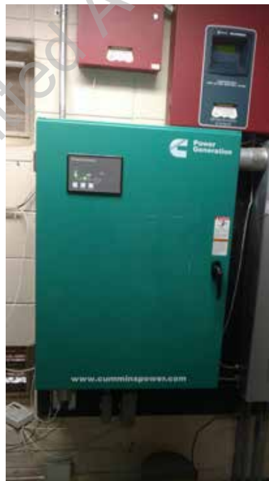
● D2. 2: Automatic Transfer Switch
