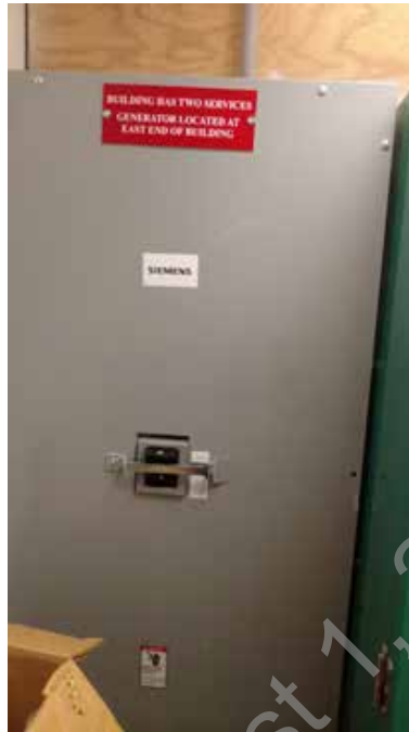
● D2. 9: Electric Service Main Switch
