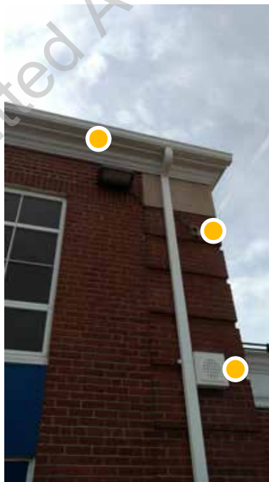
● D2. 14: View at exterior corner of gymnasium depicting roof leader, PA system and security camera retrofits.
