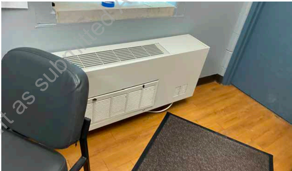
● D2. 22: Newer PTAC Unit in Fair Condition
