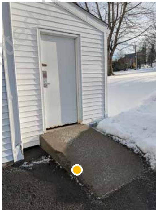
● D1. 8: Spalling concrete at rear storage ramp
