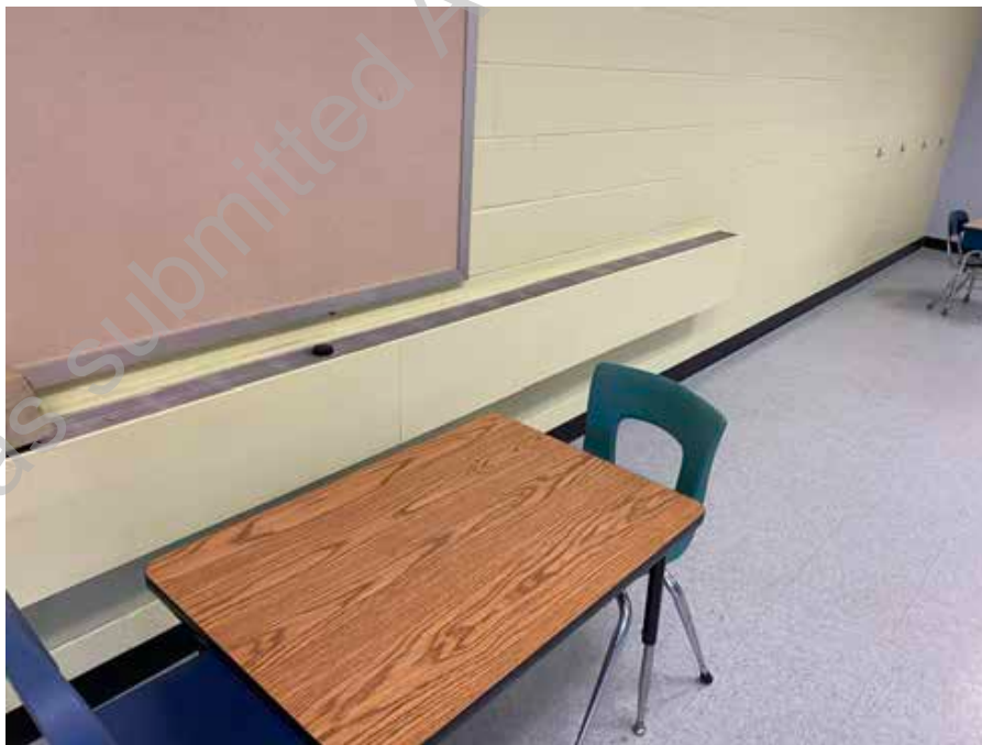
● D2. 26: View of elevated perimeter radiation (heating) in poor condition adjacent to student
