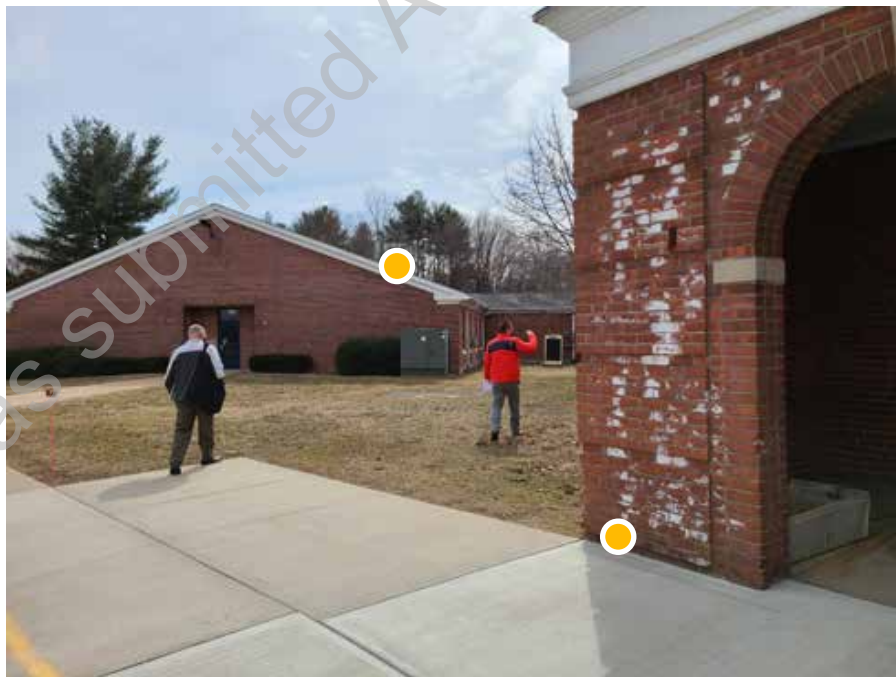
D1. 2: Detail view of the masonry efflorescence (right), view to entry into STEM, art, music, media and specialized education area (left)
