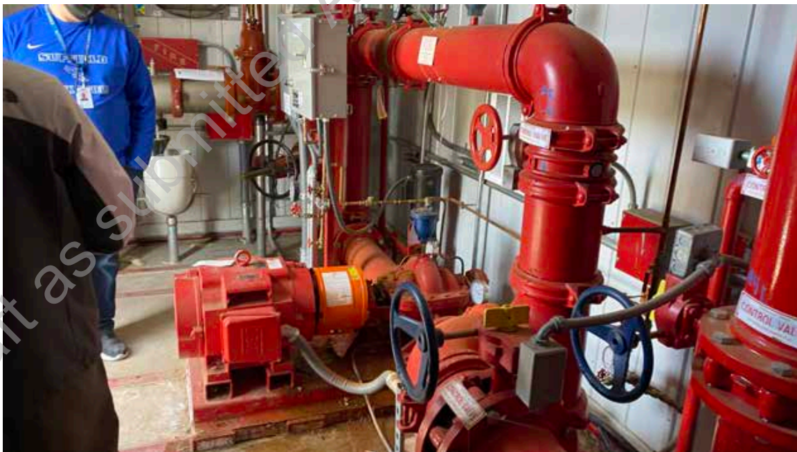
● D2. 20: Fire protection Main and Pump
