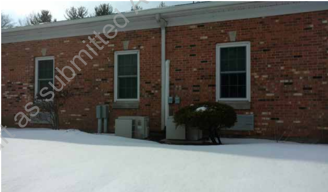
● D2. 18: Mitsubishi Condensing Units Located Outside
