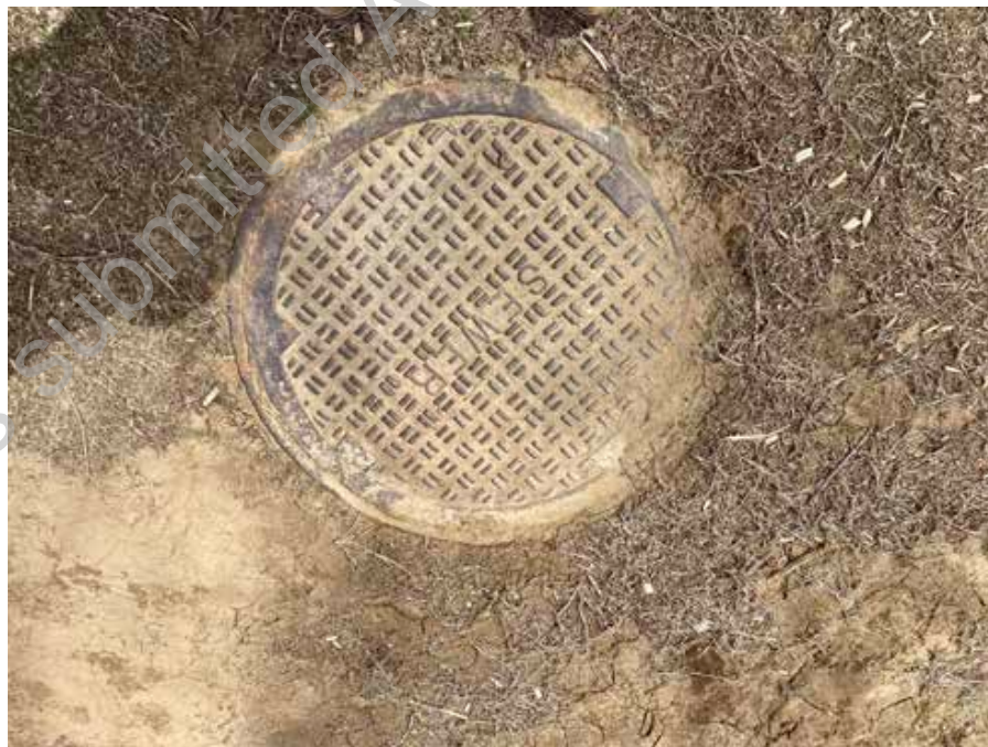
● D2. 24: View of sanitary sewer clean out.
