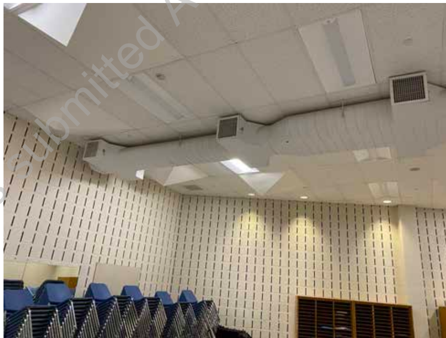
● D2. 12: Exposed Ductwork in Good Condition
