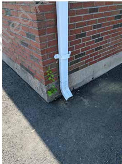
● D1. 16: Downspout dented along pavement
