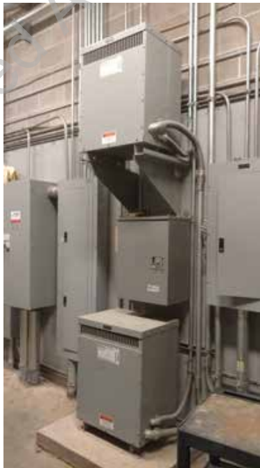
● D2. 4: Electrical Distribution Transformers
