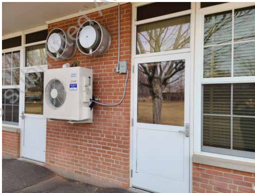
● D1. 16: Sidewall Exhaust Fans and Condensing Unit for Classroom Air Conditioning.
