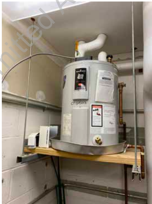
● D2. 8: Electric Domestic Water Heater in Boiler Room
