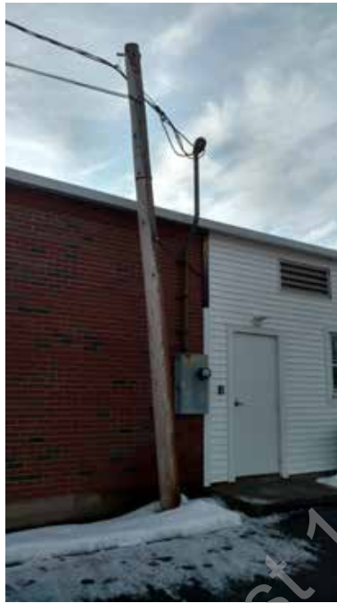
● D2. 13: Electrical Service Drop at Meter
