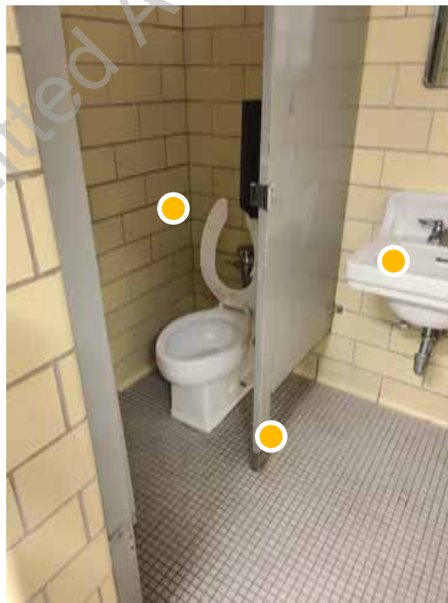
● D1. 36: Detail view of toilet configuration adjacent to girls locker room, does not meet current accessibility codes.
