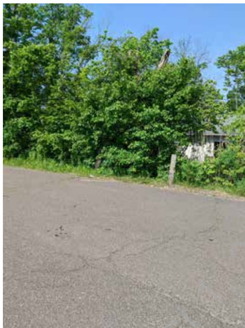
● D3. 9: Cracking pavement throughout parking areas and drive aisles
