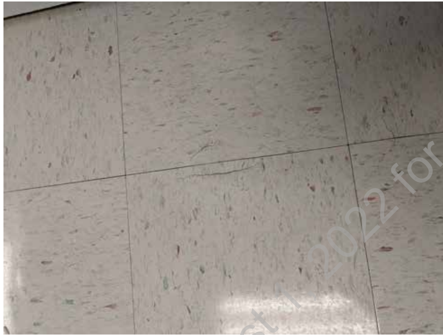
● D1. 43: Damaged vinyl tile flooring at break area
