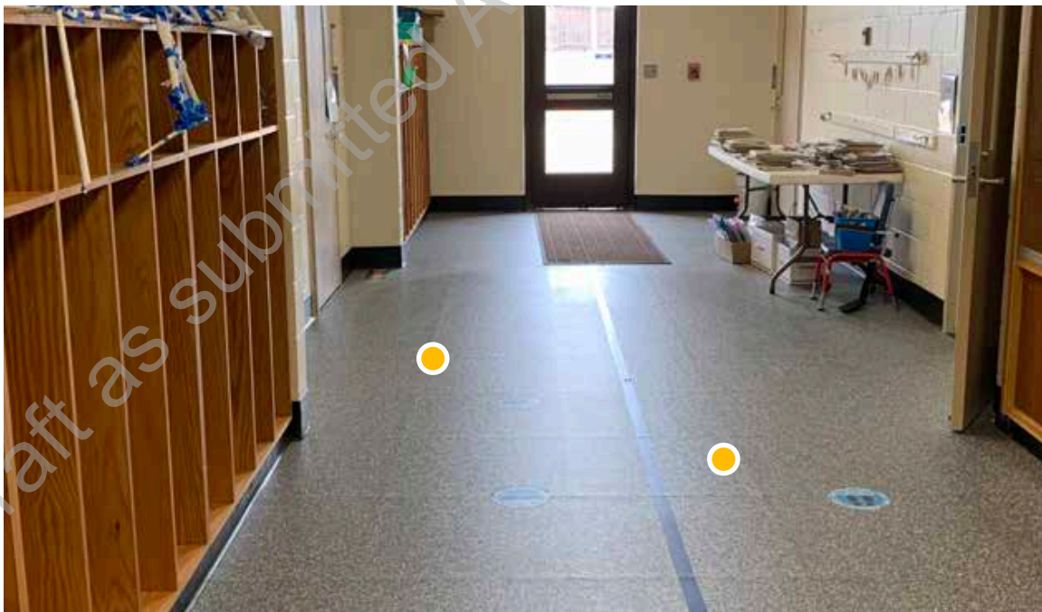
● D1. 62: View of flooring retrofit over existing possible VAT (vinyl asbestos tile). Note seaming telegraphing through surface.
