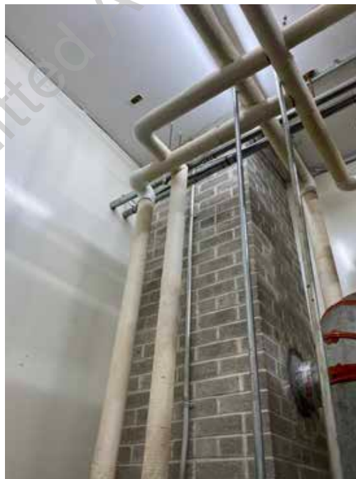
● D2. 6: Domestic Water Piping in Poor Condition
