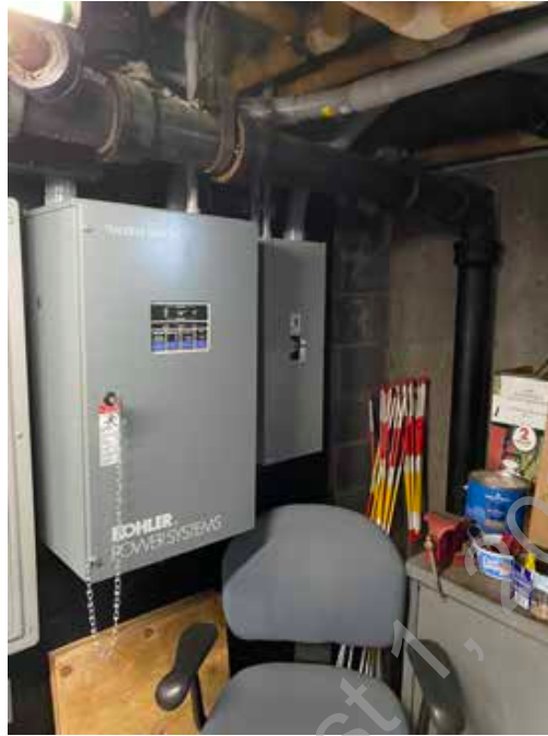
● D2. 3: Automatic Transfer Switch
