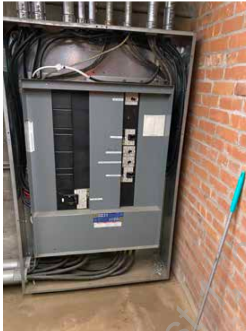
● D2. 7: Electrical Main Distribution Panel #2.
