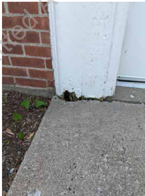
● D1. 20: Damaged wood trim at entry door
