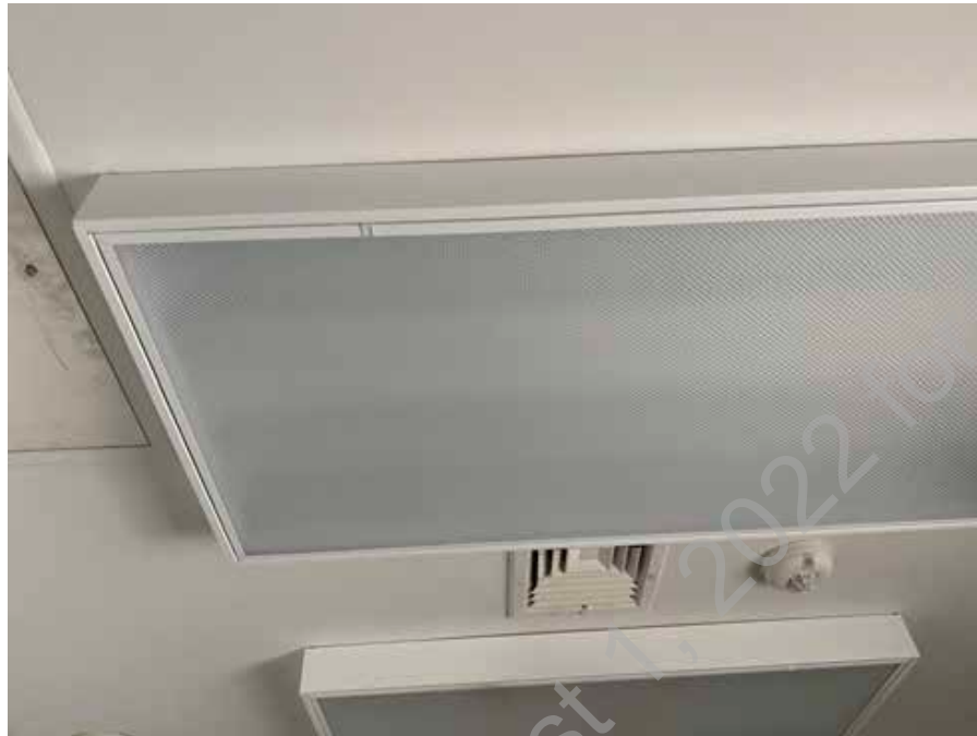
● D2. 21: Fluorescent Lighting with Occupancy Sensor Control
