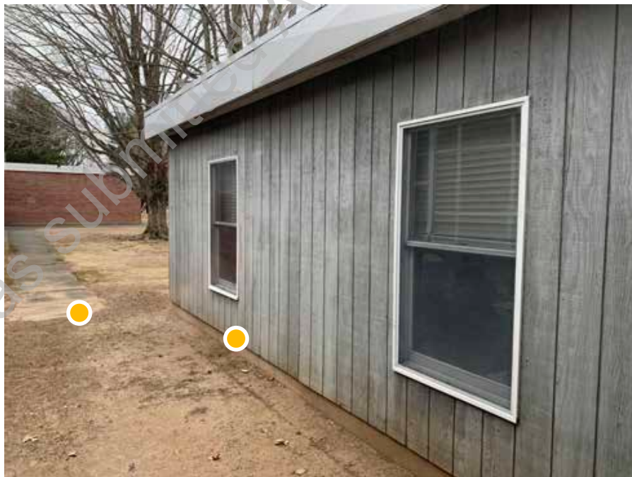
D1. 18: Detail view of the modular classroom building, note deterioration of siding and asphalt sidewalk in poor condition.
