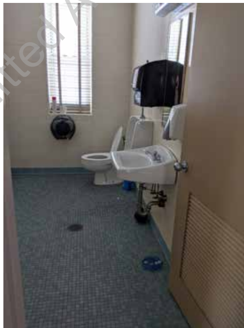
● D1. 16: Grab bars at toilet room do not meet ADA requirements to be considered compliant; pipe insulation is missing below lavatory
