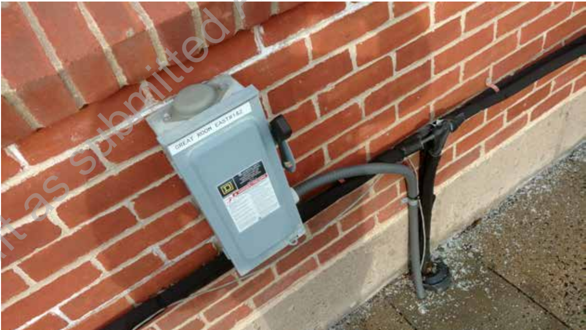
● D2. 18: Exterior Condenser Power Feed
