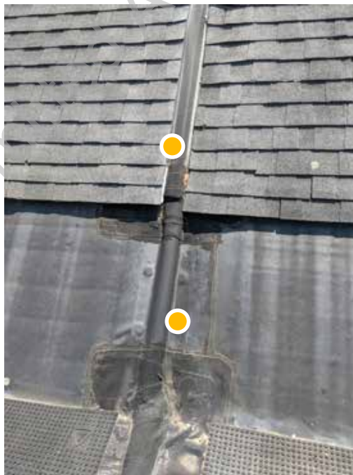
● D1. 6: Typical roof expansion joint at membrane roofing and asphalt shed roof
