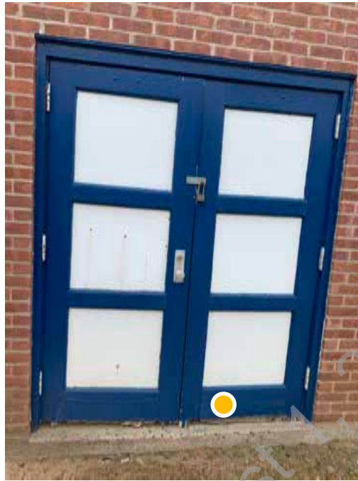
● D1. 21: View of exterior doors to mechanical space, note the poor condition at base.
