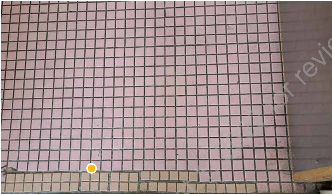
● D1. 55: Typical original bathroom floor tile with patched area.
