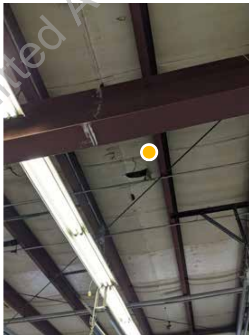
● D1. 36: Damaged roof insulation throughout storage garage
