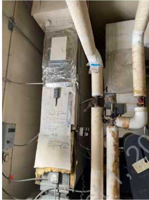
● D2. 5: Ductwork and Hot Water Piping in Poor Condition
