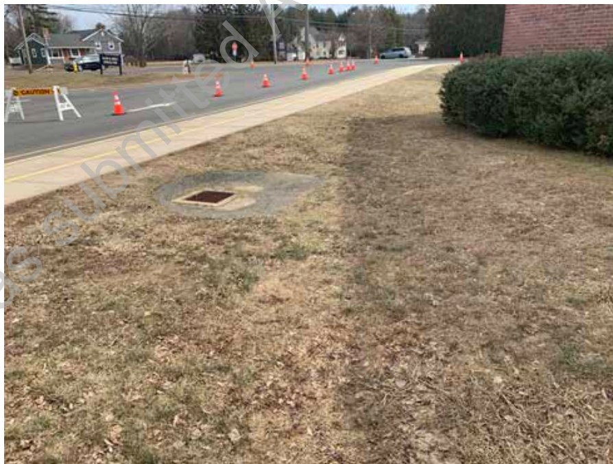
● D3. 8: Typical condition of grass areas throughout site. Unconventional location and construction of yard drain.
