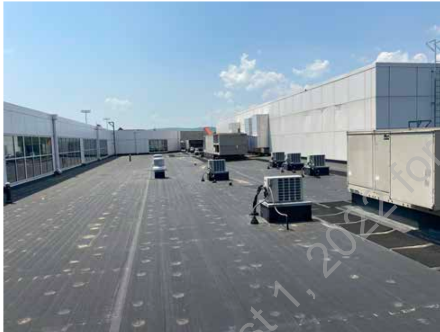
● D2. 11: Exhaust Fans, Rooftop Units, and Condensing Units on Roof
