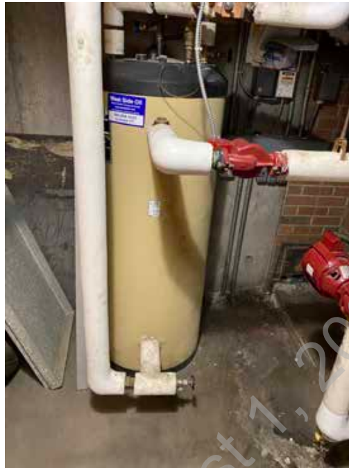
● D2. 23: Indirect Domestic Hot Water Heater
