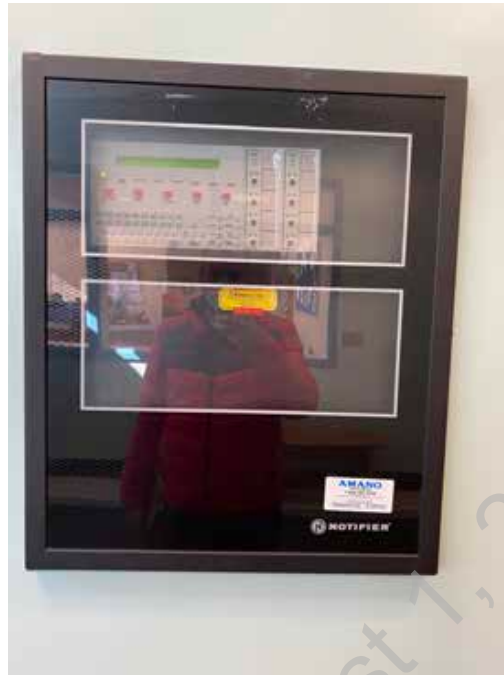
● D2. 11: Fire Alarm Control Panel.
