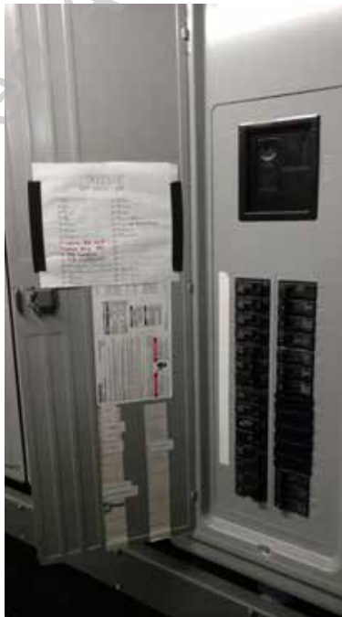
● D2. 4: Branch Circuit Panelboard
