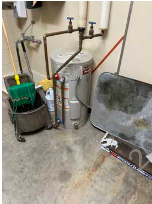
● D2. 3: Electric Domestic Water Heater
