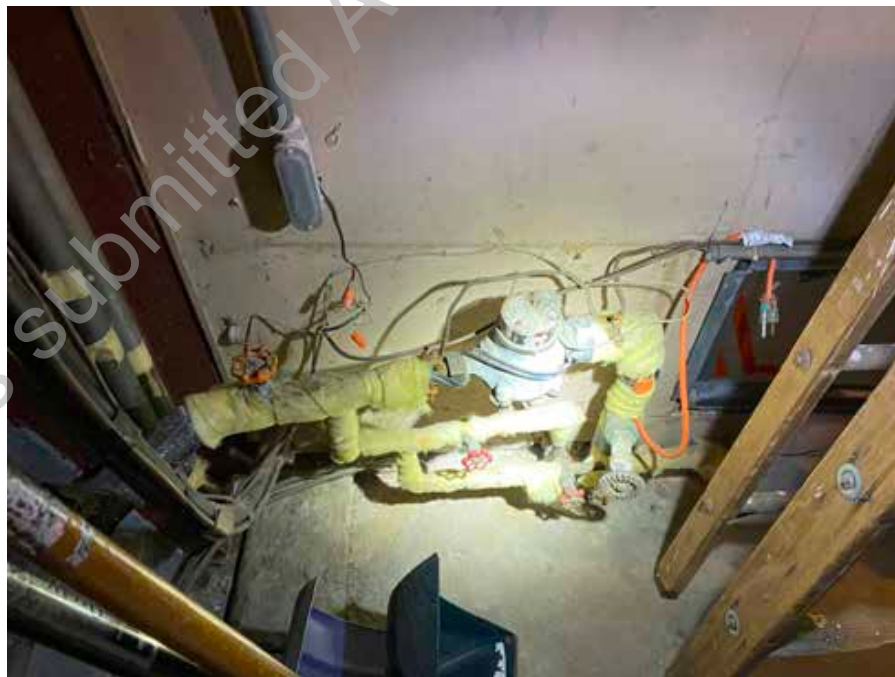
● D2. 4: Domestic Water Service in Poor Condition
