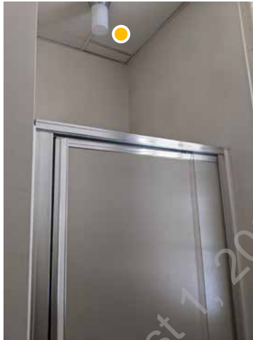
● D1. 15: Acoustic ceiling tile track showing signs of rust above shower stalls
