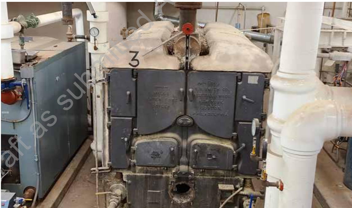
D1. 46: Abandoned Old Cast Iron Boiler in Mechanical Room.
