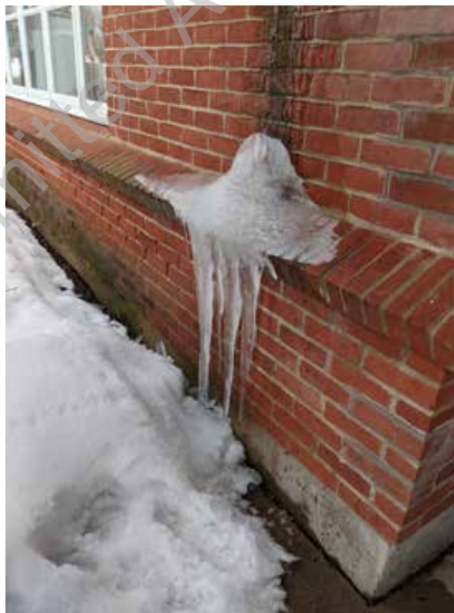
● D1. 14: Lack of proper gutter flashing above is causing ice build up and staining on brick shelf below
