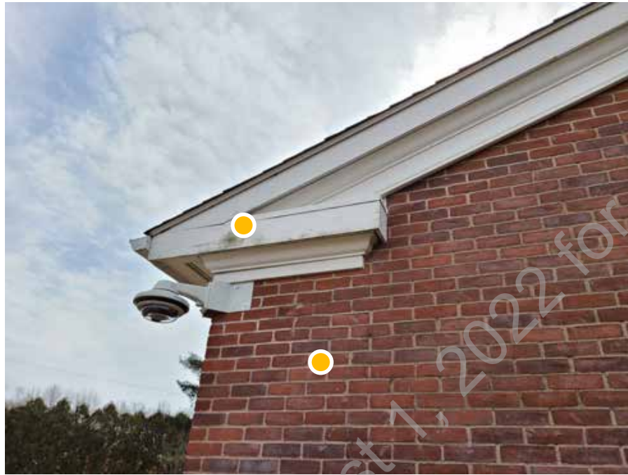
● D1. 11: Detail view of wood fascia trim at 1988 addition.
