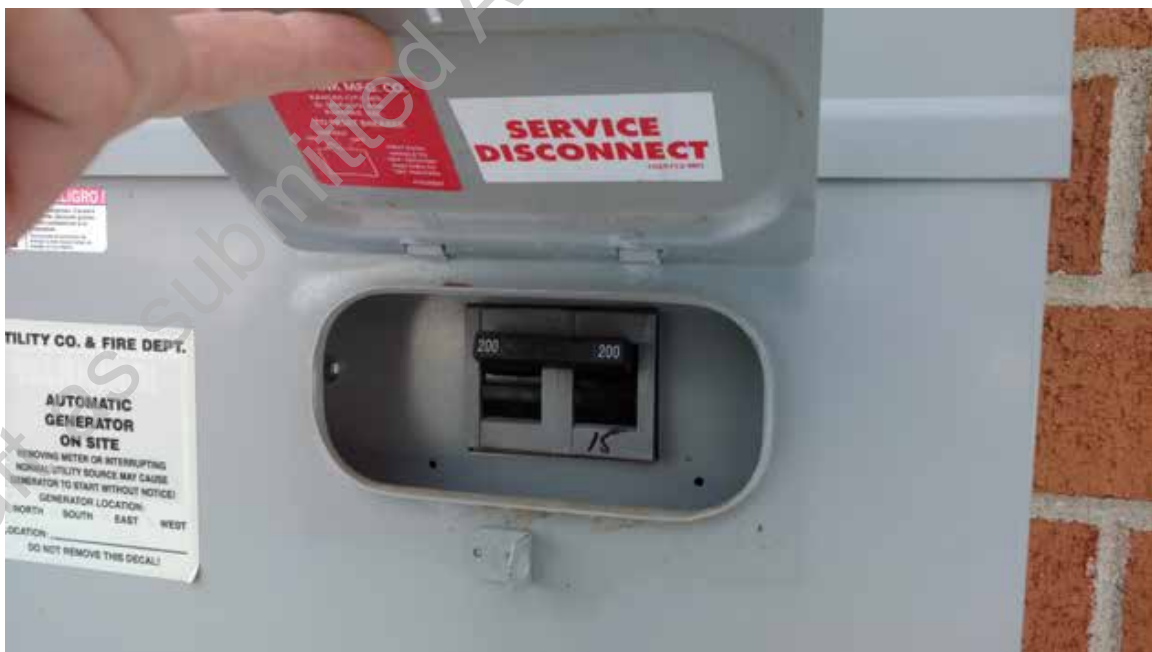
● D2. 18: Main Service Disconnect Switch
