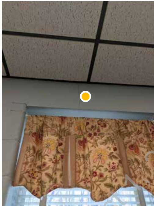
● D1. 13: Gypsum board cracking above windows throughout
