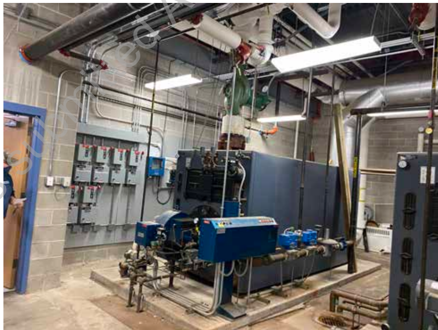
● D2. 40: Oil Fueled Cast Iron Boiler in Mechanical Room in Fair Condition
