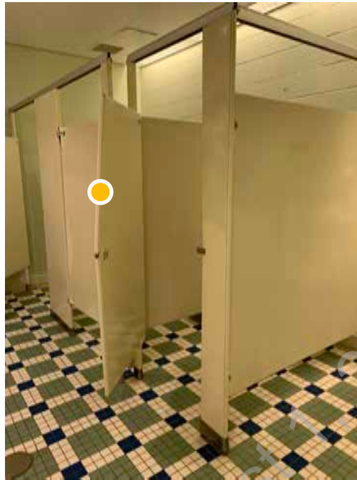
● D1. 49: Detail view of typical toilet room, note damaged metal toilet partition.
