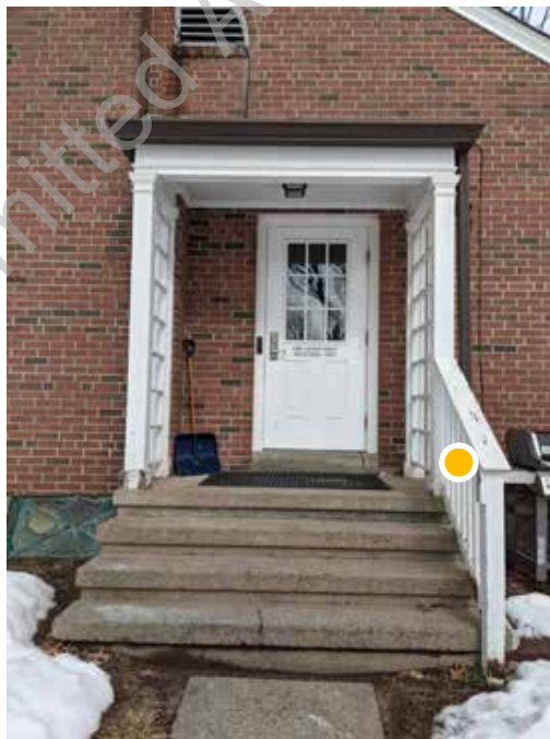
● D1. 6: Rear Staff entry is not wheel chair accessible; wood trim and railing is decaying
