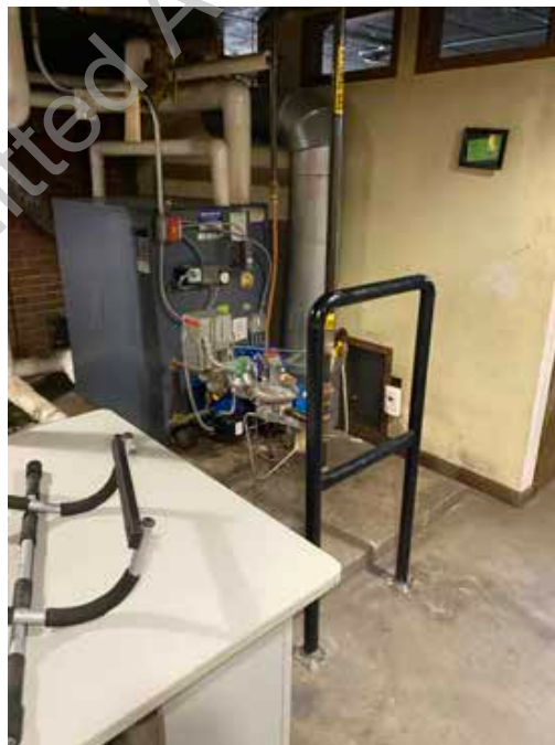
● D2. 28: Natural Gas Hot Water Boiler
