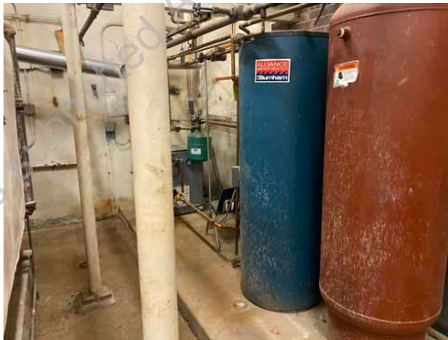
● D2. 4: Burnham Indirect Domestic Hot Water Storage Tank.
