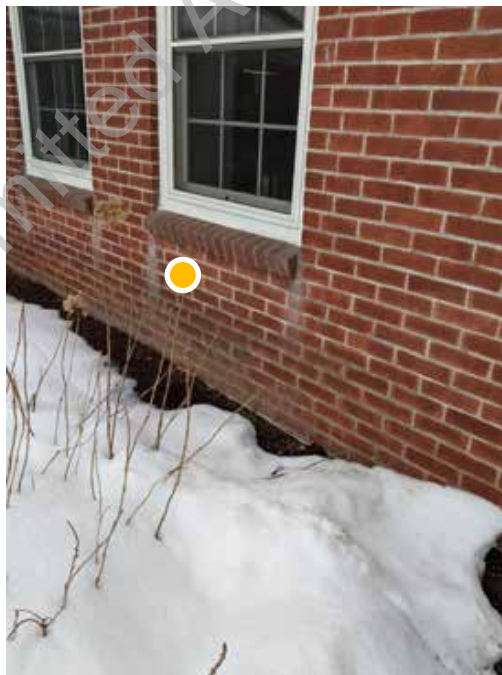
● D1. 10: Staining at brick below windows
