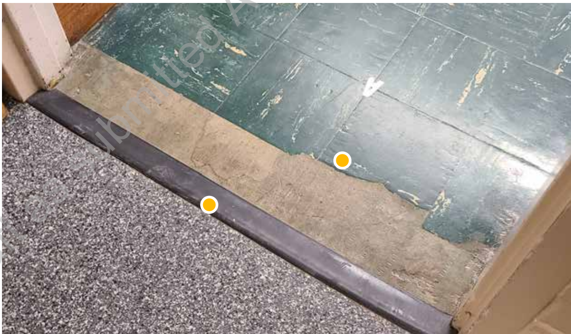
● D1. 36: Typical flooring transition between Kindergarten classrooms and corridor. Note: Possible VAT (vinyl asbestos tile).
