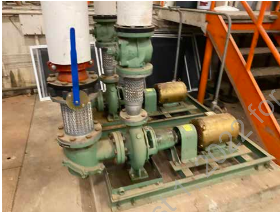
● D2. 19: Hot Water Pumps in poor condition.
