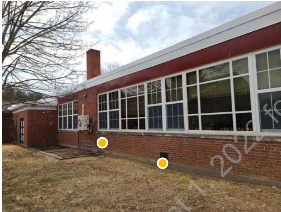
● D1. 5: View of original classroom wing (1954). Note deterioration of masonry joints and foundation wall at grade.
