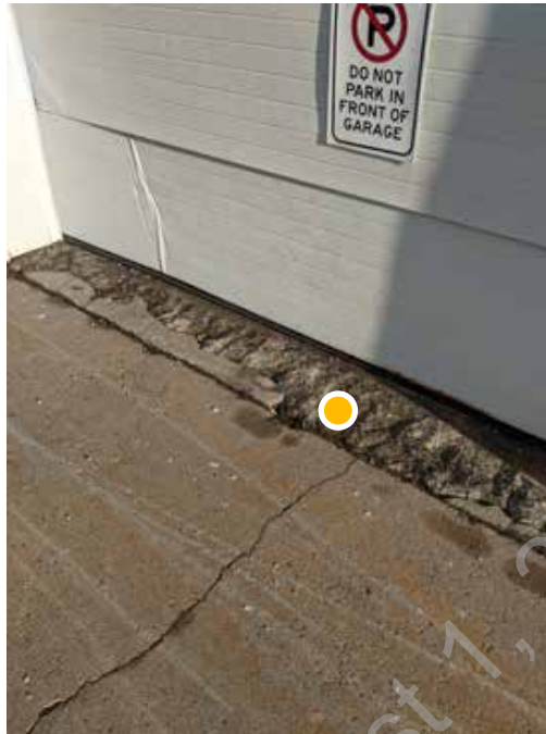
● D1. 9: Concrete spalling at garage door thresholds
