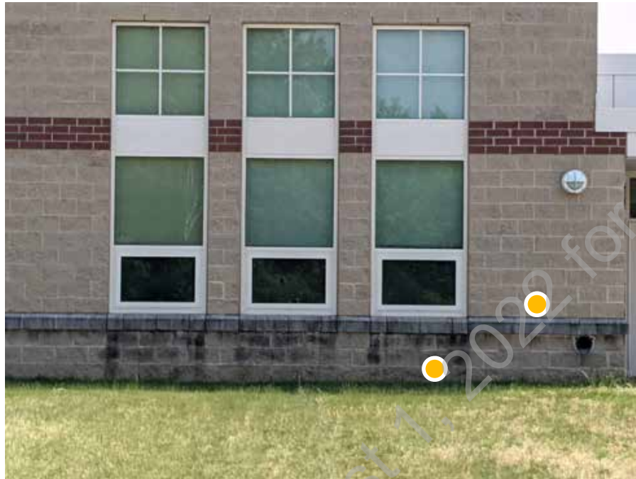
● D1. 15: North façade of existing school depicting signs of moisture infiltration and concrete block deterioration
