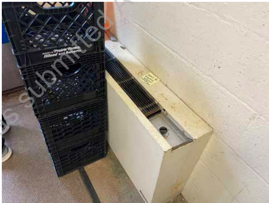
● D2. 32: Old Hot Water Convactor needs replacement.
