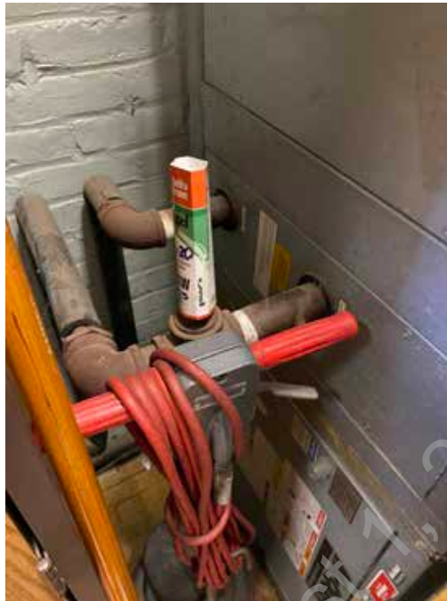
● D2. 27: McQuay Heating and Ventilating Unit.
