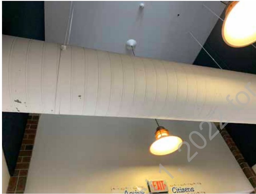
● D1. 47: Detail view of exposed spiral ductwork, note deterioration of paint finish
