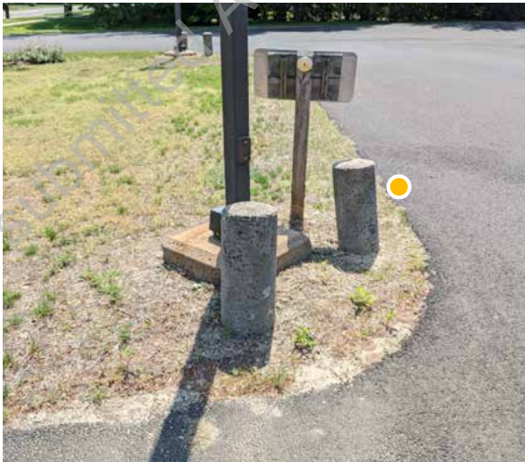
● D3. 6: Concrete bollards require reseating
