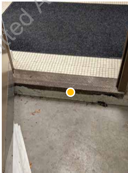
● D1. 28: Step-down into Maintenance Garage and Sally Port creates a non-accessible condition
