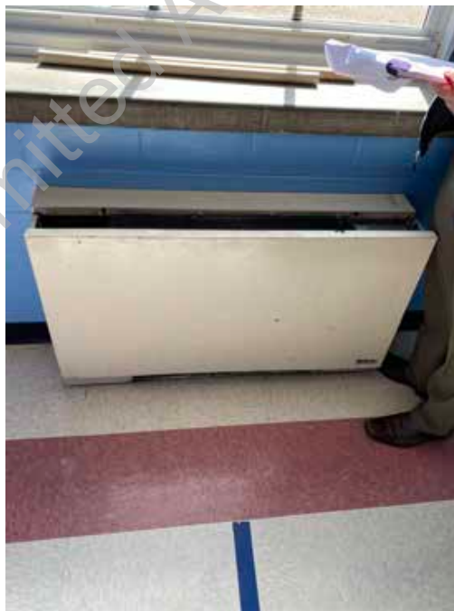
● D2. 28: Detail view of poor condition of typical cabinet heaters throughout the building. McQuay Hot Water Convectors Needs Replacement.
