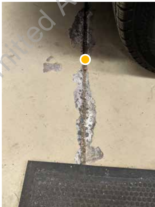
● D1. 42: Spalling concrete control joints in storage area
