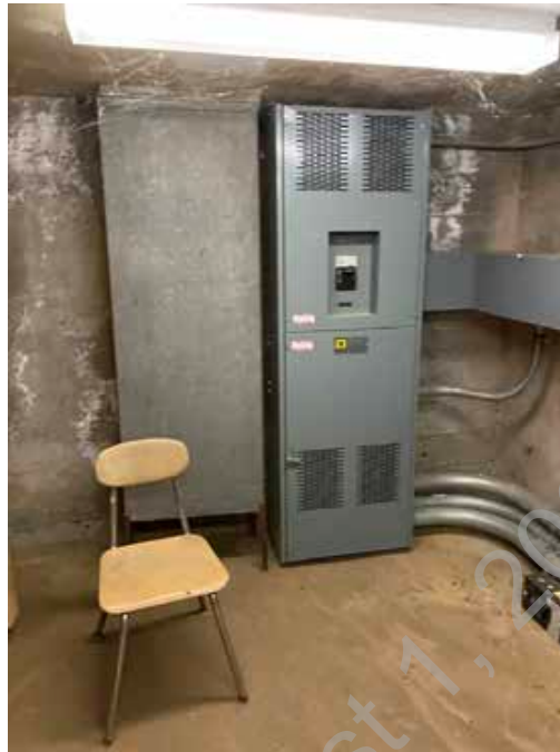
● D2. 9: Electrical Main Service Switch.
