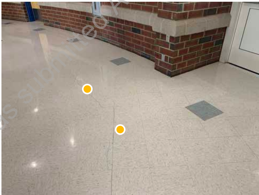
D1. 26: View of VCT flooring at main entry/cafeateria, note the stress cracks along the walkway
