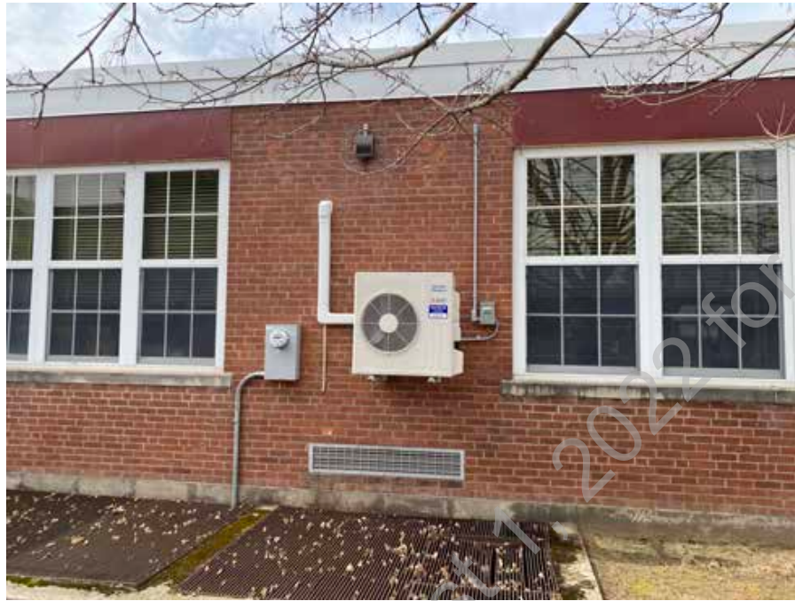
● D2. 23: Mitsubishi Condensing Unit Serving Classroom Split Units.
