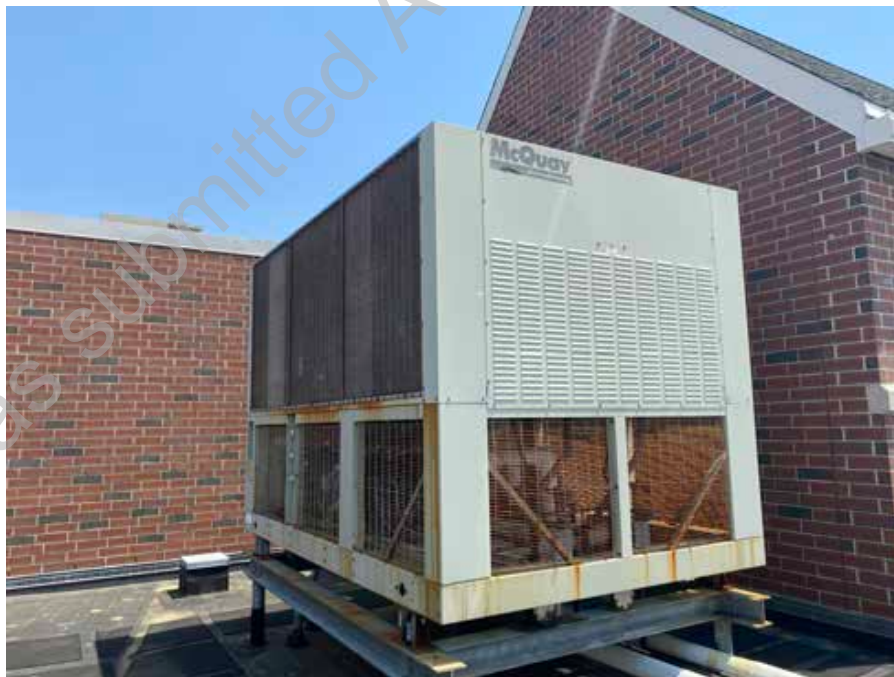
D2. 38: McQuay Air Cooled Condensing Unit on Roof
