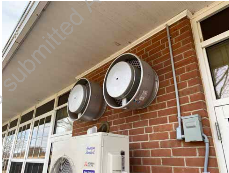
● D2. 12: Exhaust Fans Serving Labs.
