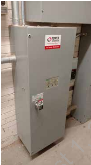
● D2. 3: Automatic Transfer Switch.
