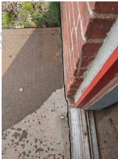
● D1. 16: Cracking at rear mechanical room sidewalk
