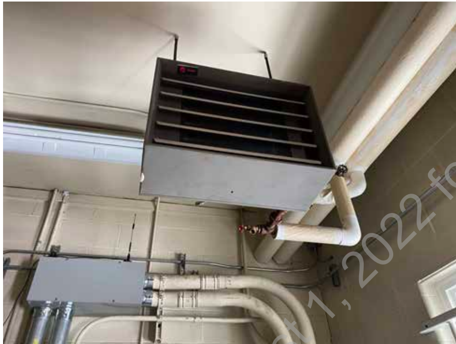
● D2. 11: Hot Water Unit Heater
