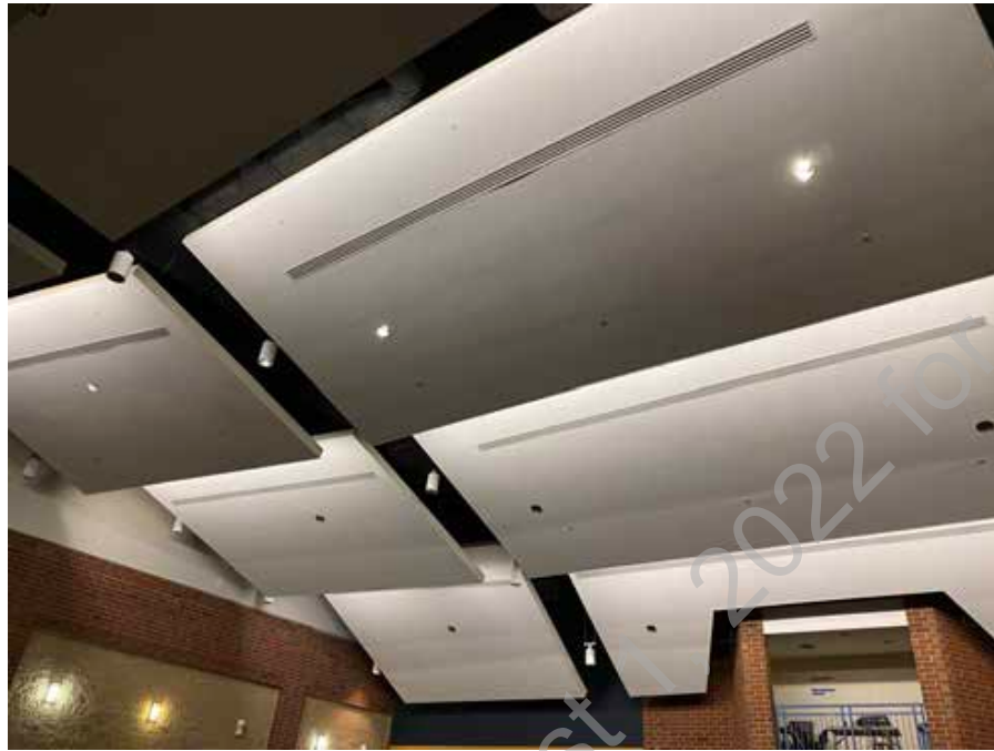
● D2. 35: Linear Slot Diffusers in Auditorium
