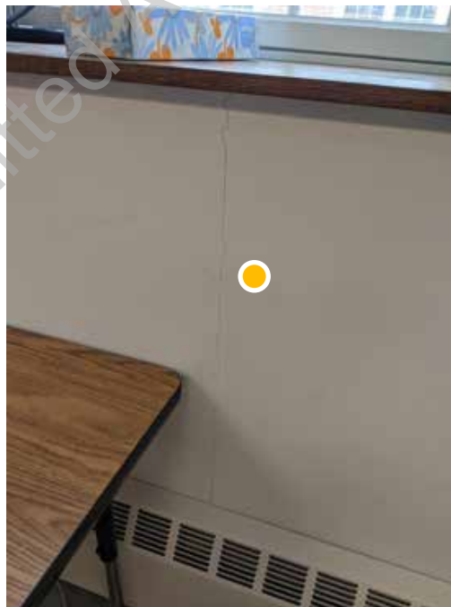
● D1. 44: Gypsum board cracking below windows
