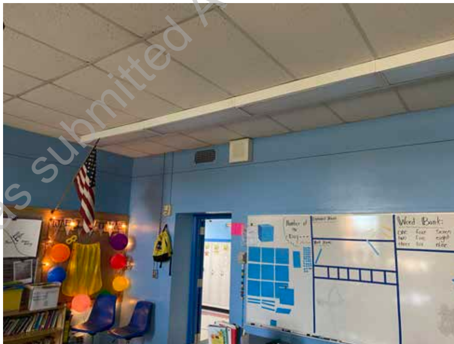
● D2. 4: View of typical classroom with antiquated and inefficient fluorescent lighting surface mounted to ceiling.
