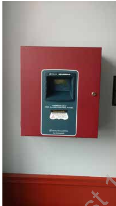
● D2. 13: Fire Alarm Control Panel
