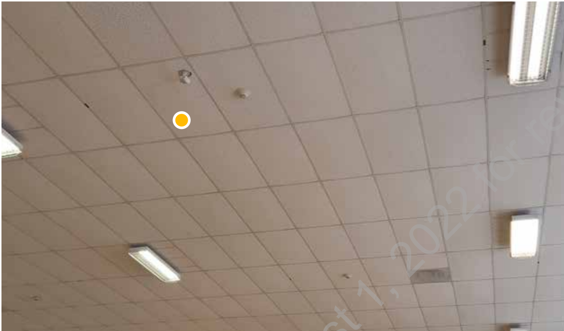
● D1. 49: View of lay in tile ceiling in the gymnasium. Several missing or damaged tile, note the cupping of the tile edges due to possible humidity control.
