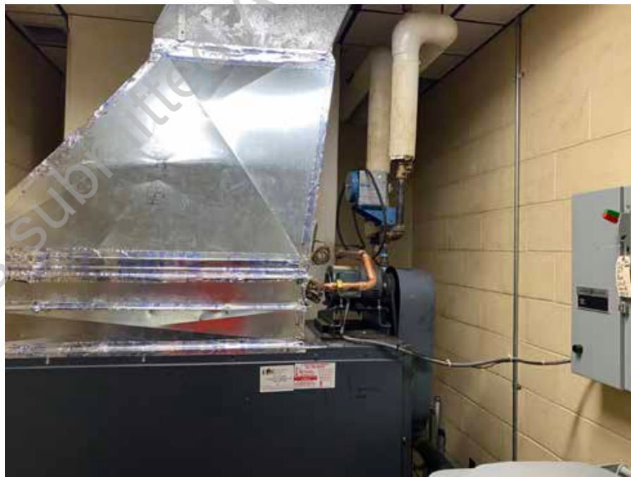
● D2. 10: Hot Water Piping and Dcutwork from HAC 2 in Poor Condition
