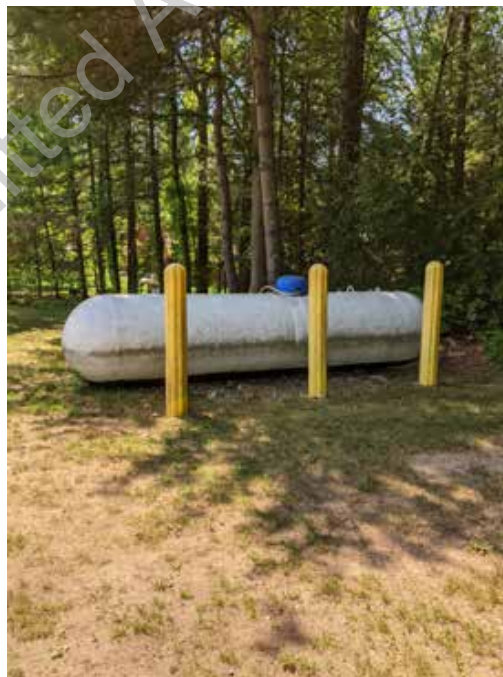
● D3. 8: Existing above-ground propane tank with bollards
