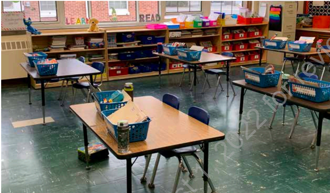
● D1. 59: View of typical classroom with linear shelving in front of perimeter radiation along exterior wall. Note patched VAT (Vinyl asbestos tile) flooring.
