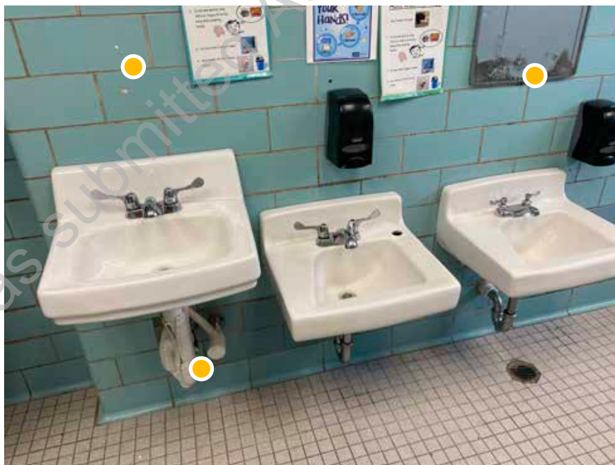
● D2. 30: View of typical toilet room with original wall and floor tile. ADA adjustments made to one site for floor clearance. Wrap protection in poor condition. No accessible mirror or soap dispenser.
