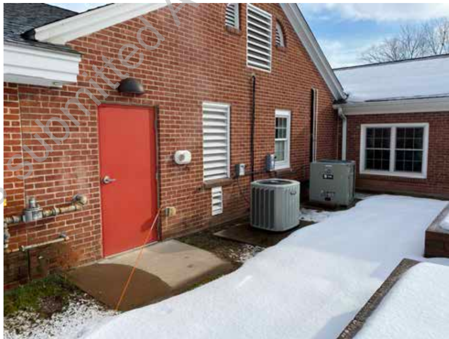
● D2. 38: Outdoor Condensing Units Serving Terminal units Indoors
