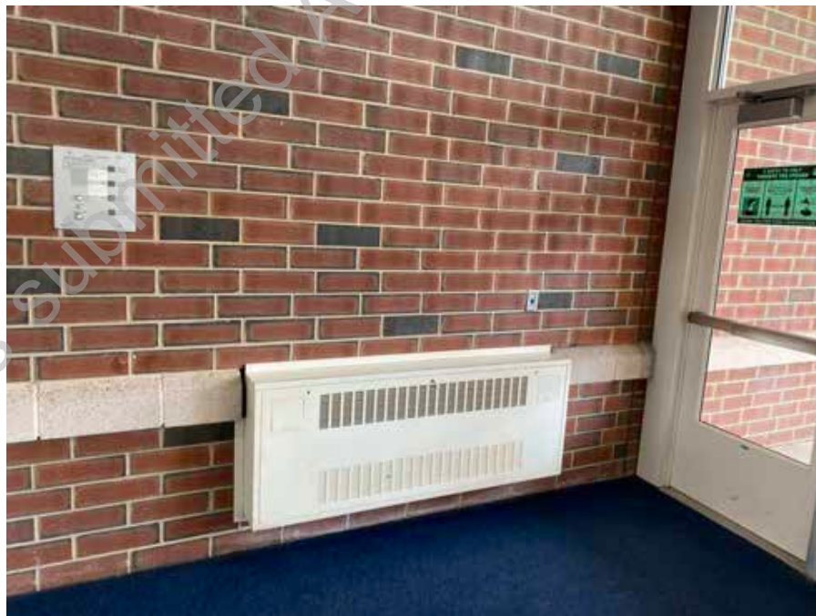
● D2. 56: Vestibule Hot Water Cabinet Unit Heater in Fair Condition
