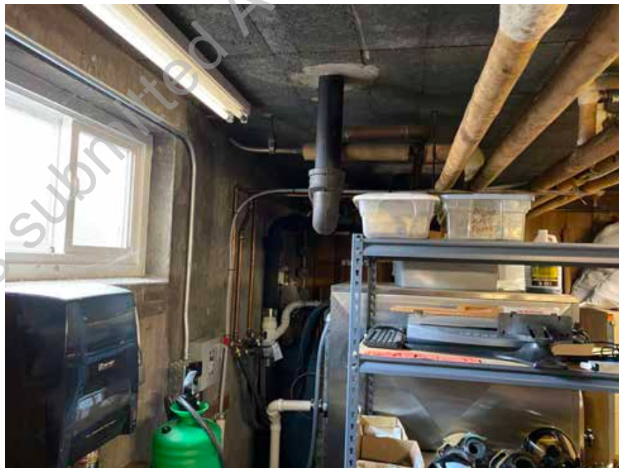
● D2. 20: Hydronic and Domestic Water Piping Needs to be Replaced
