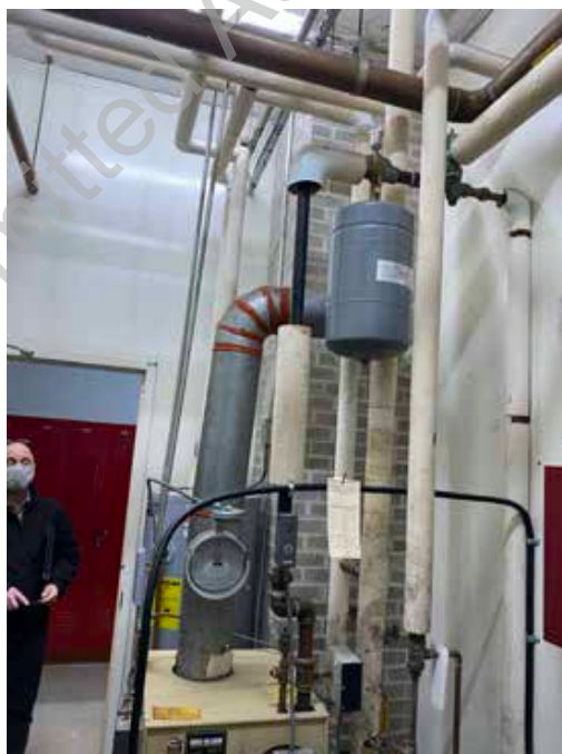
● D2. 16: Hot Water Piping in Poor Condition
