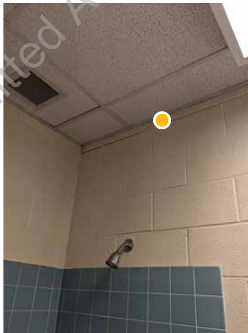
● D1. 24: Cracking of concrete masonry unit walls observed throughout
