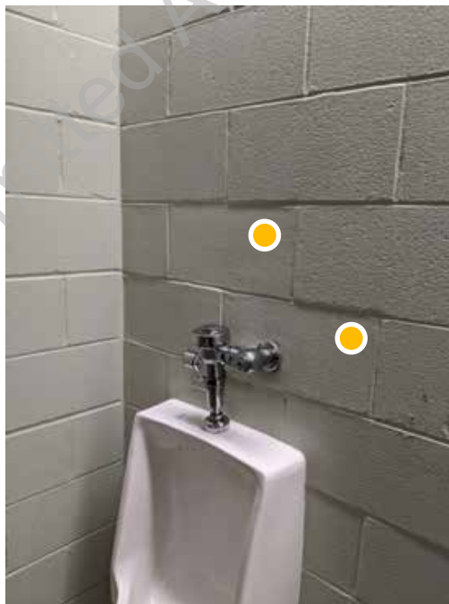
● D1. 74: Detail view of poorly constructed CMU wall, part of original construction.
