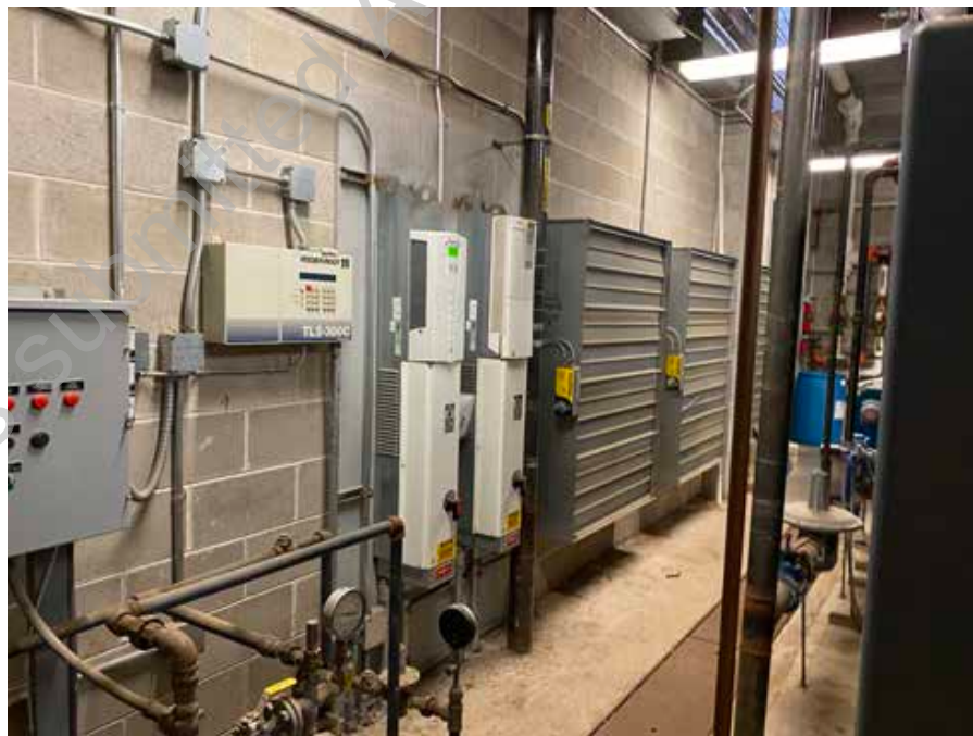
● D2. 52: VFDs Located in Mechanical Room
