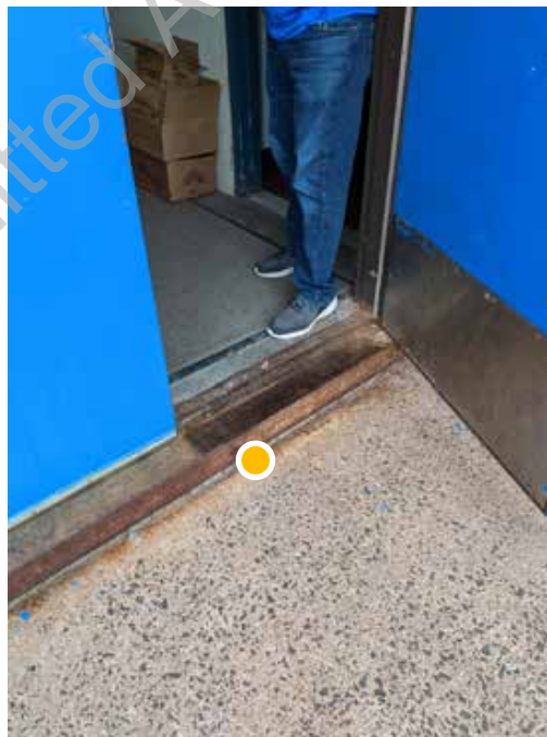
● D1. 44: Loading/receiving door access, note step up into building making delivery and access difficult.
