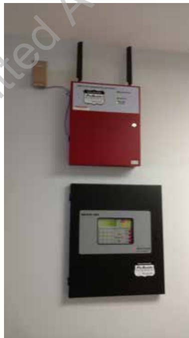
● D2. 20: Fire Alarm Control Panel
