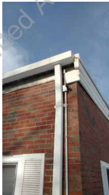
● D2. 30: Rood Drain Gutter System
