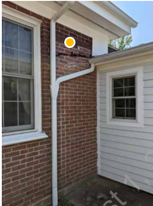
● D1. 21: Adhesive left from former roof to wall flashing location
