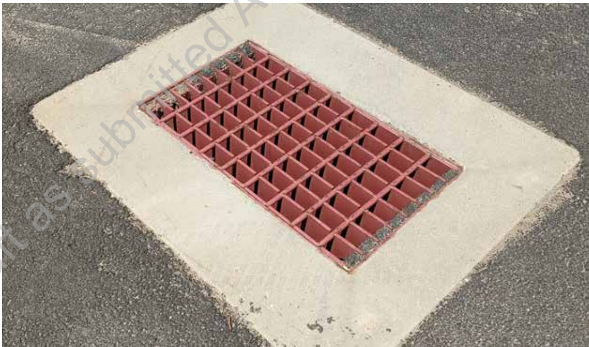
● D3. 16: Concrete basin tops are in good condition and appear to have been replaced along with recent parking lot work
