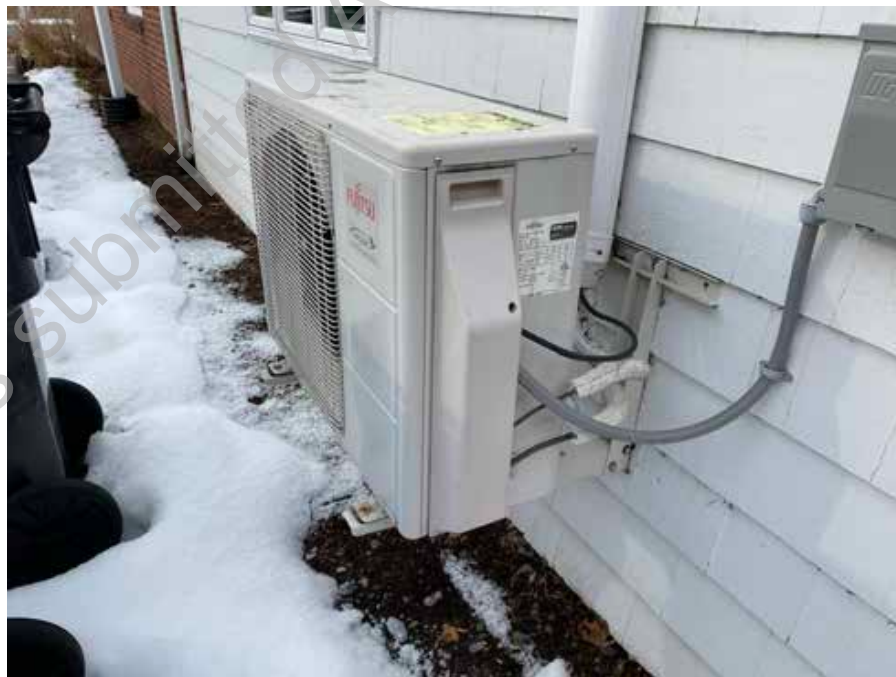
● D2. 22: Fujitsu Condensing Unit Serving Split Unit
