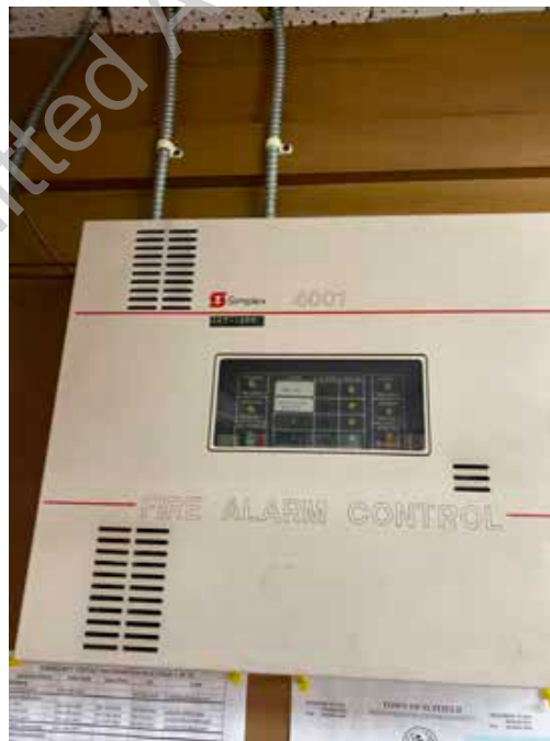
● D2. 16: Fire Alarm Control Panel
