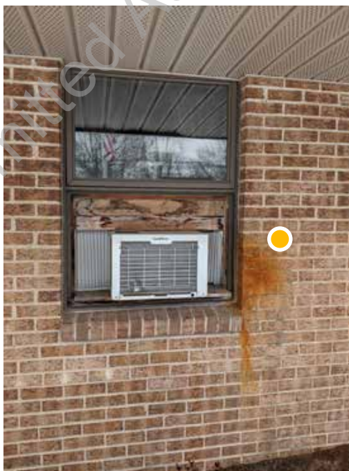
● D1. 6: Window air conditioning unit requires permanent installation solution; has caused staining on adjacent brickwork
