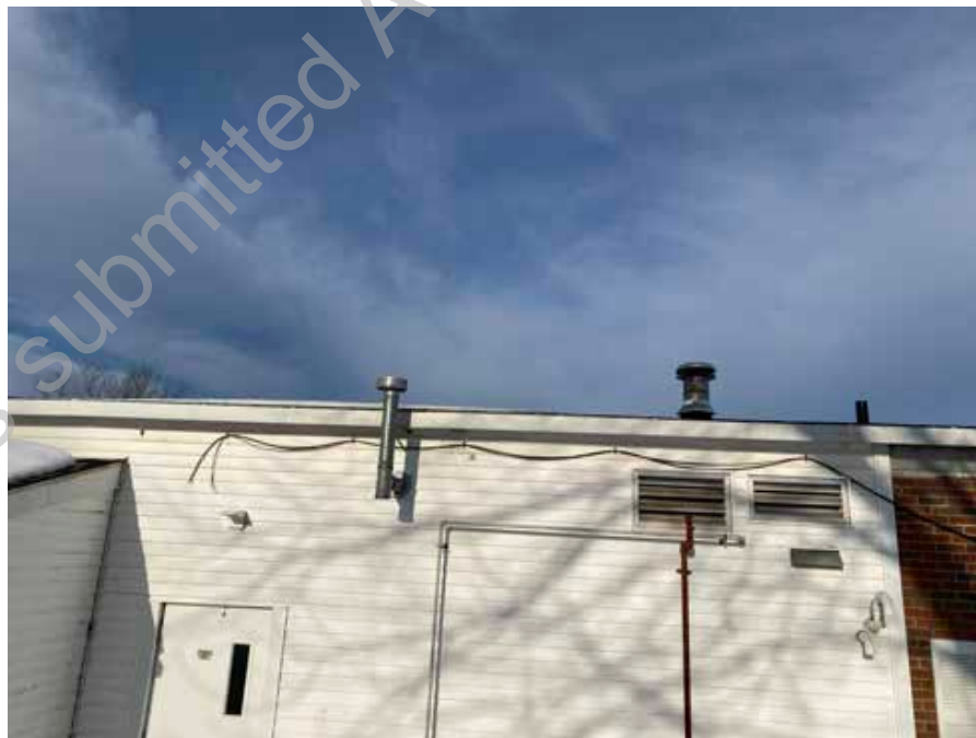
● D2. 16: Exhaust Fan and Vent on Roof
