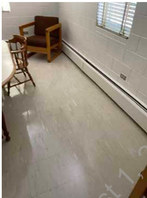
● D2. 15: Hot Water Fin Tube Radiation
