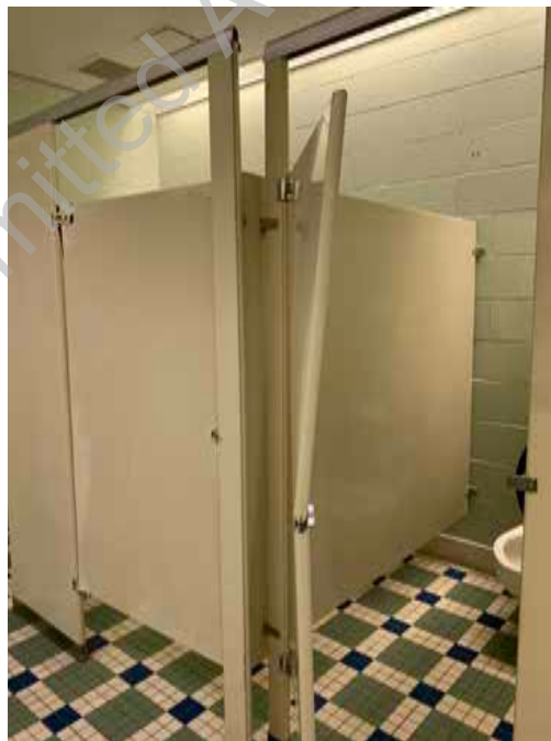
● D1. 50: Detail view of typical toilet room, note damaged metal toilet partition.
