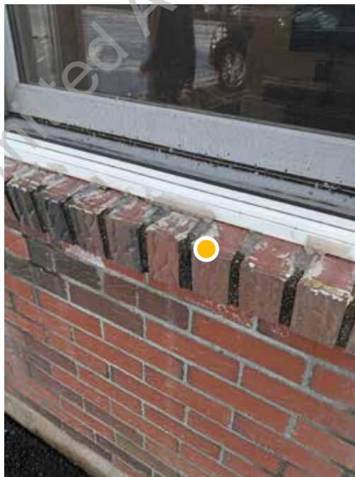
● D1. 10: Staining and poorly installed caulk at brick window sills
