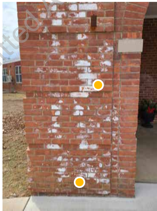
● D1. 4: Detail view of masonry arch with efflorescence and related deterioration at base of wall.
