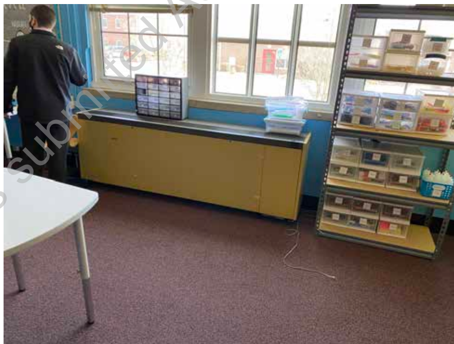
● D2. 38: Detail view of typical unit ventilator in educational spaces.
