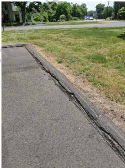
● D3. 18: Bituminous asphalt curbing is damaged at most locations
