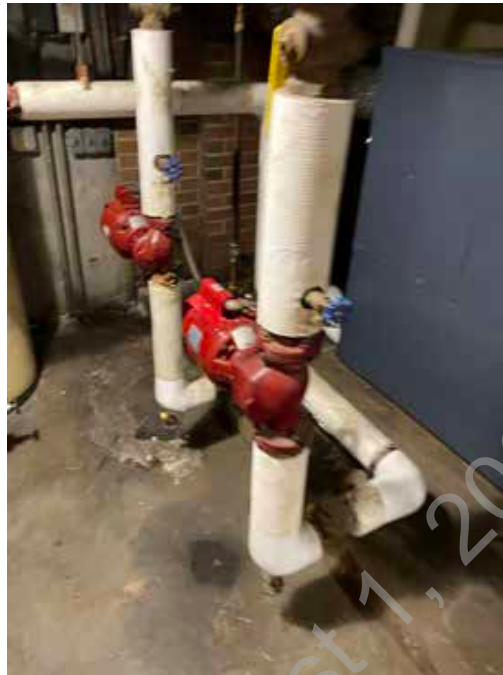
● D2. 19: Hydronic Hot Water Pumps
