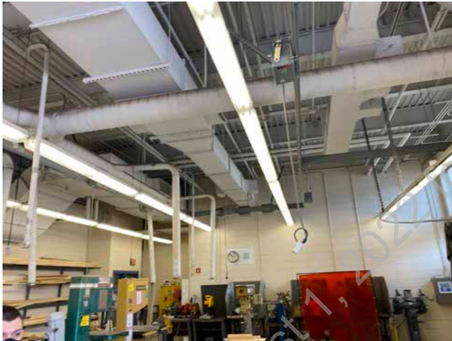
● D2. 13: Exposed Ductwork in Shop in Good Condition
