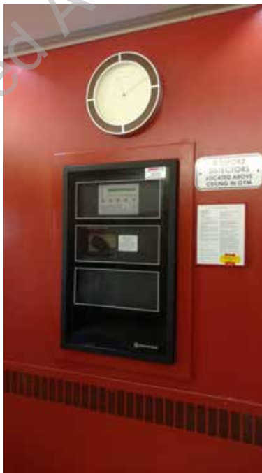
● D2. 16: Fire Alarm Control Panel.
