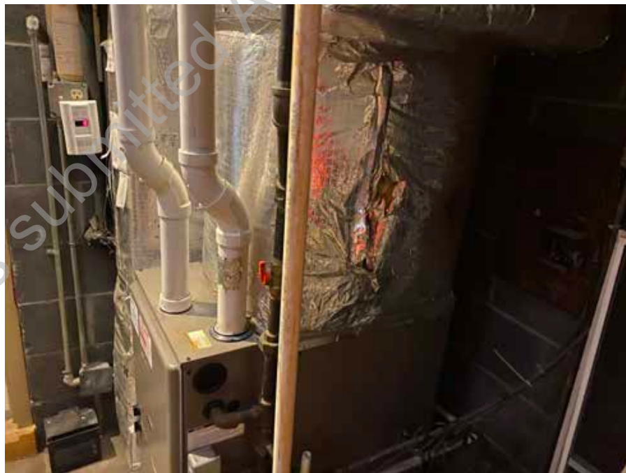
● D2. 20: Furnace Ductwork and Refrigerant Piping in Fair Condition
