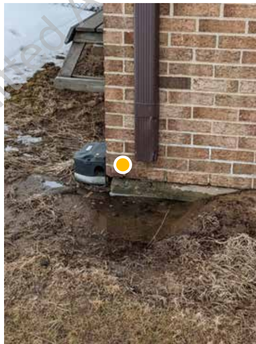
● D3. 4: Missing splash block at downspout locations causing soil erosion; Concrete foundation has begun spalling
