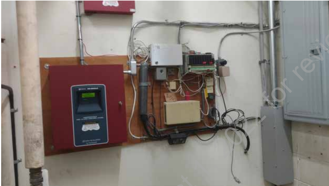
● D2. 29: Telephone Service Demarc
