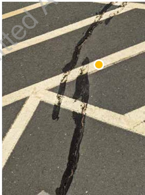
● D3. 4: Cracking throughout parking area and drive aisles has been patched
