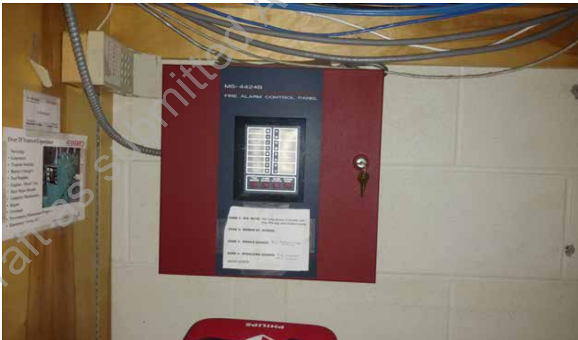
● D2. 8: Fire Alarm Control Panel Monitoring Only)
