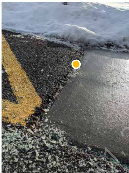
● D3. 1: Corrosion of pavement at base of entrance ramp
