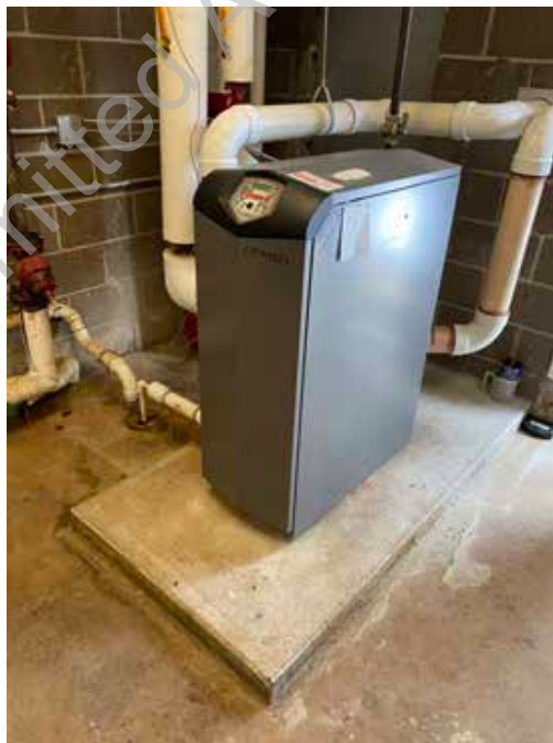
● D2. 32: Lochinvar Natural Gas Hot Water Boiler
