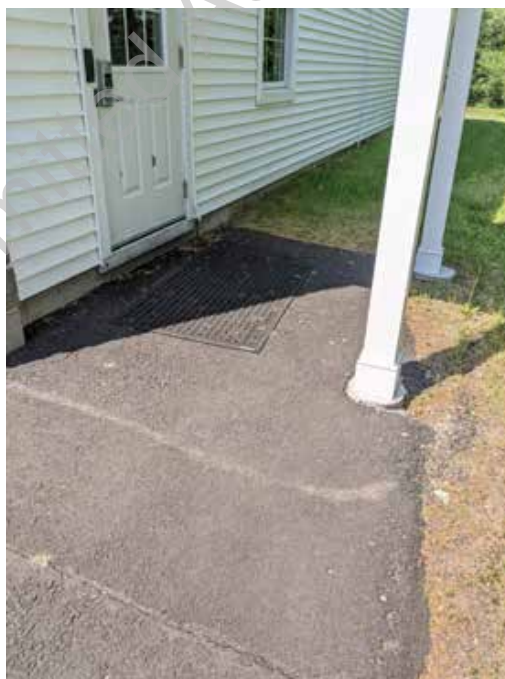
● D3. 10: Bituminous concrete paving at North entrance is beginning to show cracking
