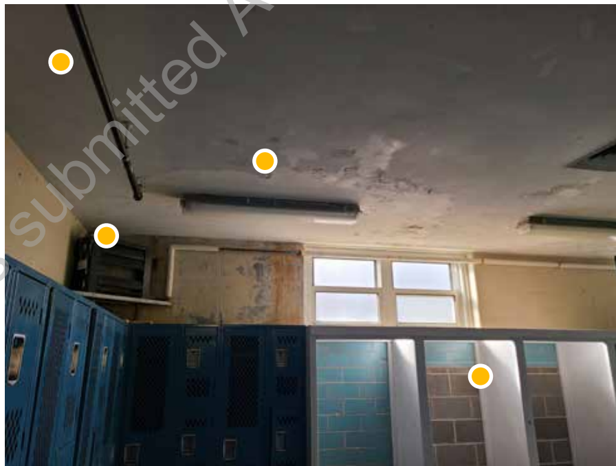
● D1. 40: Detail view of changing area retrofit in boys locker room, note poor condition of walls, ceilings, and exposed equipment and piping (original to the building).
