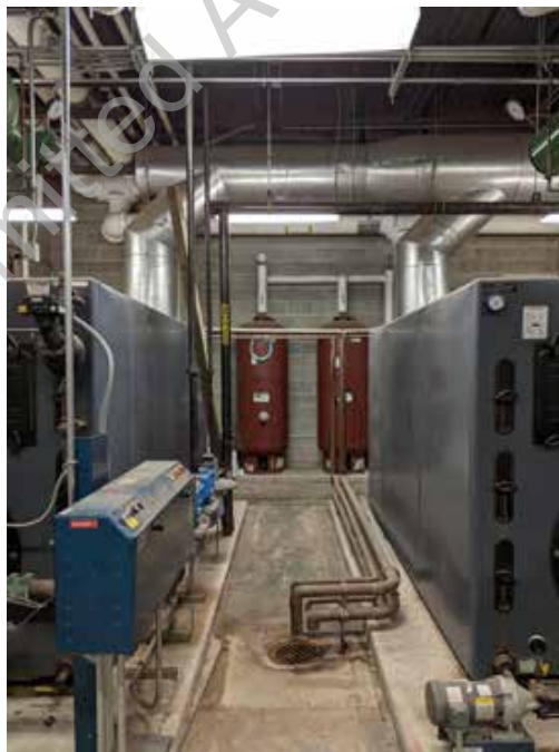
● D1. 102: View of mechanical room with floor drain (center) for condensate & drain lines.
