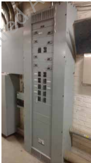
● D2. 10: Electric Main Distribution Switchboard.
