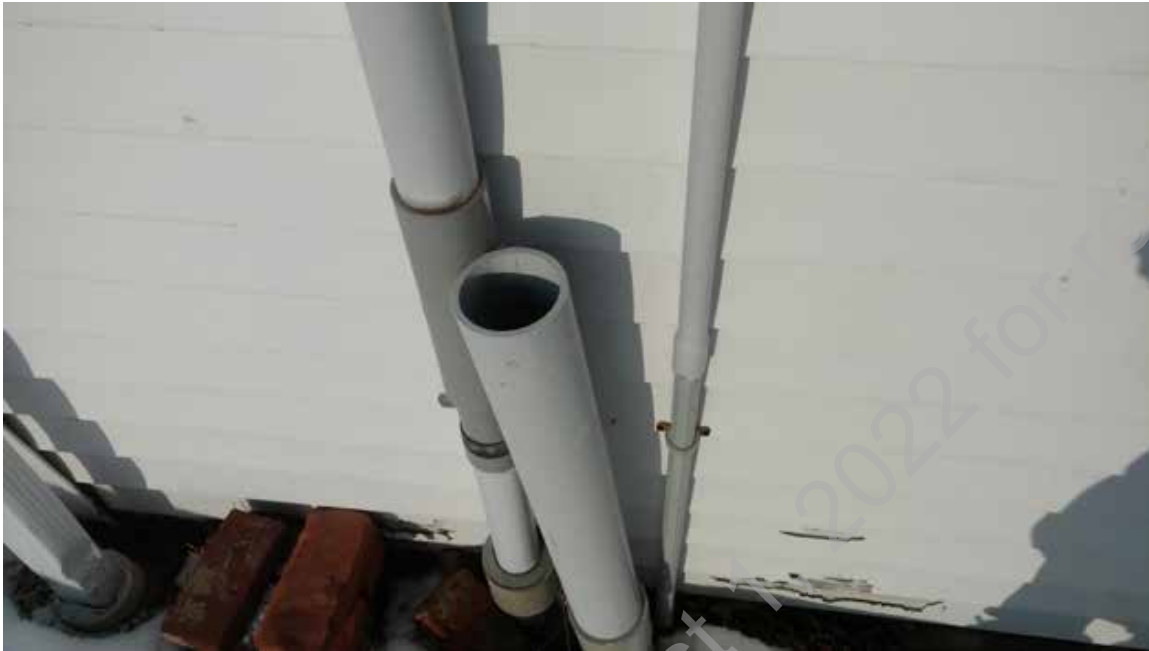
● D2. 17: Exterior Communication Conduit
