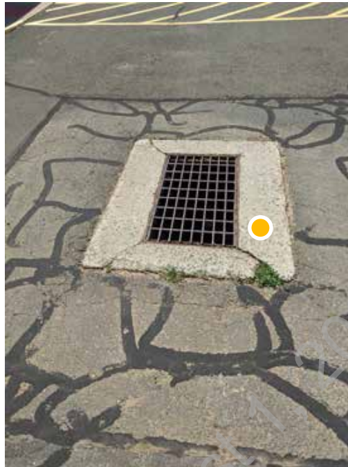
● D3. 15: Cracking and edge chipping at concrete basin top in parking area
