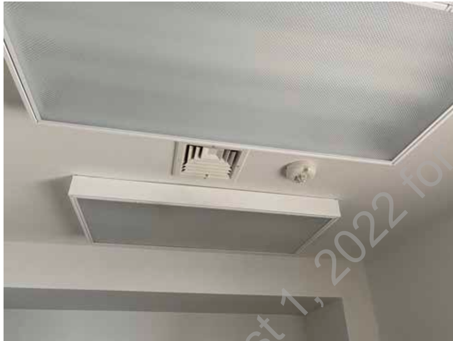
● D2. 5: Diffuser Served by a Fan Coil Unit
