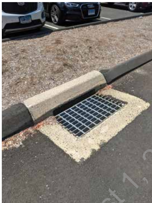
● D3. 11: View of typical precast curb/catch basin
