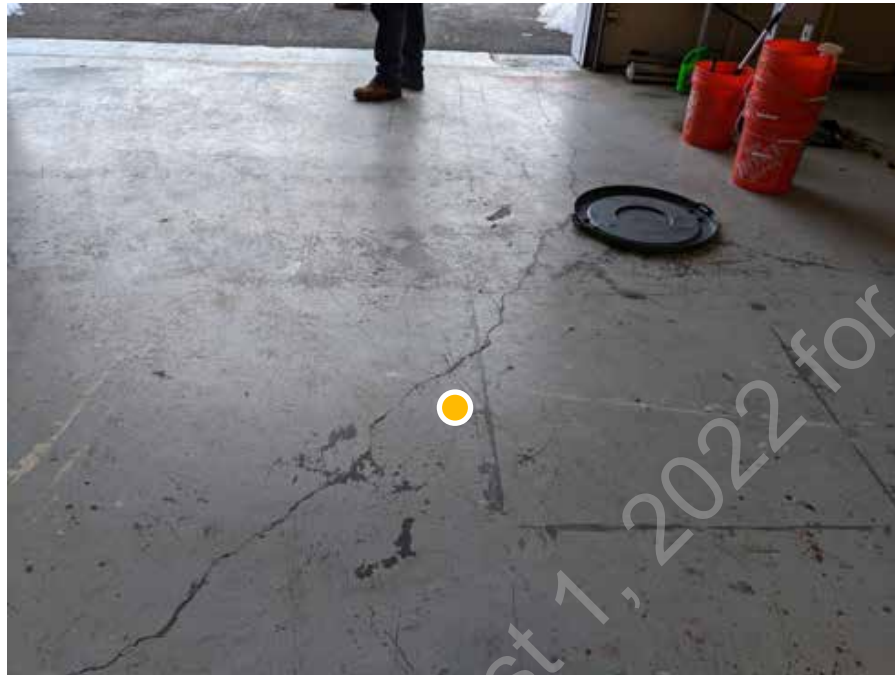
● D1. 99: Detail view of concrete slab cracking/deterioration likely caused by settlement and/or shrinkage.
