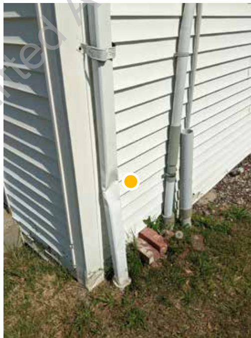
● D1. 20: Downspout damaged
