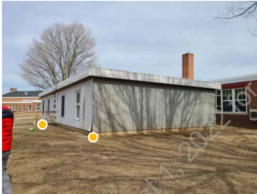
● D1. 15: Corner view of the modular classroom building with modified ramp entry shown (left). Note deterioration of T-111 siding.
