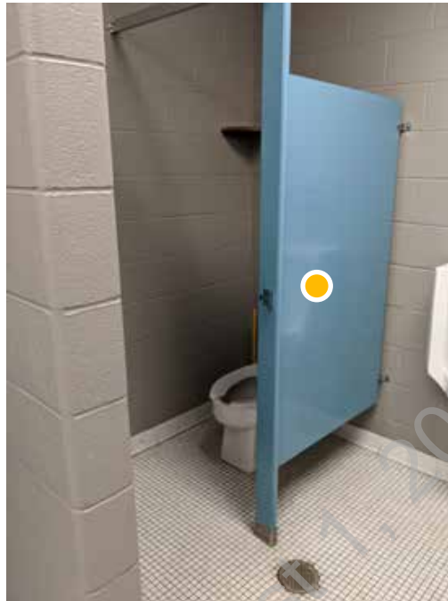
● D1. 19: Toilet stalls do not have required clear space to be considered accessible
