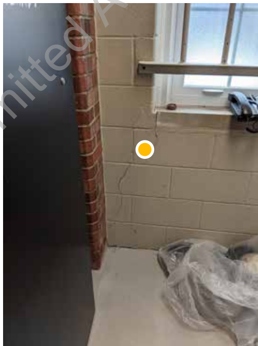
● D1. 26: Cracking of concrete masonry unit walls observed throughout
