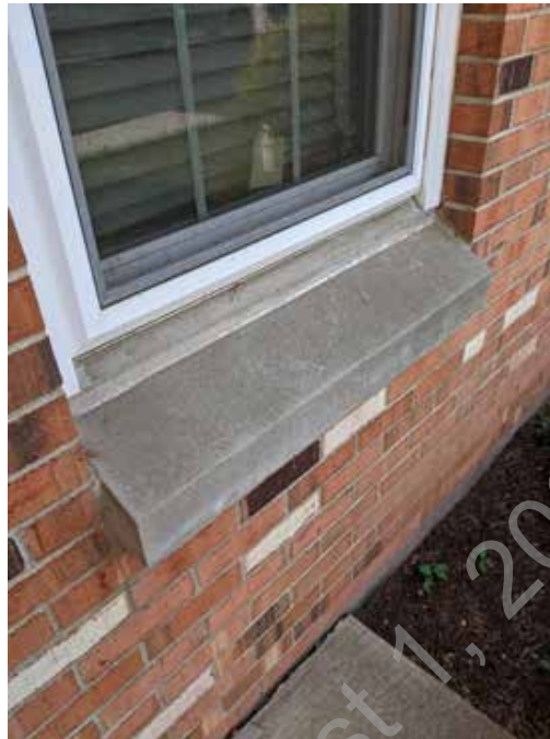
● D1. 11: Concrete window sill
