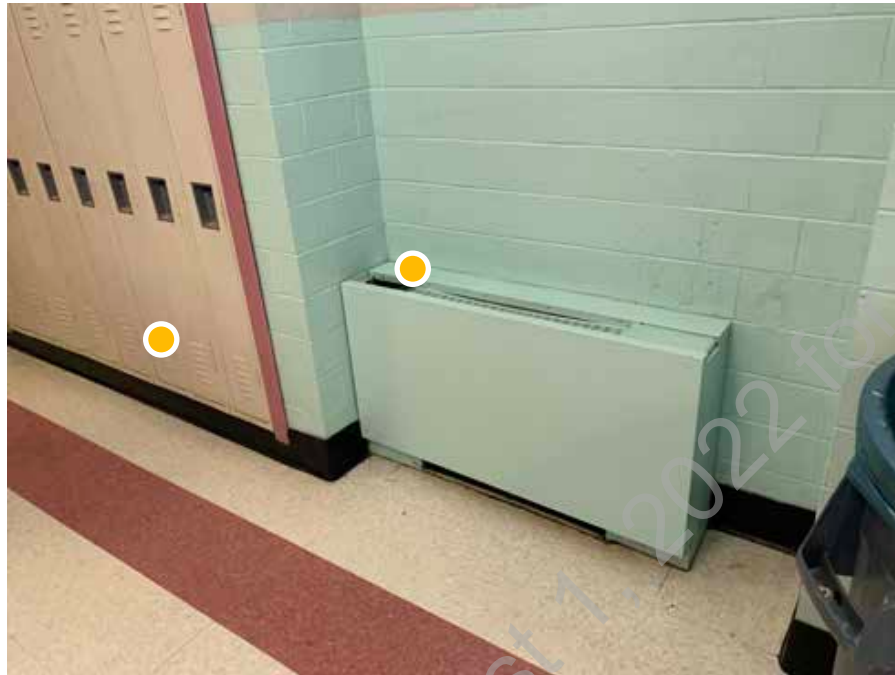
● D1. 35: Typical classroom corridor with metal lockers and unit cabinet heater (poor condition overall)
