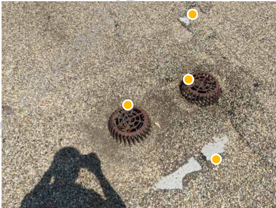
D1. 10: View of built up roofing with double roof drain, note portions of the roof have exposed built up with limited gravel protection.
