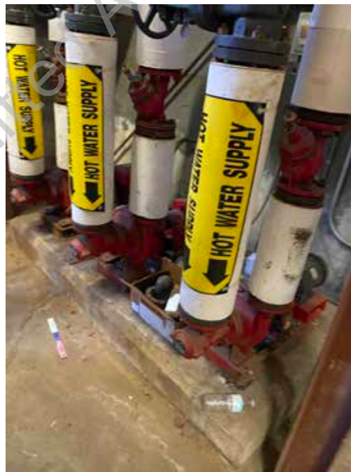
● D2. 18: Hot Water Supply Pumps in poor condition.
