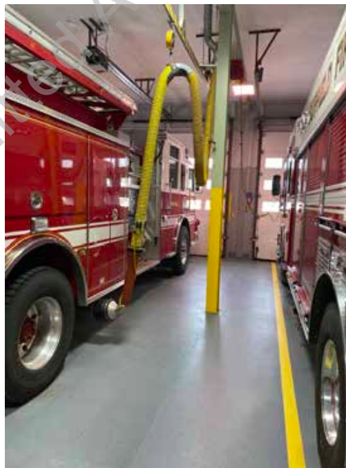
● D2. 36: Plymovent Exhaust
