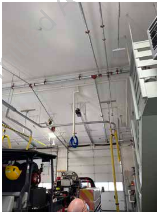
● D2. 14: Fire protection Sprinkler System in App Bay
