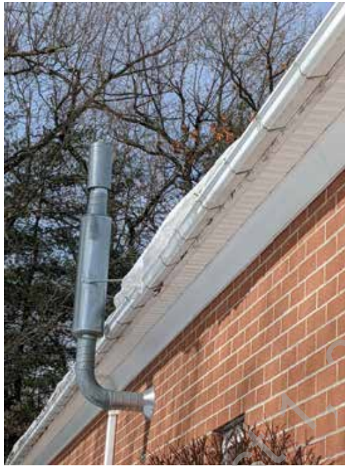
● D1. 5: Ice and snow build up at gutter system
