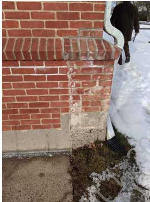
● D1. 11: Detail view of masonry; appears to be poorly patched
