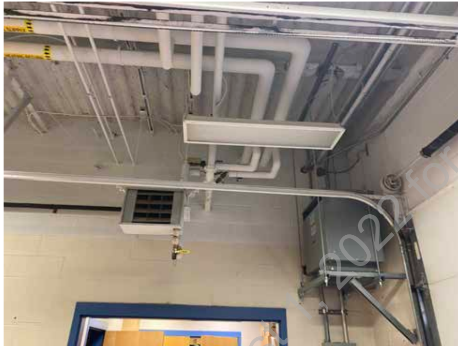
● D2. 27: Hot Water Unit Heater in Poor Condition
