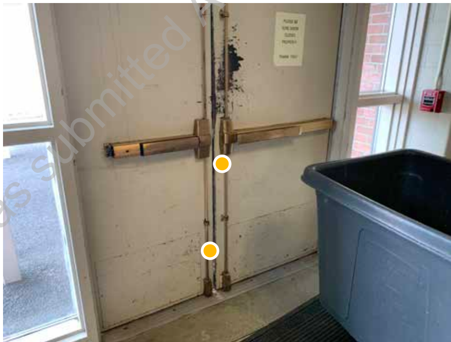
D1. 26: Detail view of typical exterior double door assembly. Note the overall poor condition and gaps in the perimeter.
