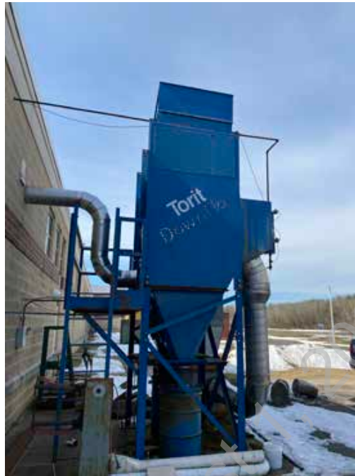
● D2. 51: Torit Downflo Garage Exhaust System
