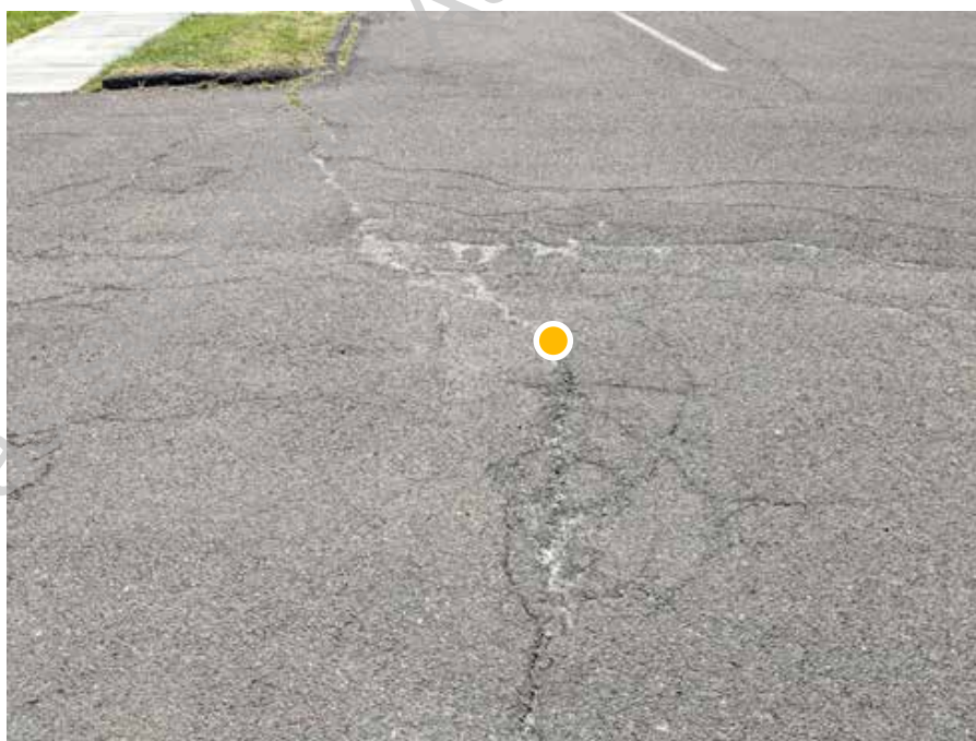
● D3. 2: Cracking pavement throughout parking areas and drive aisles
