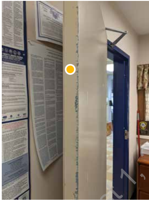
● D1. 29: Office doors need adjustment to prevent rubbing on frames
