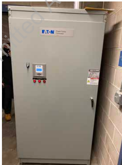
● D2. 42: Power Factor Correction Capacitor Bank
