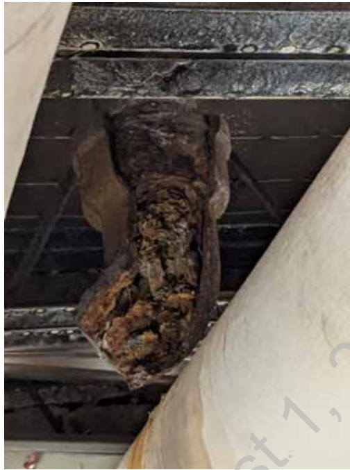
● D1. 57: Abandoned Floor Drain.
