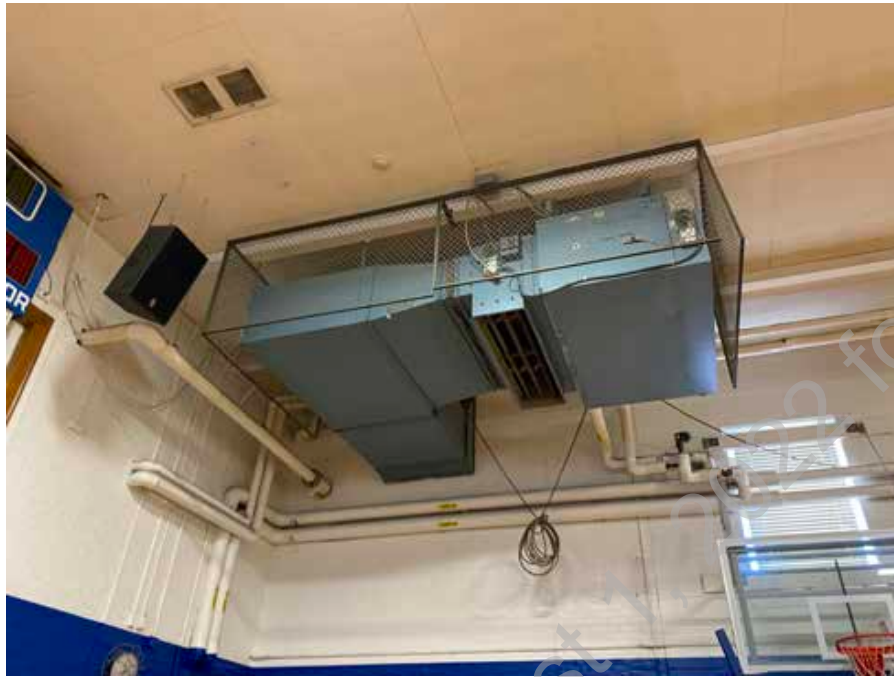
● D2. 15: Heating and Ventilating Unit Serving Gymnasium.
