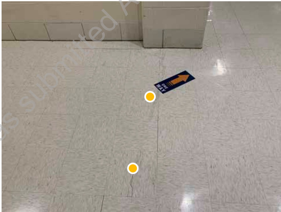
D1. 34: Detail view of the VCT flooring with stress cracks and indications of settlement in multiple locations.
