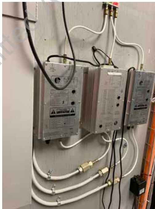
● D1. 112: Cable Broadband Distribution Amplifiers
