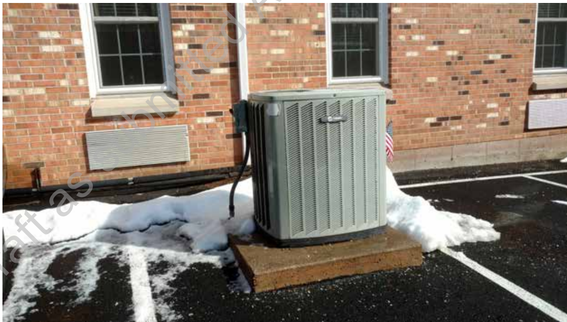
● D2. 28: Second Trane Condensing Unit Servinf Indoor Air Handler
