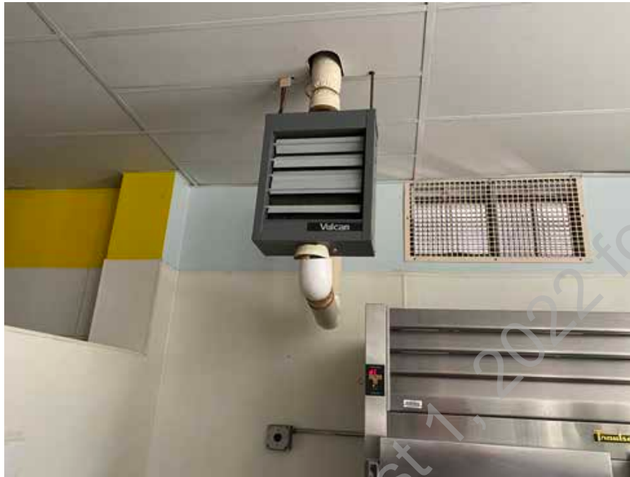
● D2. 19: Hot Water Unit Heater Serving Kitchen.
