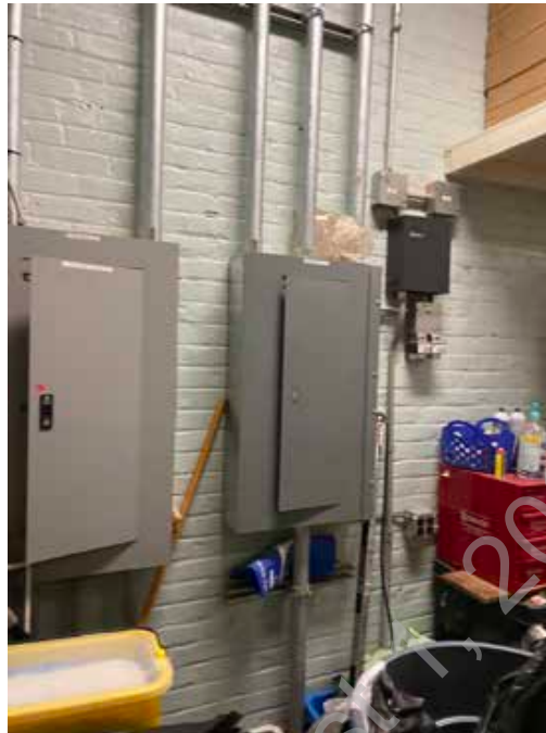
● D2. 5: Electrical Branch Circuit Panels.
