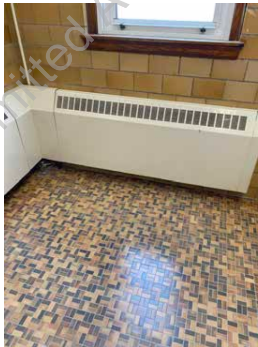
● D2. 16: Hot Water Fin Tube Radiation in poor working condition.
