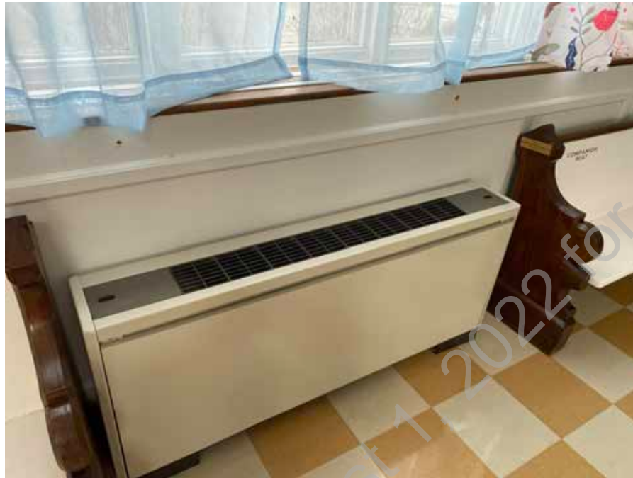
● D2. 29: Indoor Heat Pump Unit in Good Condition
