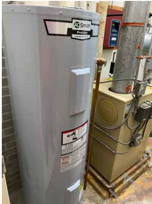
● D2. 7: Electric Domestic Water Heater
