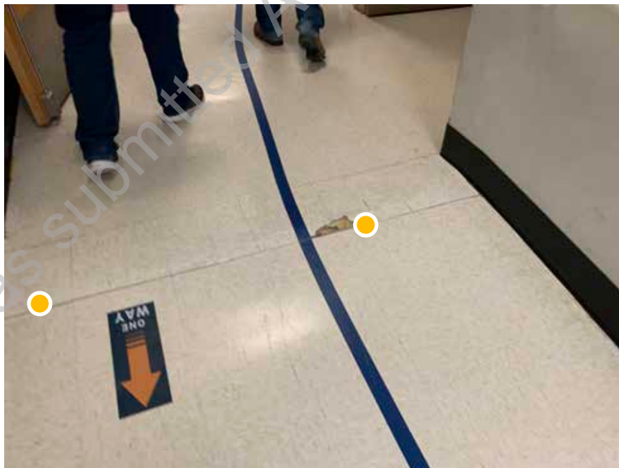
● D1. 34: Typical VCT flooring in corridors, note the deterioration, missing and/or broken tile at the expansion joints between building additions.
