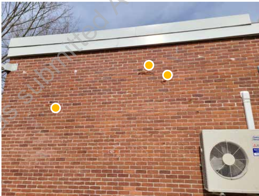
● D1. 14: Detail view of 1988 classroom addition with brick spalling and deterioration of masonry joints.
