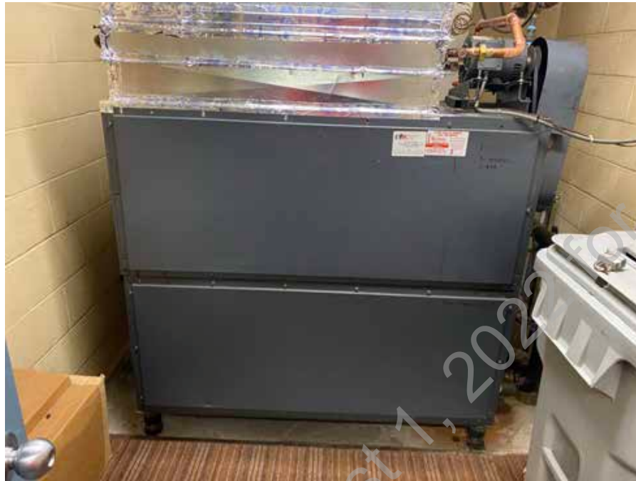
● D2. 13: Indoor Air Handler (HAC 2) in Poor Condition
