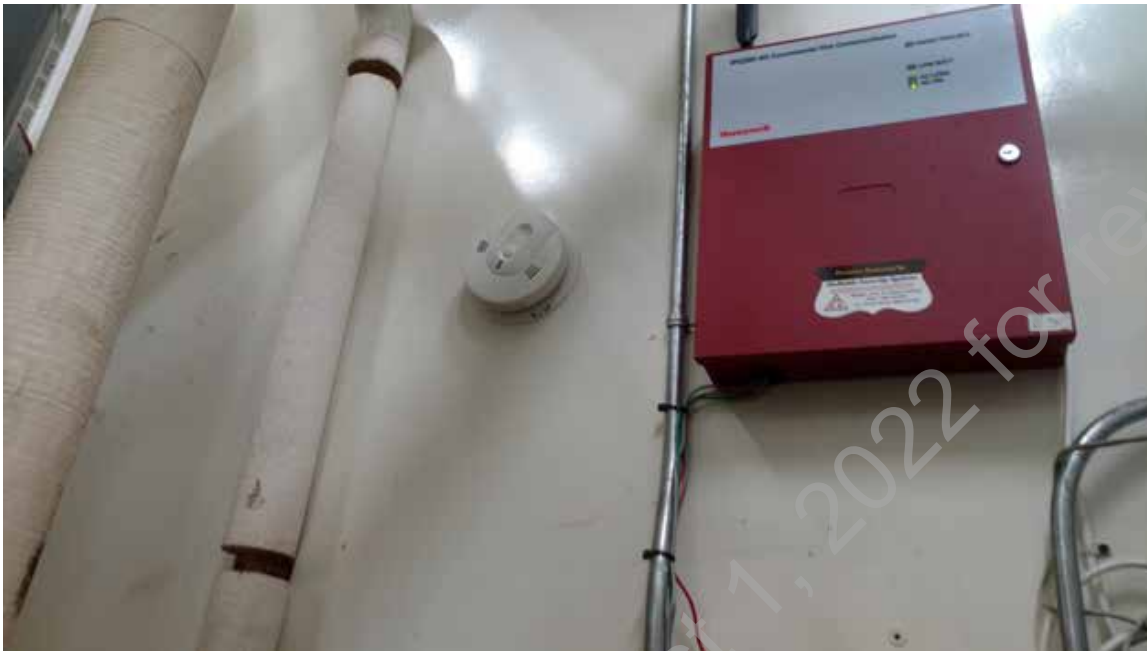
● D2. 27: Smoke Detector and Fire Alarm Communicator
