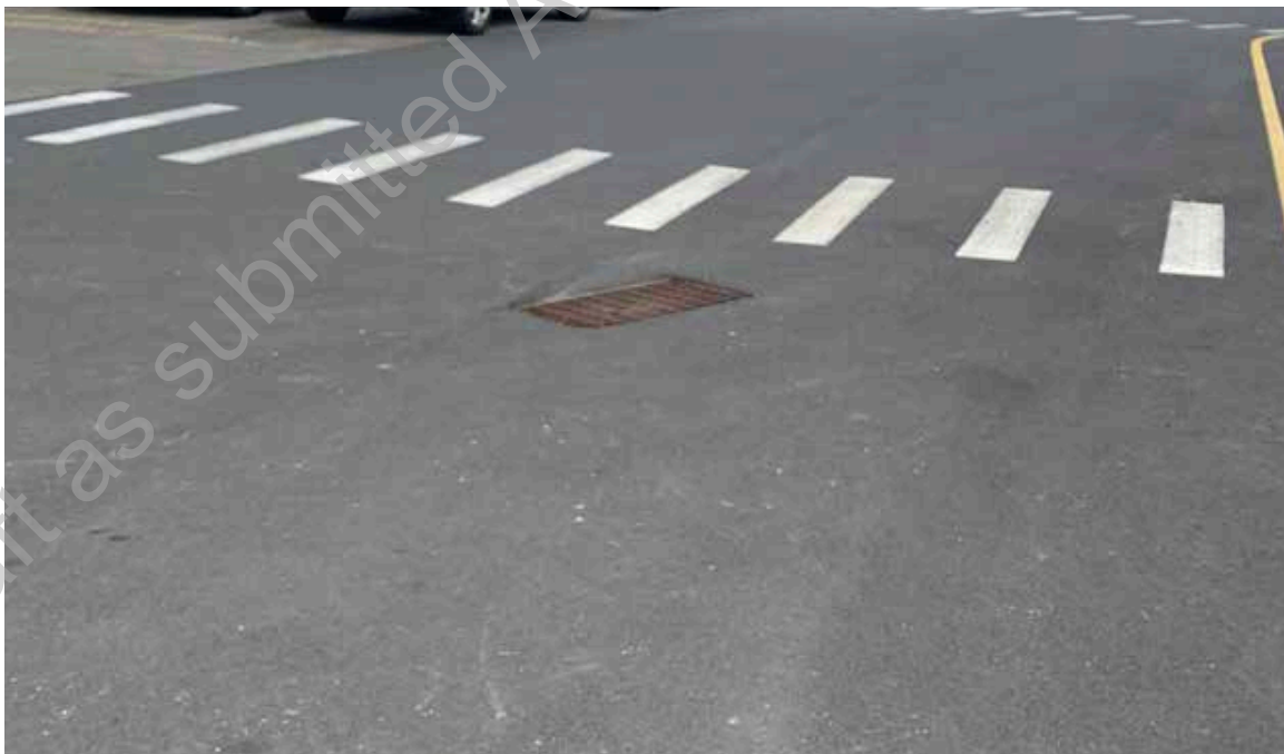
● D3. 14: View of repaired/paving replacement at main entrance drive. Storm water collection system as originally installed.
