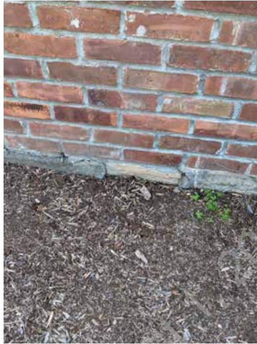
● D1. 23: Spalling concrete foundation at perimeter
