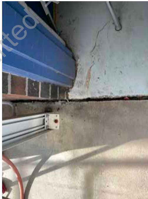
● D1. 60: Detail view of greenhouse/building intersection, note gap in expansion joint and condition of greenhouse frame system
