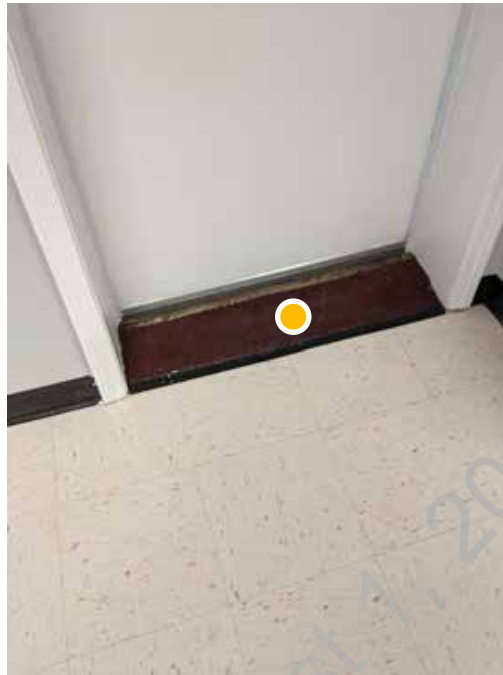
● D1. 39: Mismatched flooring at door threshold in break area
