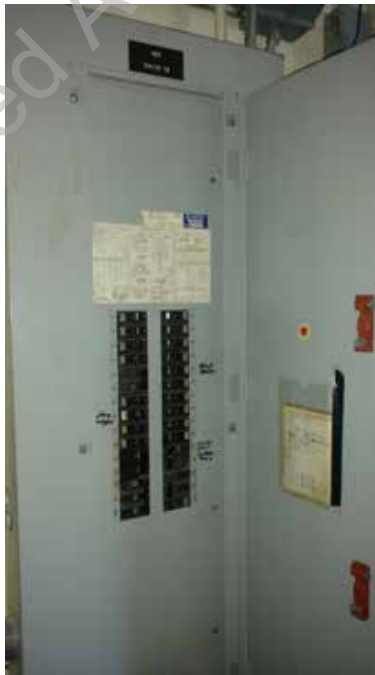
● D2. 6: Electrical Branch Circuit Panel
