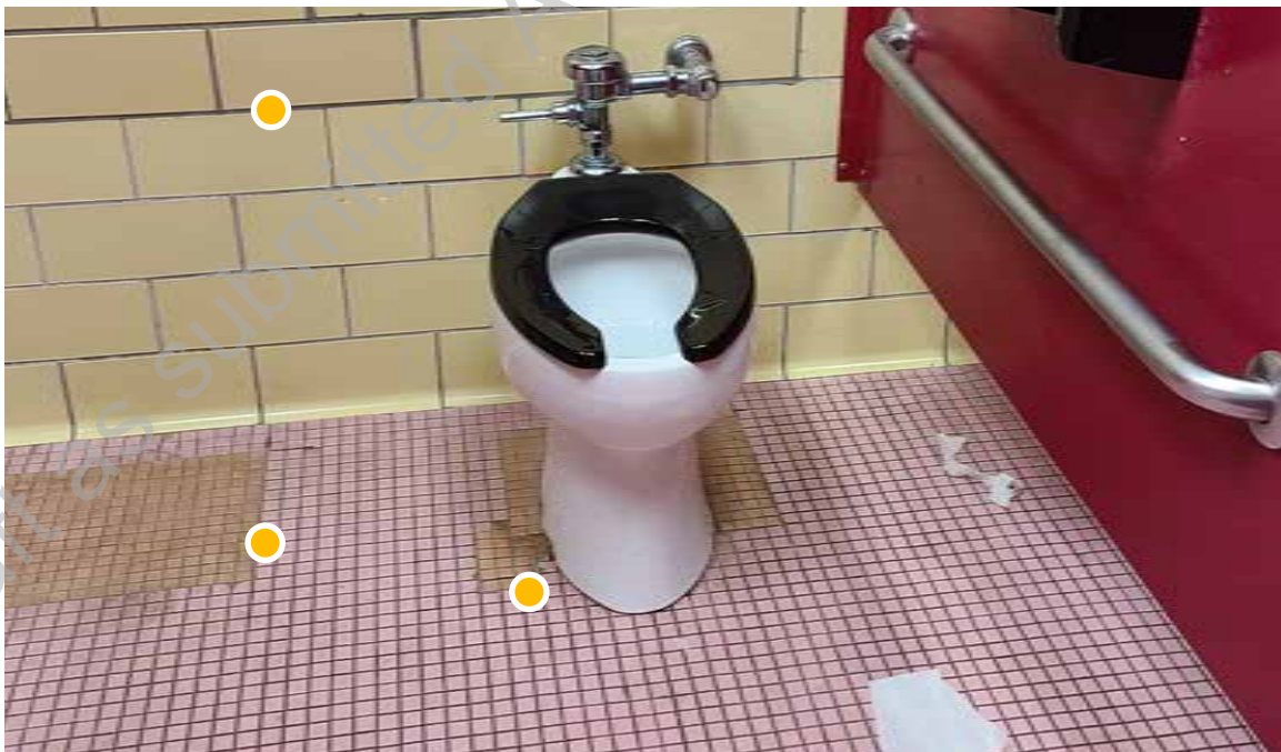
● D1. 56: Typical original bathroom with modified toilet location for ADA accessibility. Missing rear grab bar. Note the patched tile work on both wall and floor.
