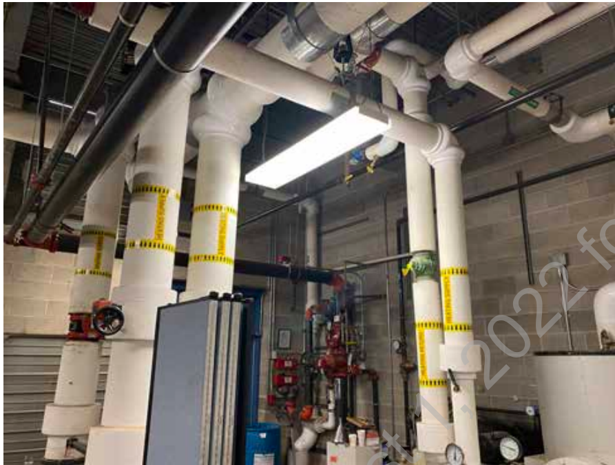
● D2. 25: Hot Water Piping in Good Condition
