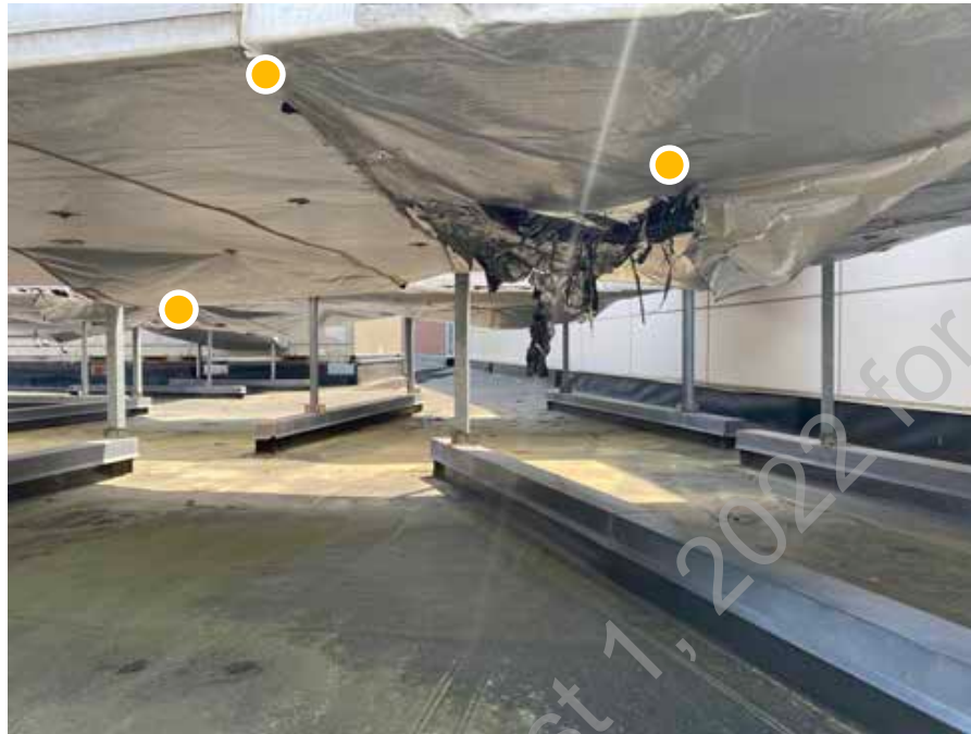
● D2. 43: View of the underside of the roof mounted ductwork, insulation wrap is in poor condition overall.
