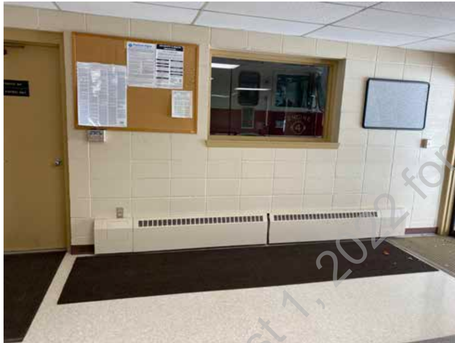
● D2. 11: Hot Water Fin Tube Radiation Needs Replacement
