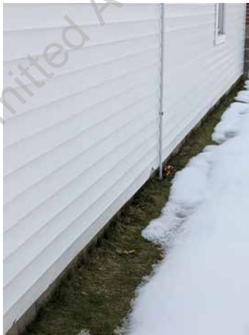
● D1. 6: Damaged vinyl siding at base
