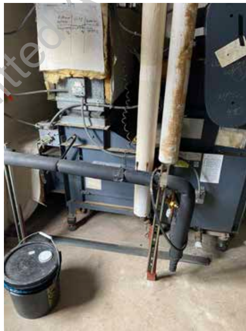
● D2. 14: Indoor Air Handler in Mechanical Room Needs Replacement
