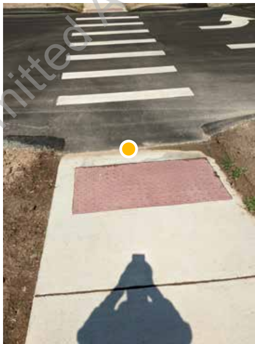
● D3. 6: A low point was observed between concrete sidewalk and parking area and may collect water
