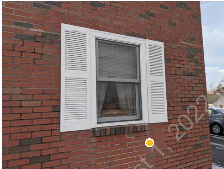
● D1. 5: Aluminum windows with brick sill; Brick staining
