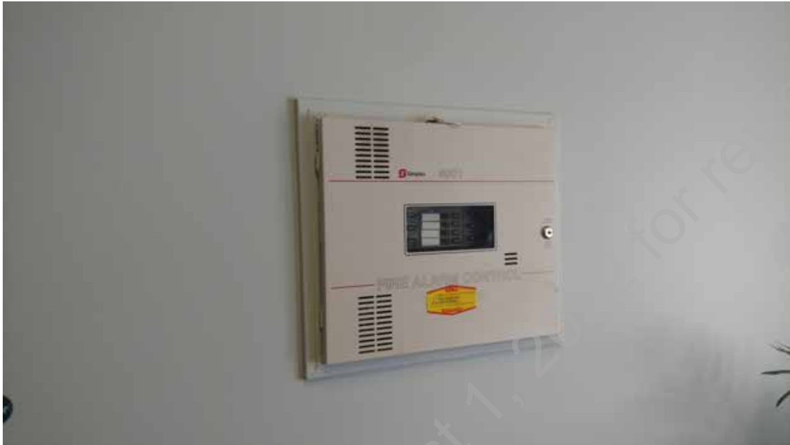
● D2. 19: Fire Alarm Control Panel
