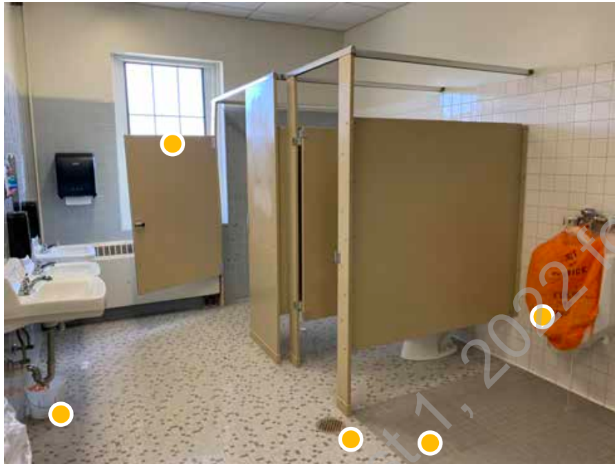
● D1. 33: View of typical bathroom space, note non functioning fixtures, broken and/or deteriorated toilet partitions, and buckets to prevent sink leaks. Also note indication of previous modifications to space via the different floor tiles.
