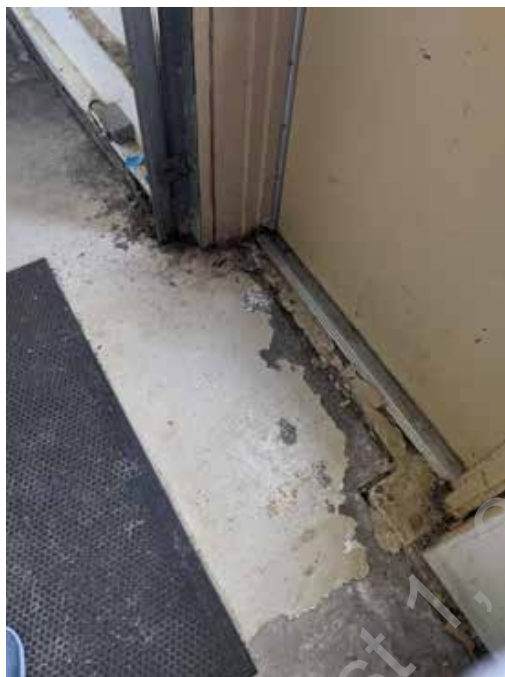
● D1. 37: Damaged vinyl tile flooring in storage garage
