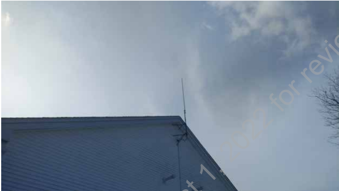
● D2. 11: Fire Alarm Communicator Antenna
