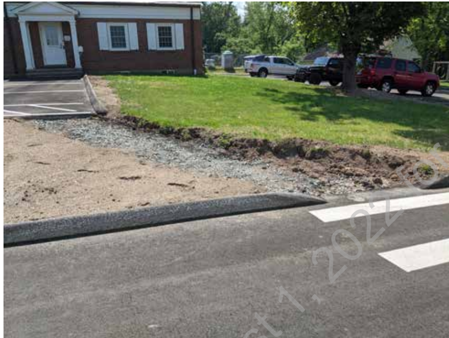
● D3. 3: New sidewalk substrate has been prepared but was not completed at the time of walkthrough
