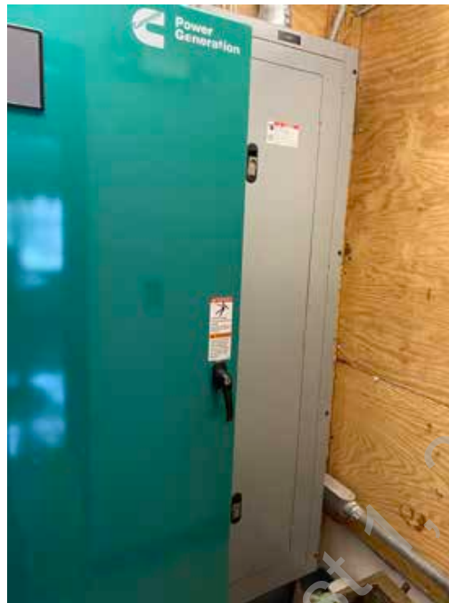
● D2. 11: Electrical ATS and Distribution Panel
