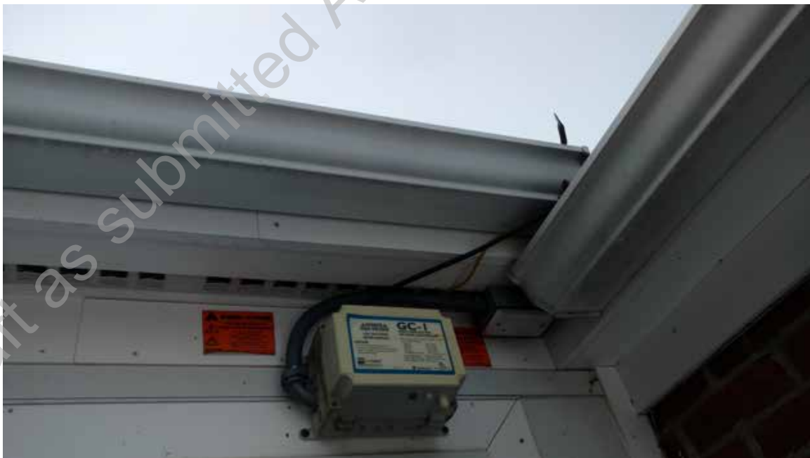
● D2. 42: Rain Gutter De-Icing Equipment
