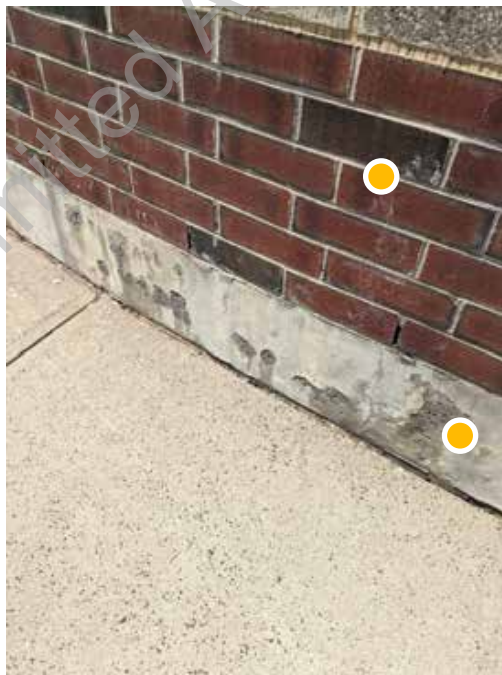
D3. 20: Detail view of typical screen wall, note deterioration of masonry jointing, efflorescence, and spalling at concrete foundation wall.
