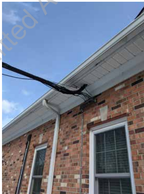
● D1. 8: Radio tower feed into Police Station
