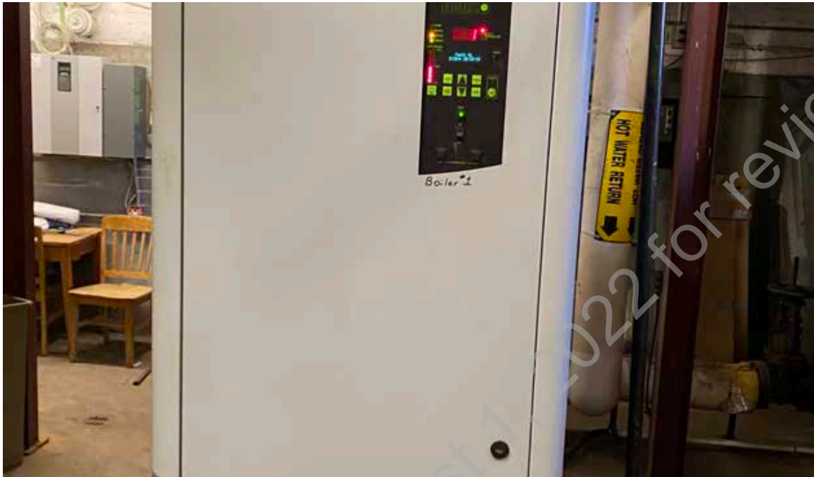
● D2. 1: Aerco Natural Gas Condensing Boiler in good condition.
