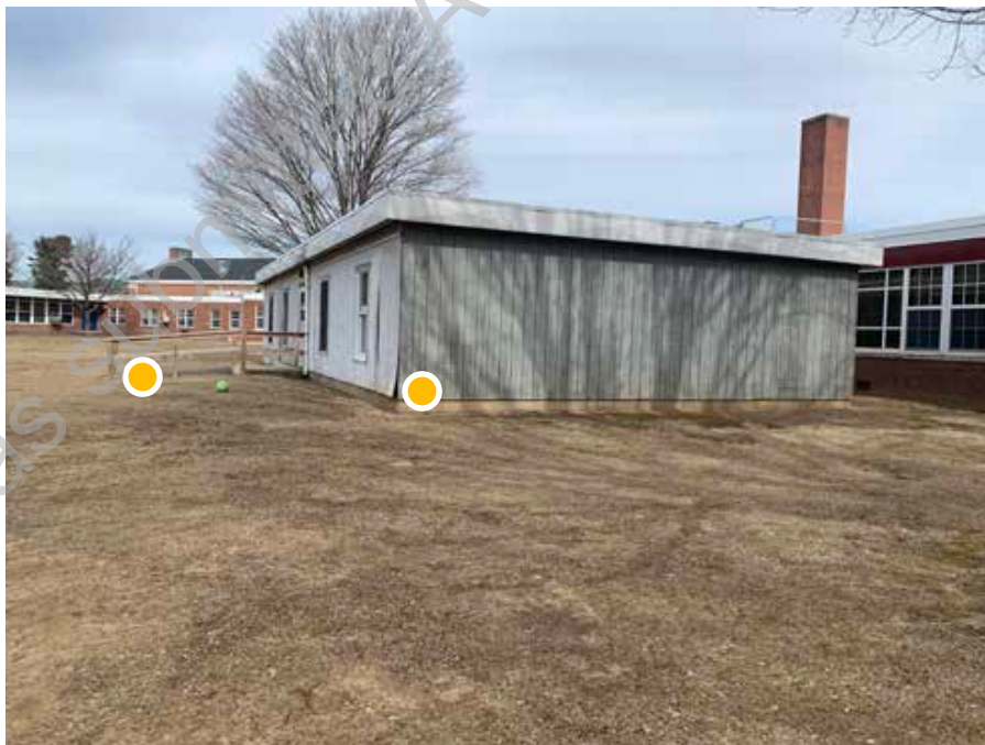
● D1. 26: View of 1985 modular classroom building. Note deterioration of the T-111 siding and non compliant ADA access ramp.
