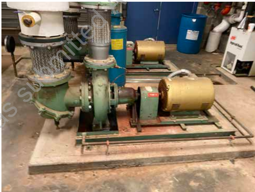
● D2. 26: Hot Water Pumps in Poor Condition
