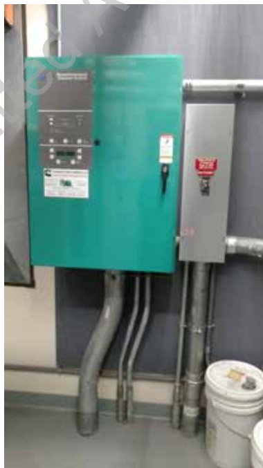
● D2. 2: Automatic Transfer Switch
