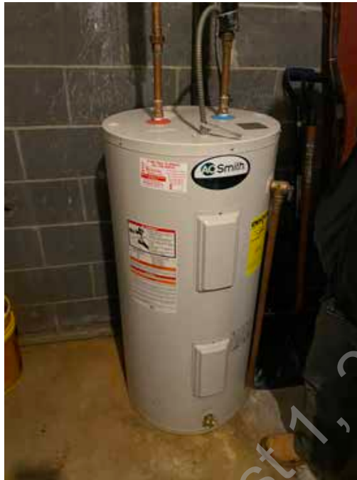
● D2. 5: Electric Domestic Hot Water Heater Located in Mechanical Room
