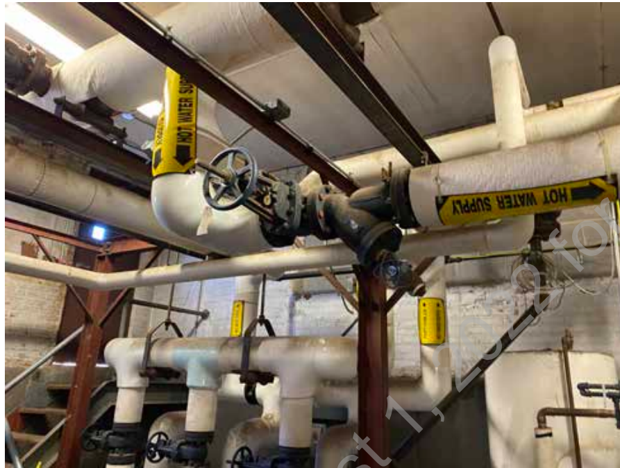
● D2. 17: Hot Water Piping in poor condition.
