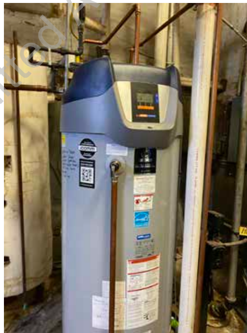
● D2. 30: Natural Gas Domestic Hot Water Heater.
