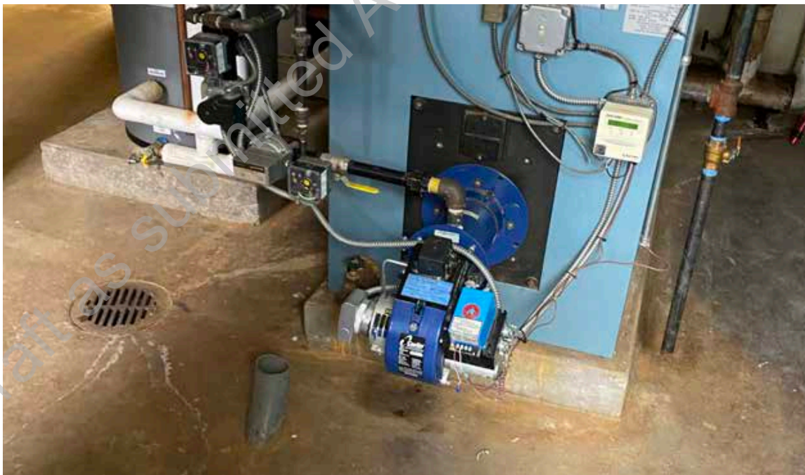
● D2. 20: Natural Gas Hot Water Boiler
