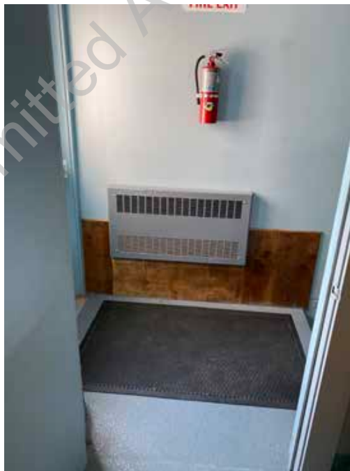
● D2. 18: Hot Water Wall Convector Needs Replacing
