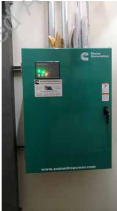
● D2. 2: Automatic Transfer Switch
