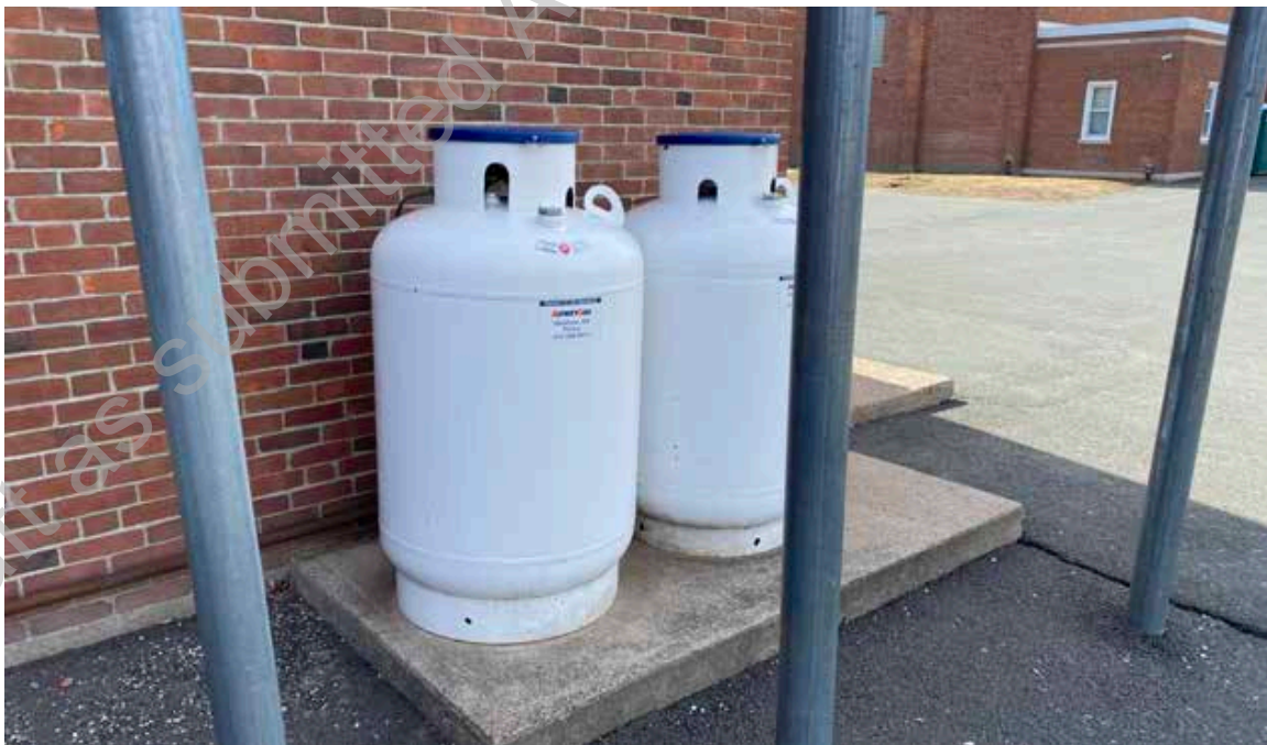
● D2. 2: AmeriGas Propane Tanks Serving Kitchen Equipment.
