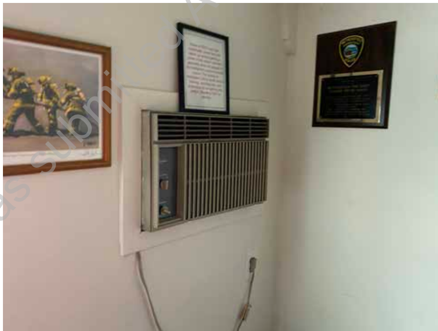
● D2. 42: Thru Wall AC Unit in Poor Condition
