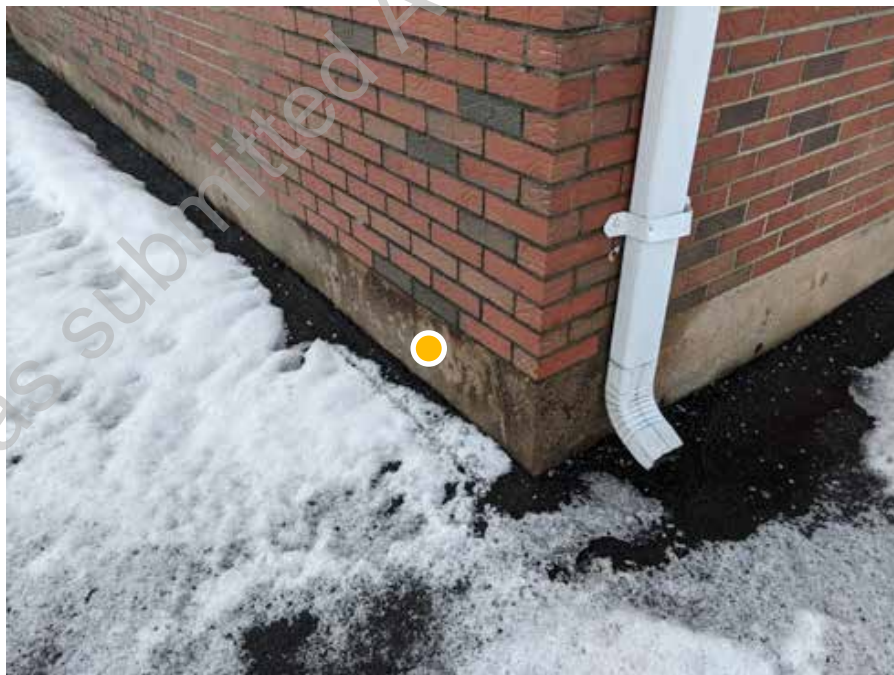
● D1. 6: Brick and concrete staining at base
