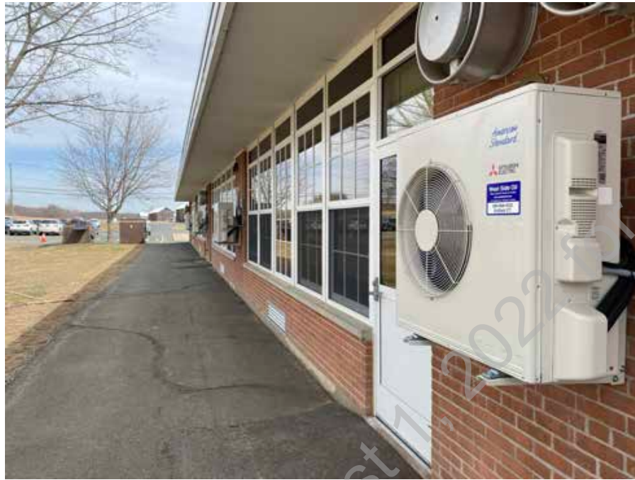
● D2. 31: Row of Condensing Units Serving Split Units in Each Classroom.
