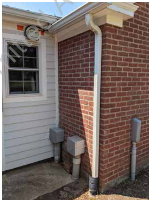
● D1. 22: Detail view of interior corner; a gap is present at the joint between brick and vinyl siding
