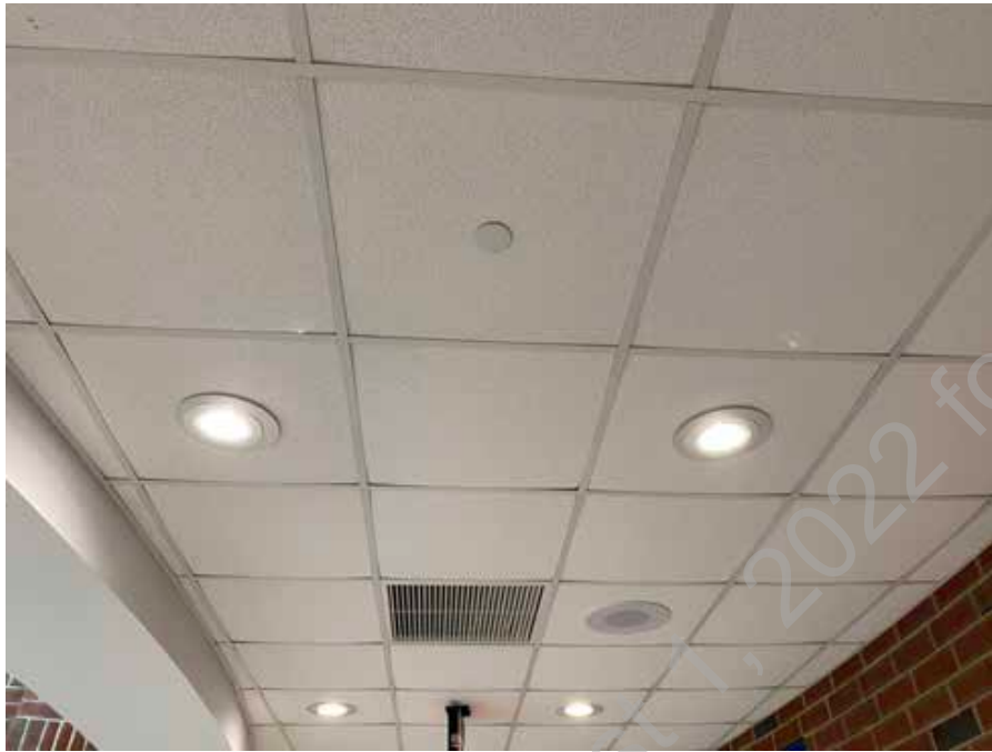
● D2. 9: Electrical Recessed Downlighting
