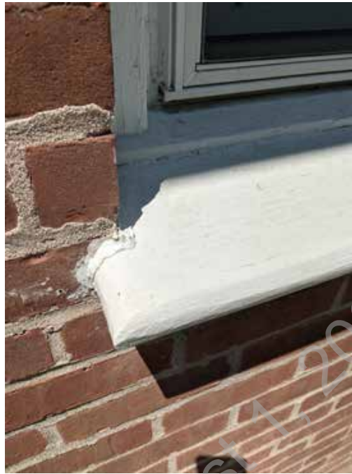
● D1. 19: Wood windows are poorly caulked
