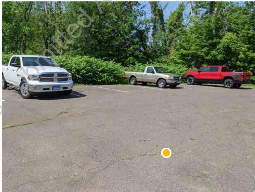
● D3. 12: Cracking pavement throughout parking areas and drive aisles
