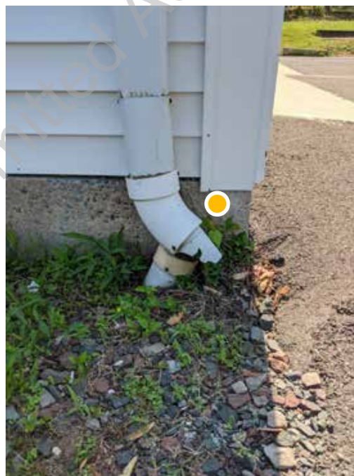
● D1. 18: Damaged downspout at connection to sub-surface drainage system
