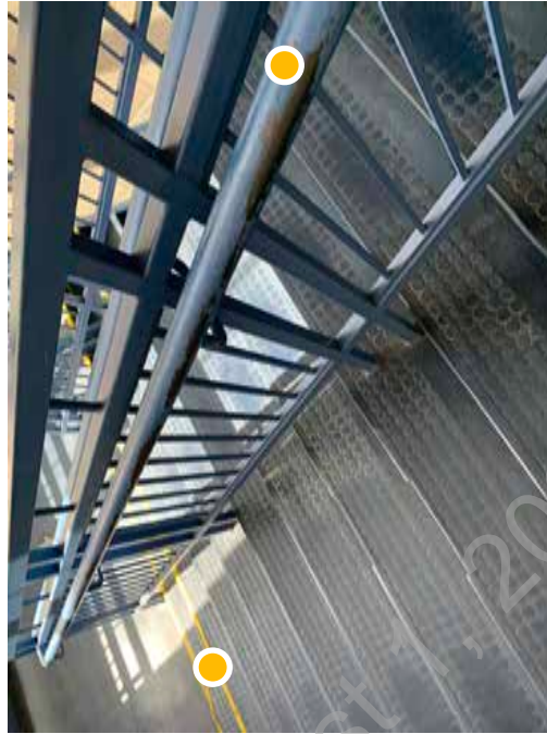
● D1. 55: Detail view of the rubber treads/risers and painted steel handrail/guard at egress stairwell, note poor age/condition due to continual use.
