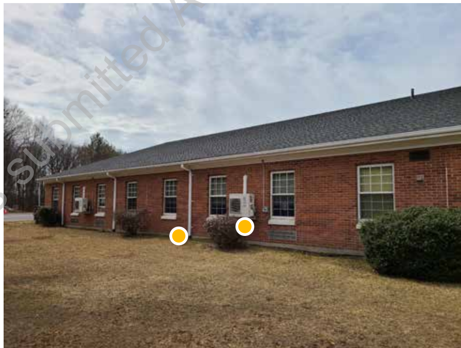
● D1. 12: Overall view of 1988 addition, note rain leaders connected to storm water collection system and retrofit wall mounted air conditioning units.
