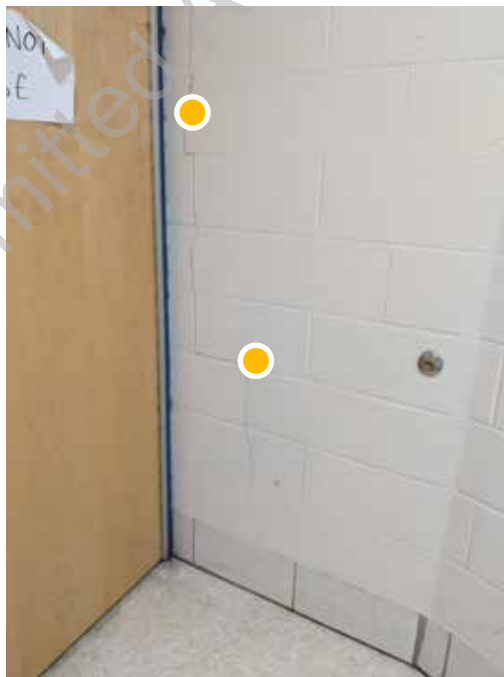
● D1. 70: Detail view of stress fractures in the CMU block wall likely due to building settlement.
