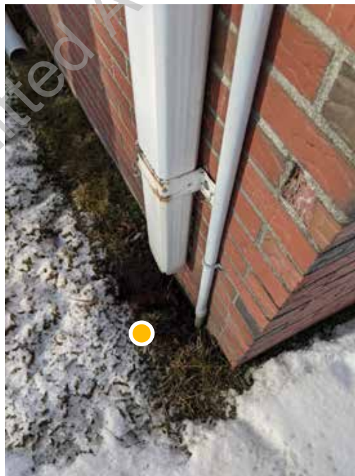
● D1. 12: Missing splashblock causing soil erosion
