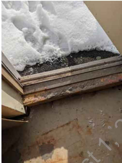
● D1. 41: Spalling concrete sill at exterior door in storage garage
