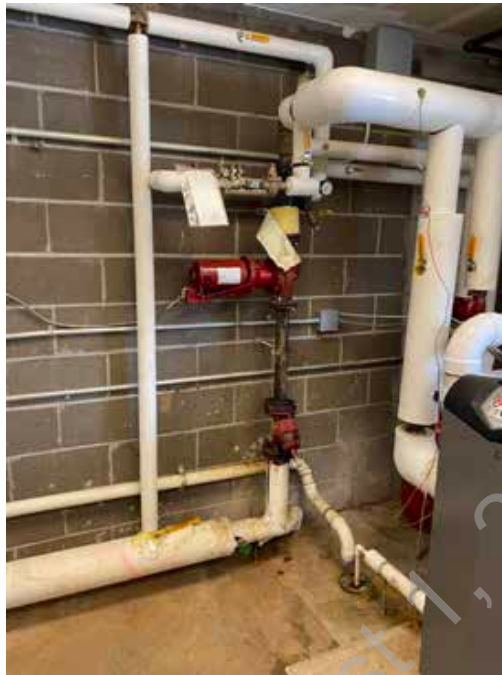
● D2. 27: Hot Water Pumps and Piping in Good Condition
