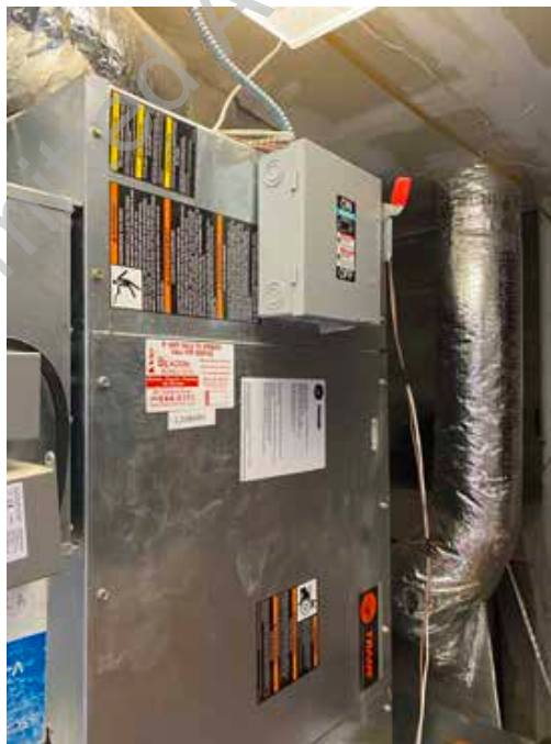
● D2. 44: Trane Fan Coil Unit Serving the Library
