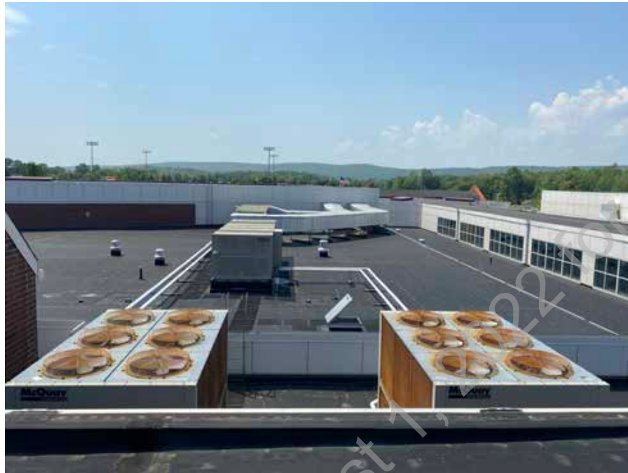
● D2. 39: McQuay Rooftop Units and Exposed Ductwork in Fair Condition
