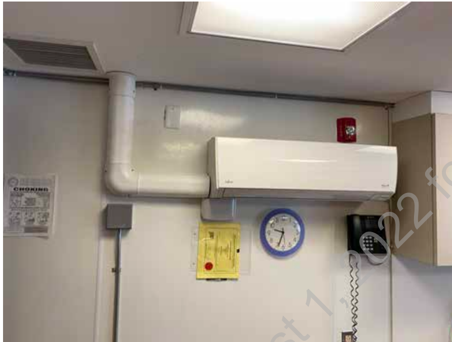
● D2. 23: Fujitsu Wall Mounted Split Unit in Good Condition
