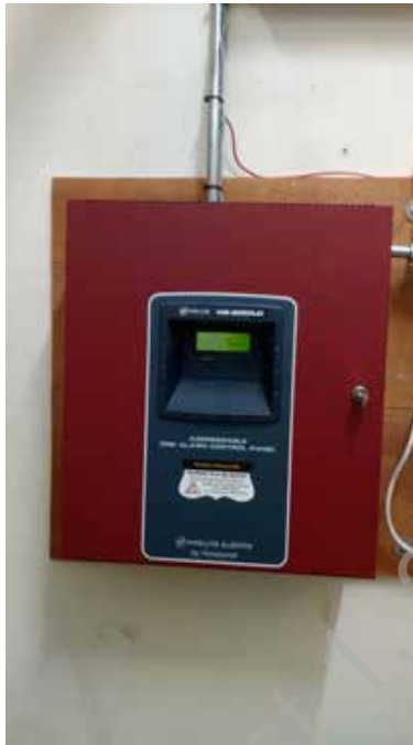
● D2. 13: Fire Alarm Control Panel
