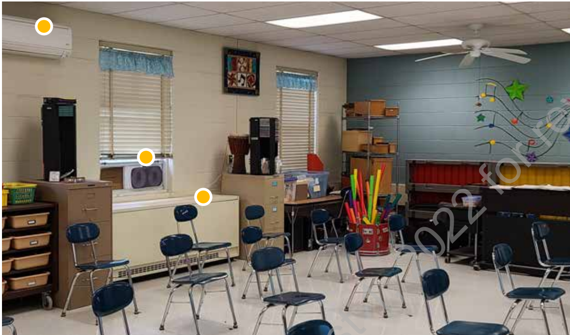
● D1. 41: View of music room with unit ventilator (center/left), window mounted fan for fresh air, and mini split unit (top left).
