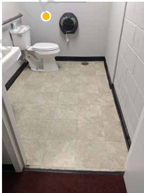
● D1. 28: Missing ADA grab bar at toilet rooms
