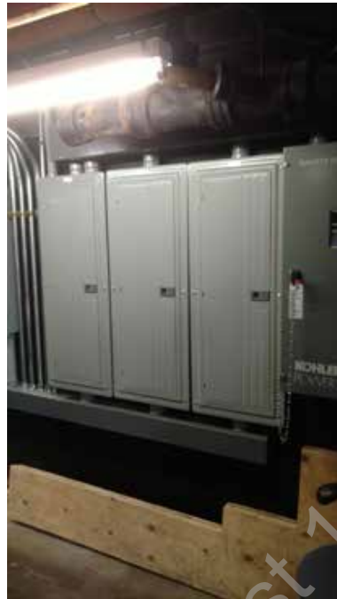
● D2. 5: Branch Circuit Panelboards
