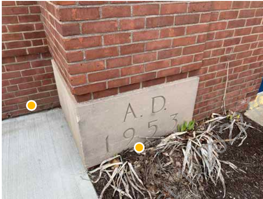
D1. 17: Monument stone at original building. Note deterioration at base of masonry wall.
