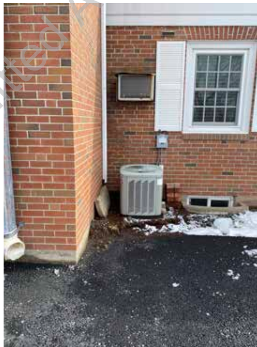
● D2. 8: Condensing Unit Serving FCU Provideing Cooling
