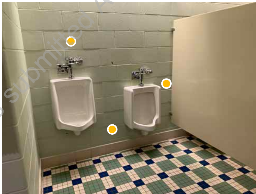
● D1. 36: View of typical boys/mens toilet room, note overall poor quality of construction and condition of CMU wet wall
