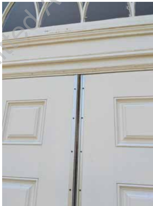
● D1. 24: Exterior doors at Lexture room appear to have received upgrades to weather seals
