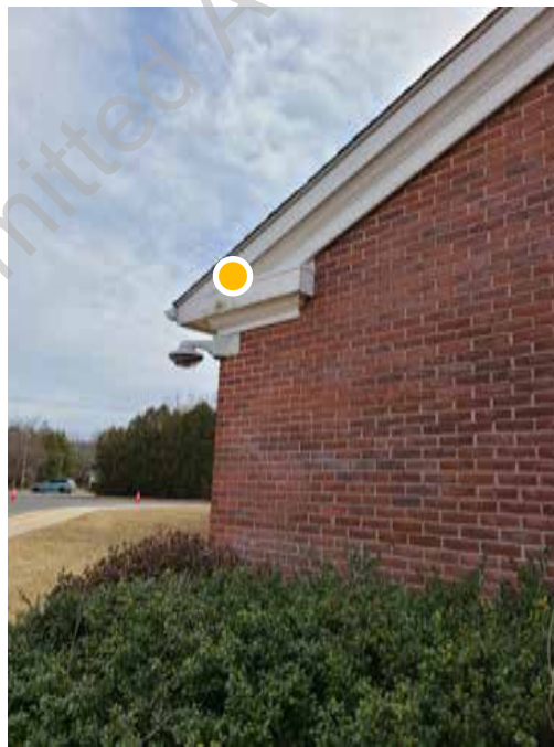
D1. 10: Detail view of trim detailing at 1988 addition along with spalling and deteriorated masonry composite wall.
