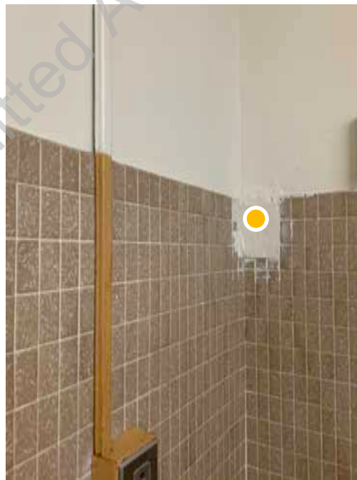
● D1. 64: Detail view of the wall tile repairs, various conditions throughout the bathroom spaces.
