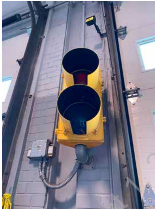
● D2. 25: Internal Traffic Control Light (Non-functional)
