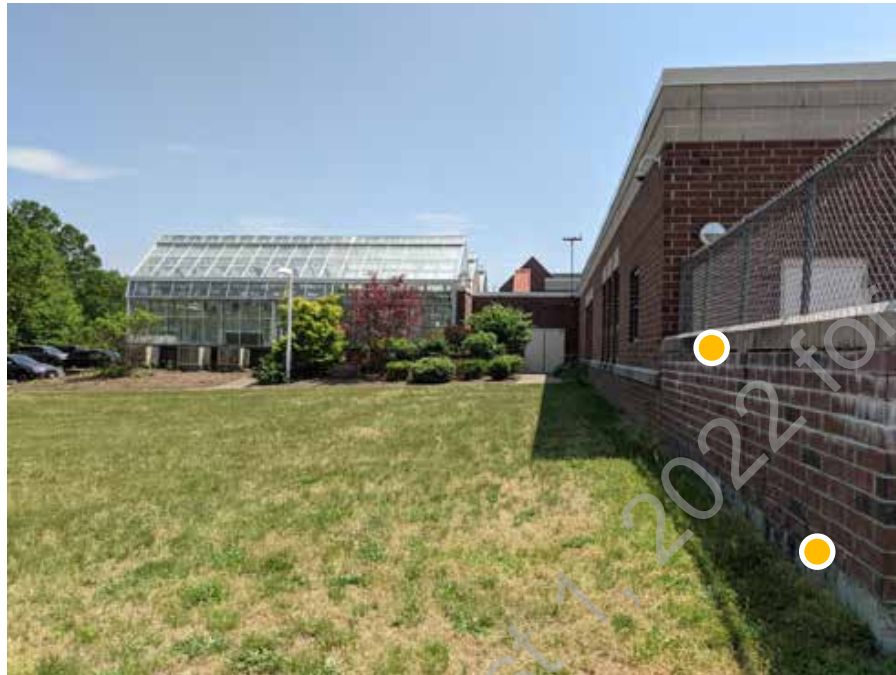
● D3. 17: View of east side of building with greenhouse structure in background. Masonry screen wall to right, note deterioration of masonry joints and efflorescence
