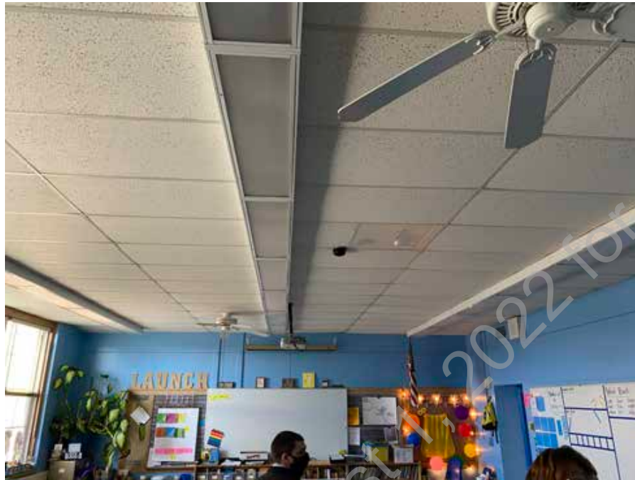
● D2. 37: View of typical classroom ceiling with inefficient fluorescent lighting surface mounted to ceiling.
