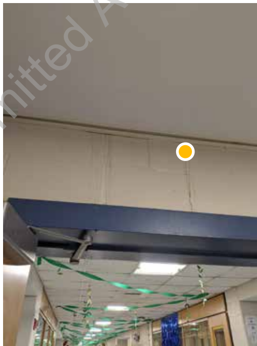
● D1. 90: Detail view of head condition at corridor doors, note visual signs of moisture/leaking.
