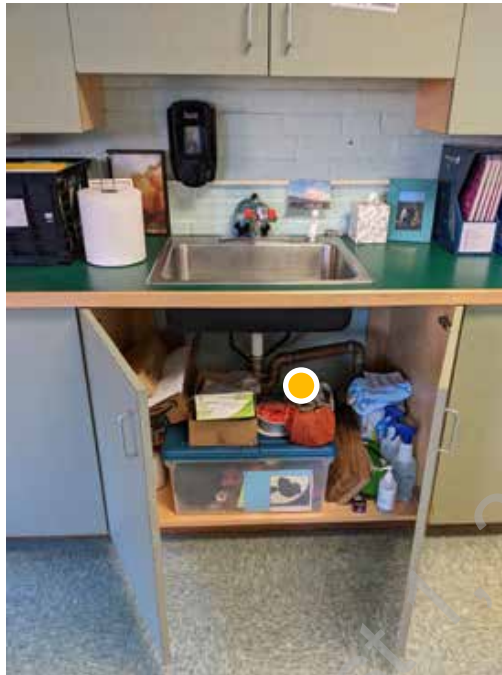
D1. 21: Detail view of inaccessible sink unit in the art room
