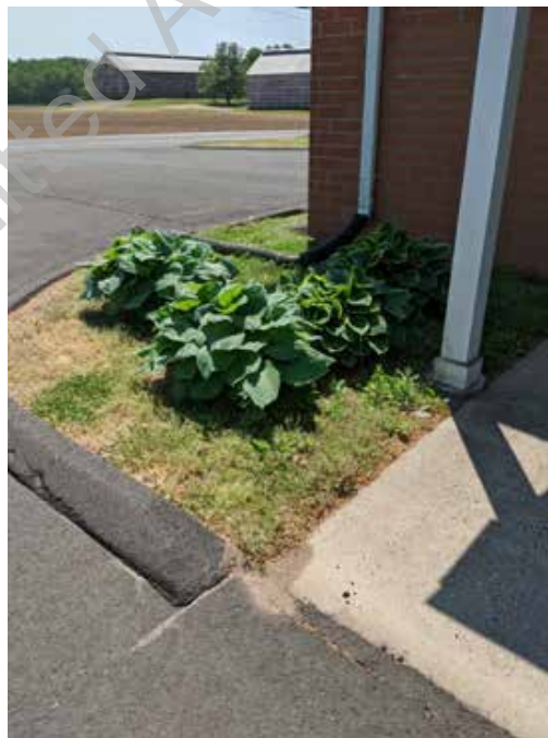
● D3. 4: Downspout requires permanent solution to assist in directional shedding of roof drainage
