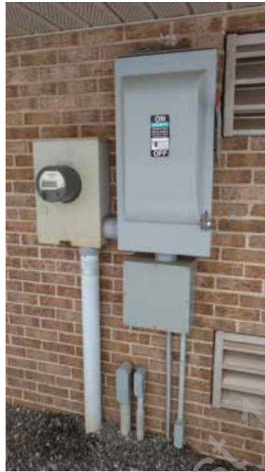
● D2. 5: Electrical Main Switch and Meter
