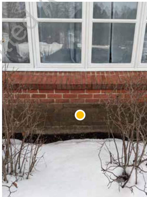
● D1. 12: Lack of gutter system above is causing soil erosion below and splashback onto brick façade
