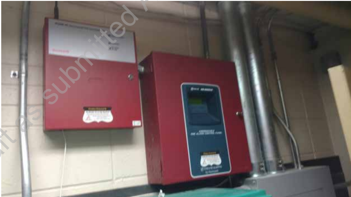
● D2. 8: Fire Alarm Panel and Communicator
