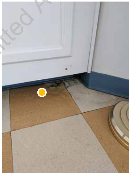
● D1. 32: Radiator leak has caused damage to vinyl tile floors
