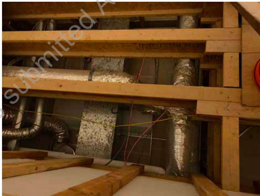
● D2. 16: Furnace Ductwork Routing through Attic Space
