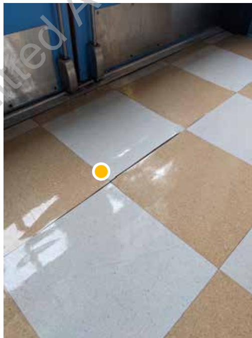
● D1. 36: Damaged vinyl tile flooring at entry doors into Dining
