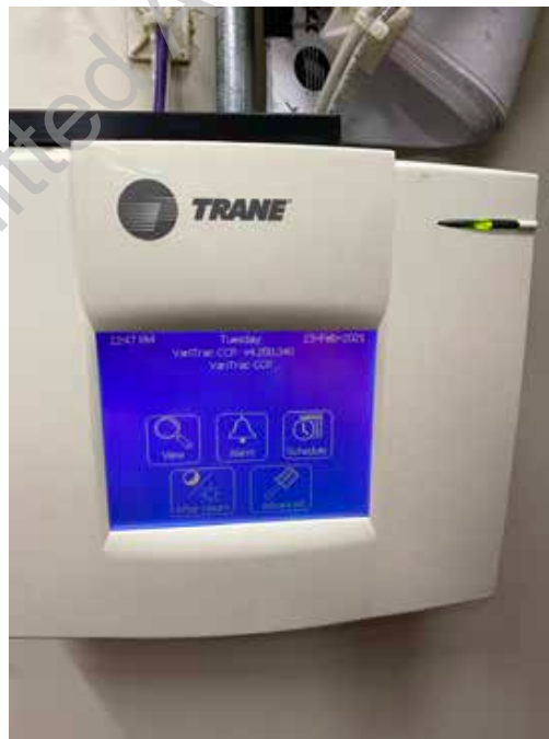
● D2. 32: Trane VariTrac CCP Temperature Control
