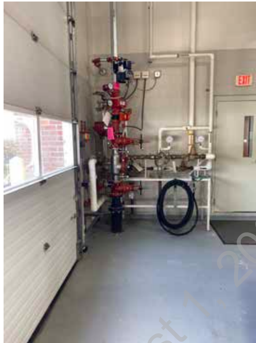
● D2. 15: Full Fire Protection Service Located in App Bay
