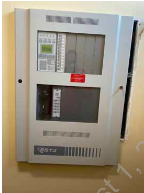
● D2. 17: Fire Alarm Control Panel (Remote)
