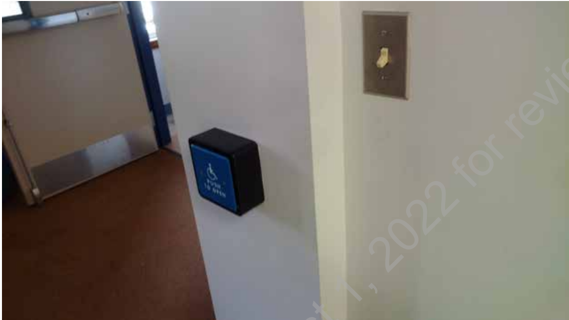
● D2. 41: Powered Door Control
