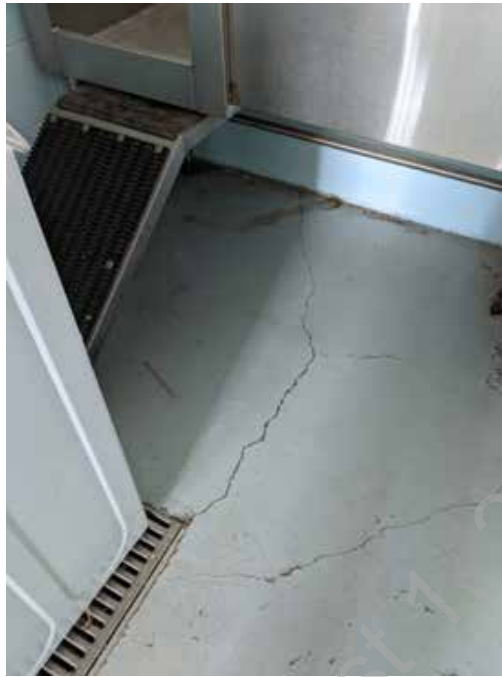
● D1. 97: Detail view of flooring and trench drain at animal science suite
