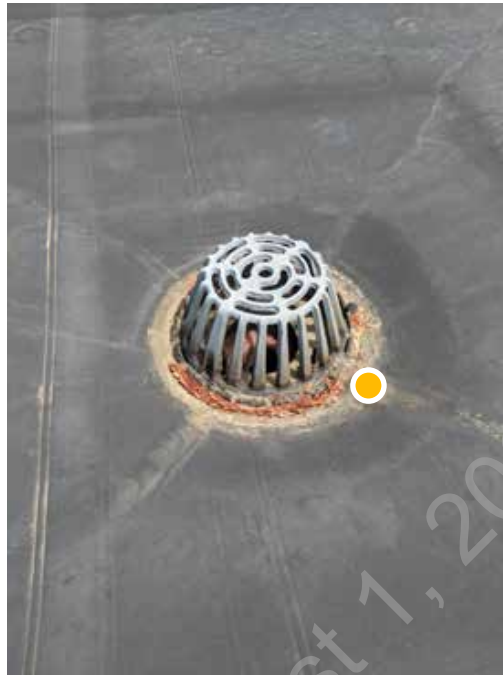
● D1. 3: Detail view of typical roof drain
