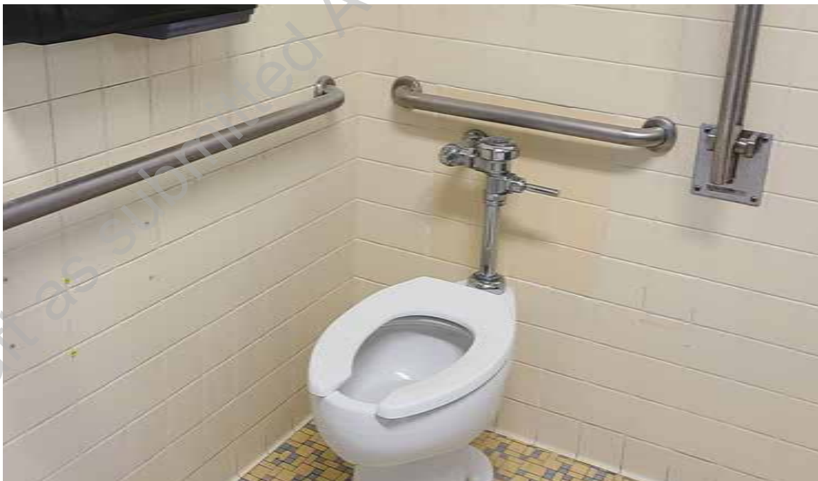
● D1. 32: Modified toilet stall to accommodate ADA requirements.
