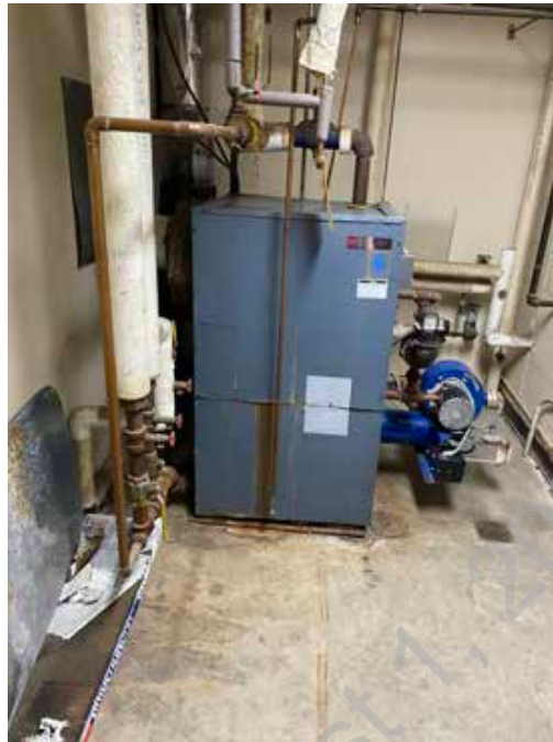
● D2. 15: Natural Gas Boiler
