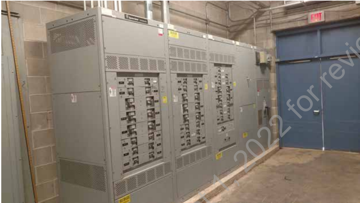
● D2. 7: Electrical Main Service Switchboard
