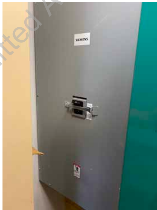
● D2. 14: Electrical Main Service Switch (1)
