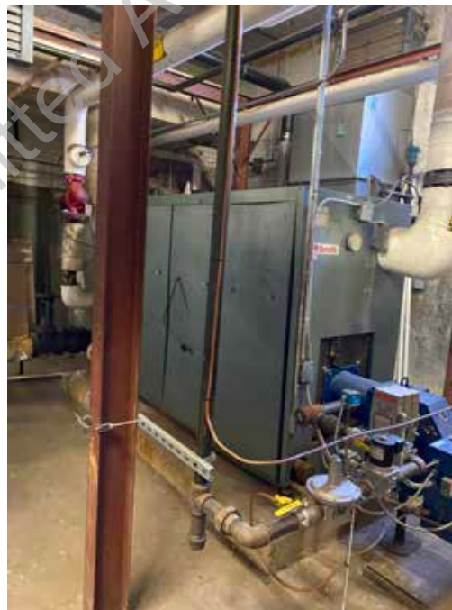
● D2. 14: H.B. Smith Natural Gas Boiler in Poor Working Condition.
