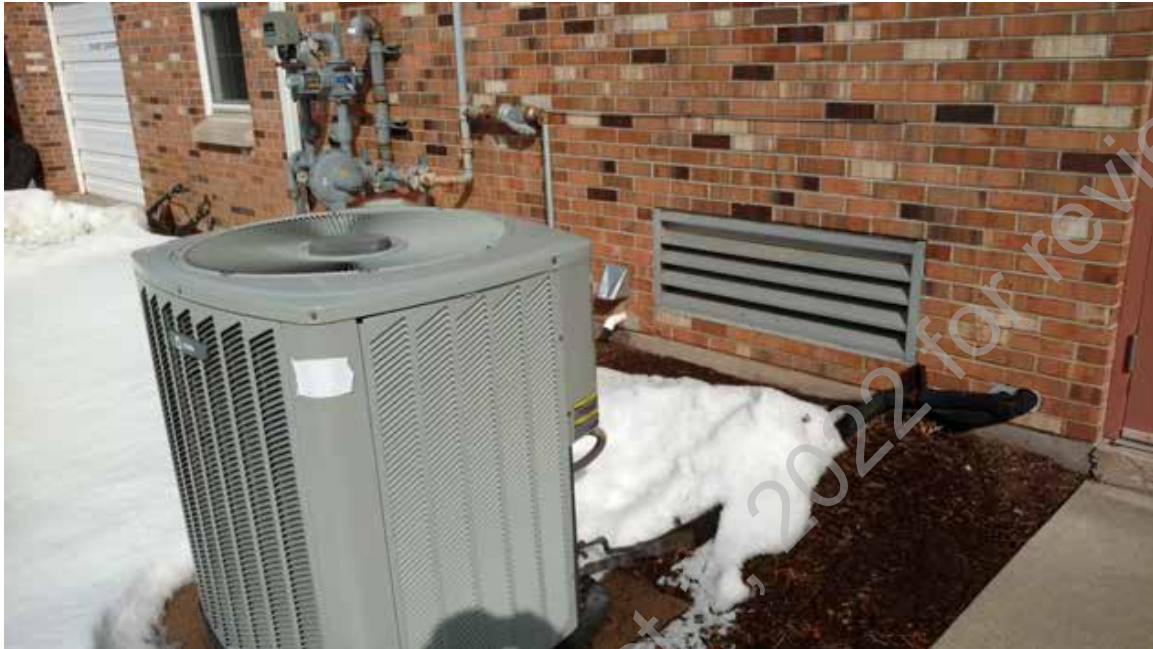
● D2. 33: Trane Condensing Unit Serves Indoor Air Handler
