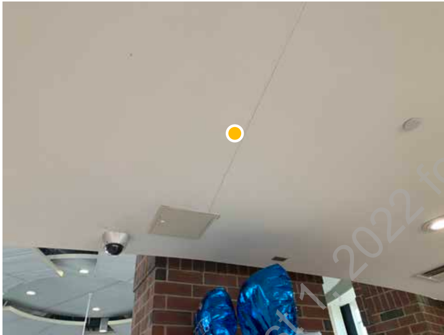
D1. 25: View of gypsum board ceiling around perimeter of cafeteria, note shrinkage cracking throughout ceiling.
