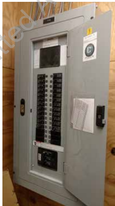
● D2. 12: Electrical Branch Circuit Panel
