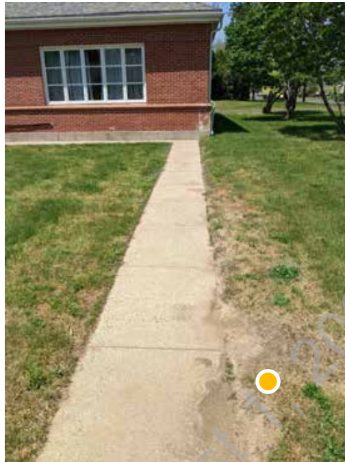
● D3. 11: Soil has eroded onto concrete sidewalks
