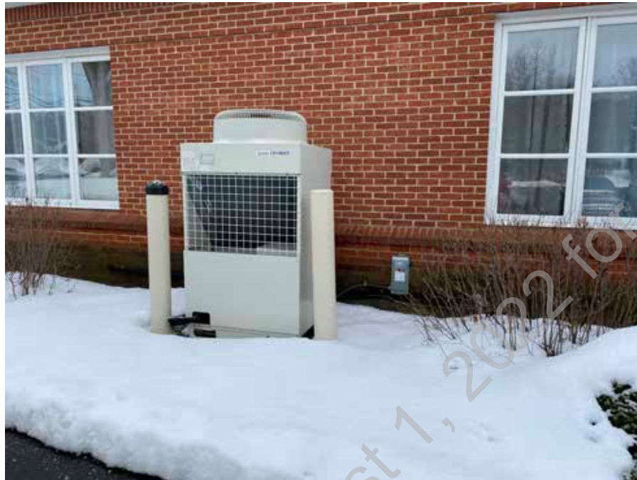
● D2. 37: Outdoor Condensing Unit
