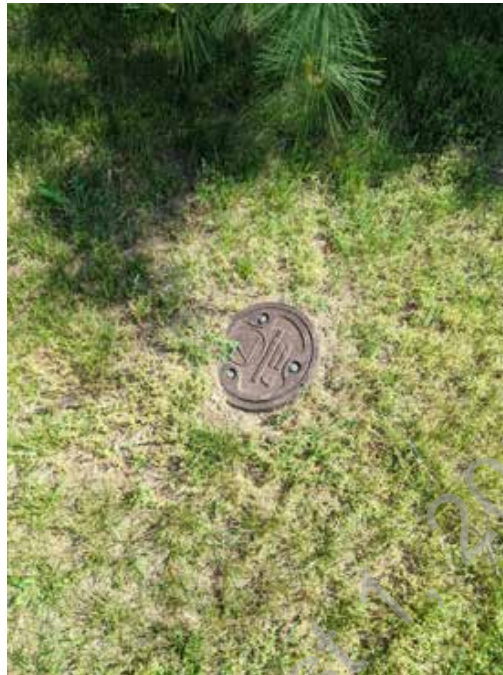
● D3. 7: Cleanout is partially buried
