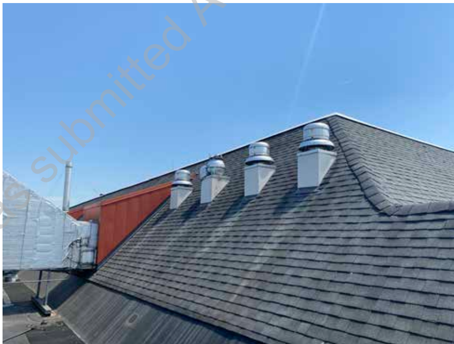
● D2. 10: Exhaust Fans on Roof in Good Condition
