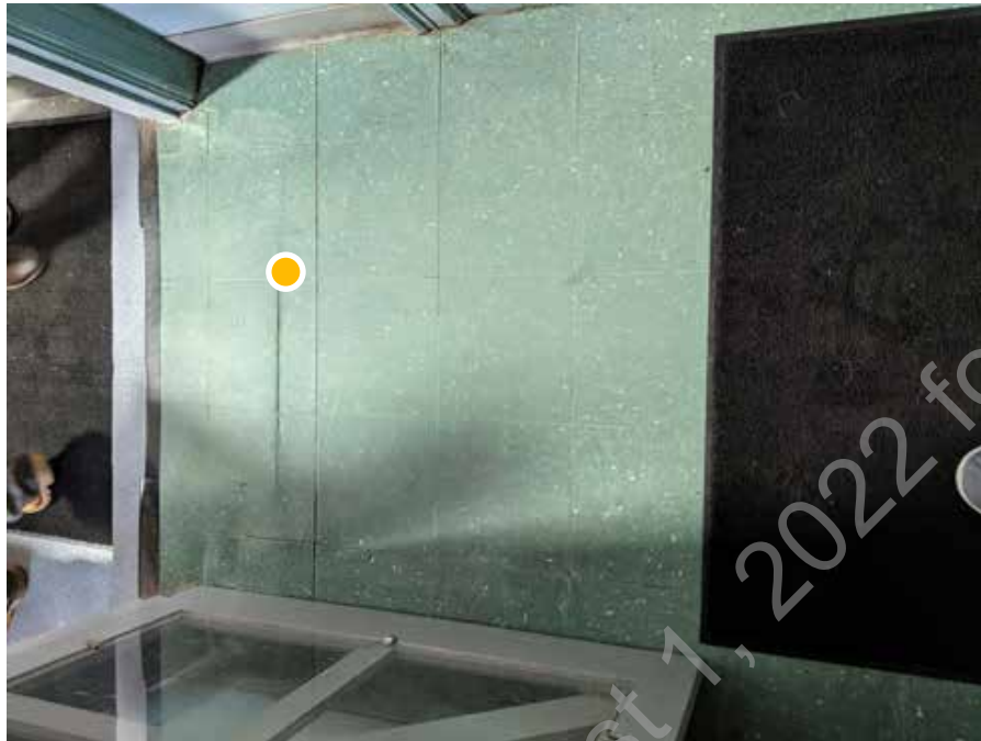
● D1. 17: Vinyl asbestos tile is present throughout, some cracking is beginning to show
