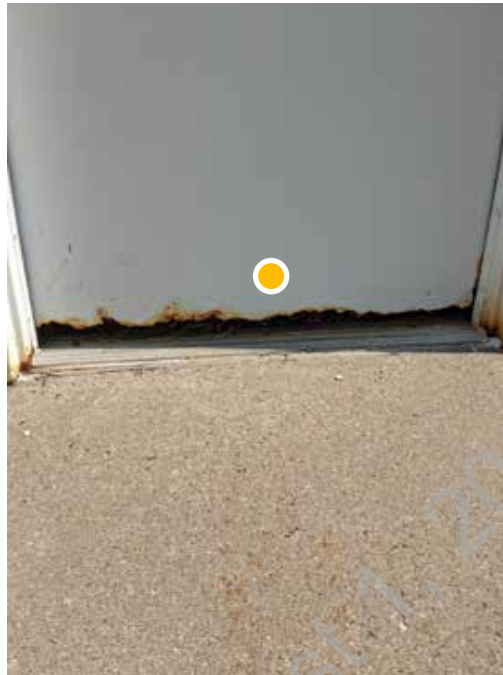
● D1. 19: Corrosion at base of storage room exterior door
