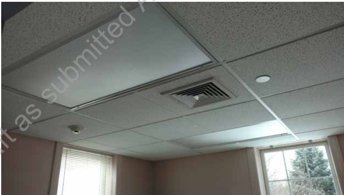
● D2. 4: Diffuser Being Served by the Furnace
