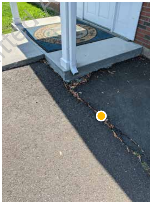
● D3. 8: Bituminous pavement cracking at main entry
