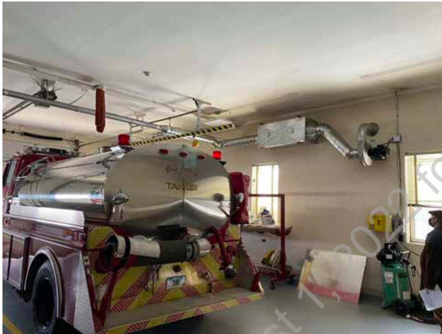
● D2. 23: Plymovent Exhaust System in App Bay
