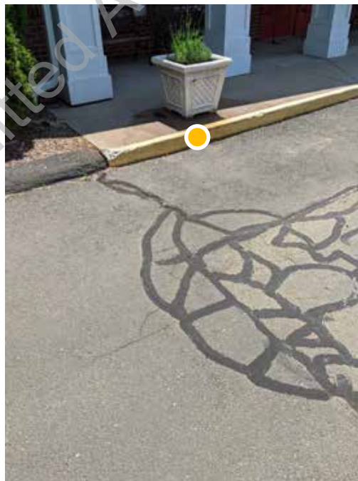
● D3. 16: Spalling concrete curb at main entry sidewalk
