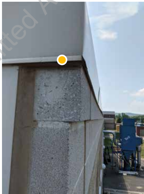
● D1. 8: Detail view of metal roof fascia at block wall, note the gap between face of wall and flashing, allows for pests and weather to penetrate the exterior envelope
