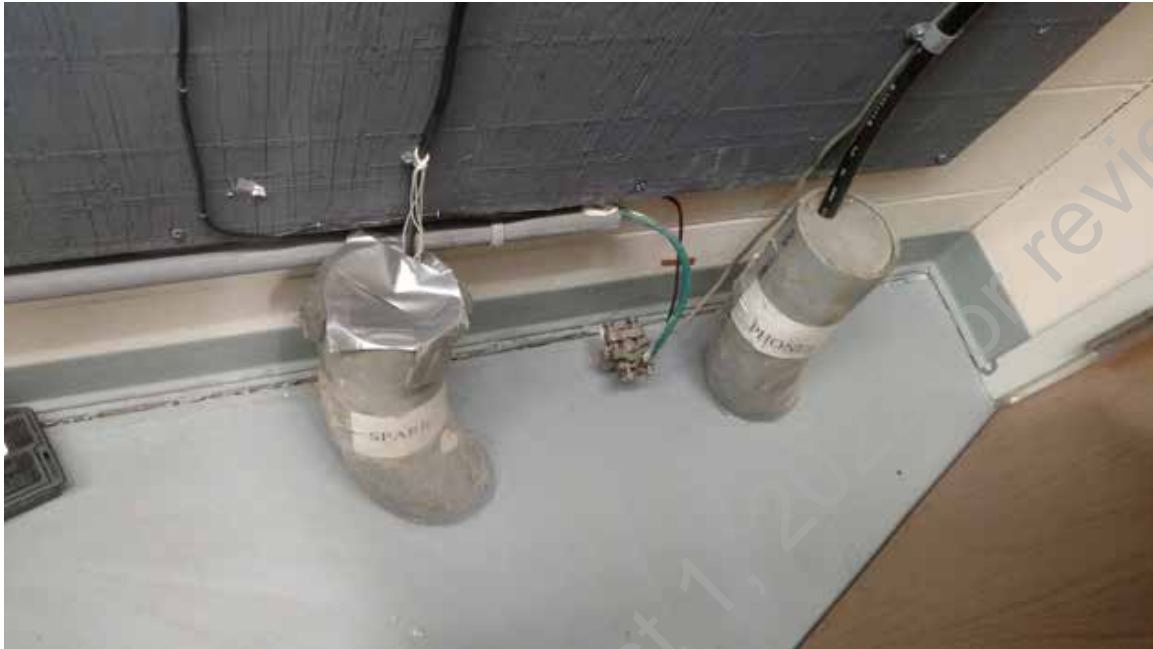
● D2. 3: Communication Service Conduits
