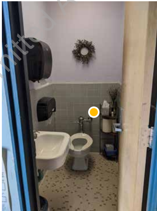
D1. 62: View of single use toilet room, does not comply with current accessibility codes( no grab bars, floor clearances, sink/reach, etc.).
