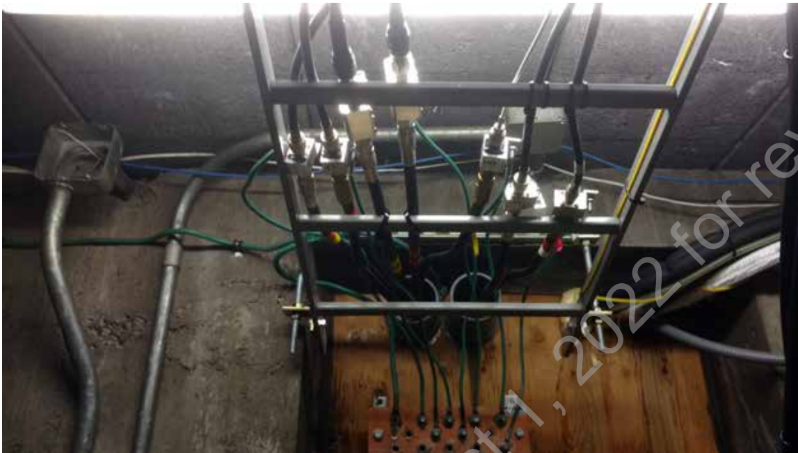
● D2. 1: Antenna Cables with Bonding
