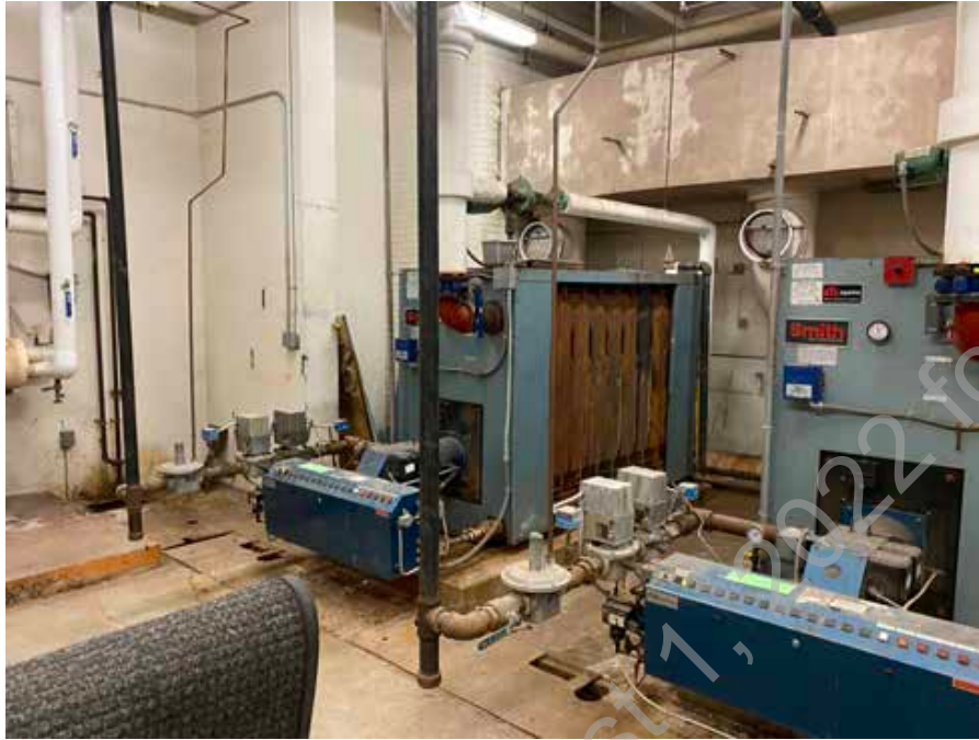
● D2. 33: Smith Natural Gas Cast Iron Hot Water Boilers in poor condition.
