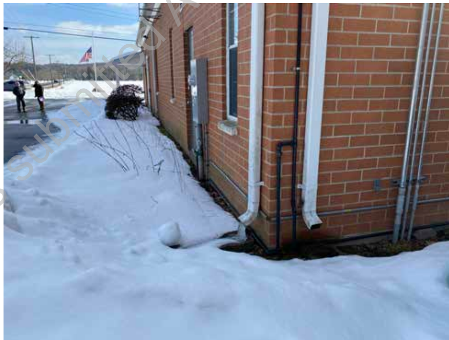
● D2. 14: Gutter Roof Drain Storm Service
