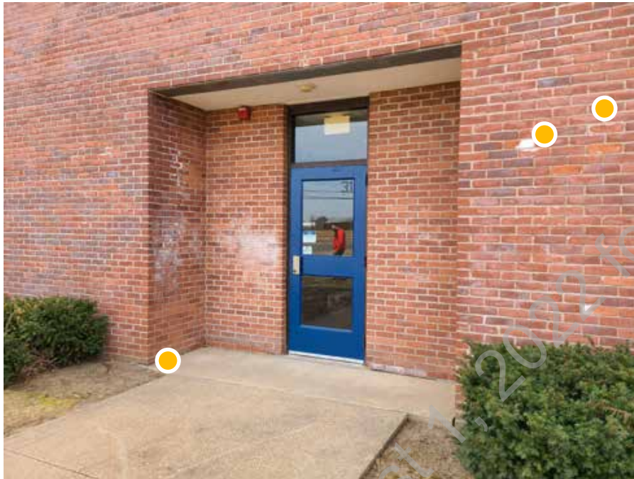
D1. 9: Detail view of entrance into 1988 classroom addition. Note masonry spalling and efflorescence due to moisture infiltration into composite wall construction.
