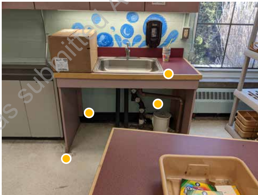
D1. 22: Detail view of inaccessible art room sink. Note the age and poor condition of the millwork and adjacent flooring.
