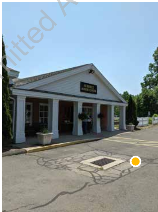
● D3. 2: Cracking throughout parking area and drive aisles has been patched
