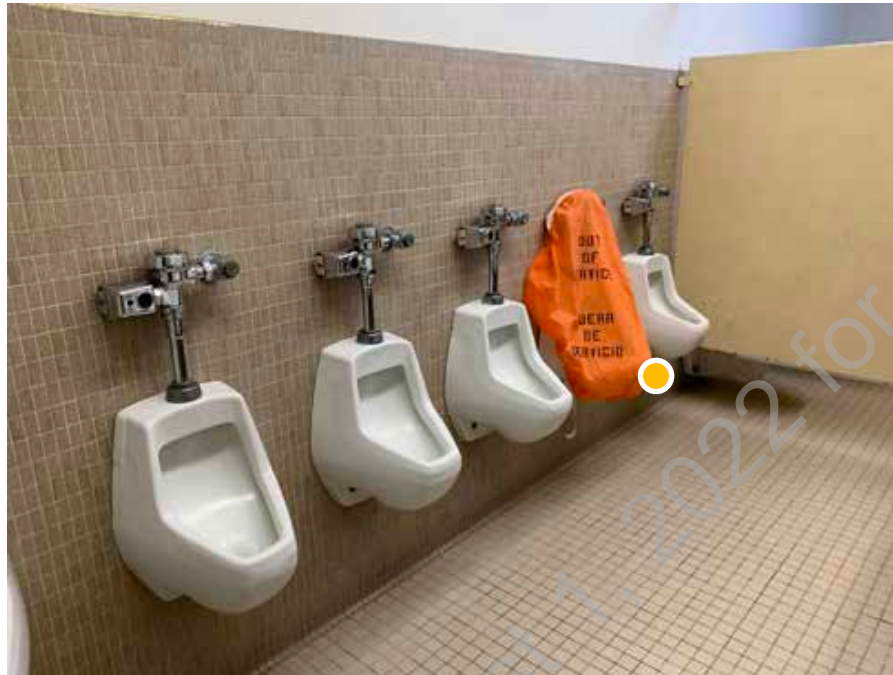
● D1. 63: View of typical bathroom assembly with some non functioning fixtures.
