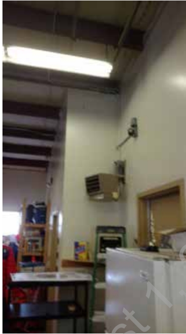
● D2. 7: Electric Unit Heater Serving Garage - Currently Inoperable
