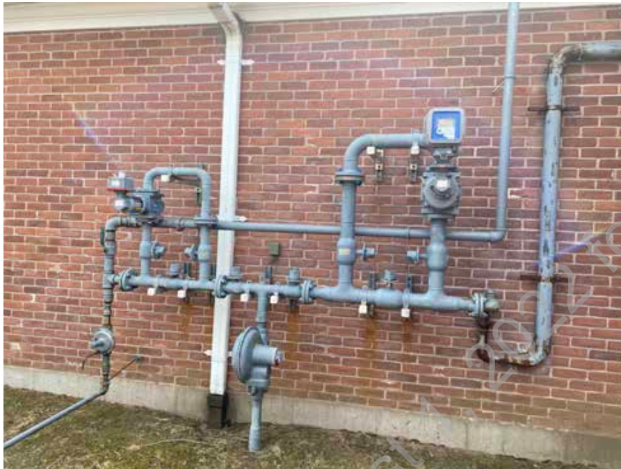
● D2. 25: Natural Gas Service in Good Condition.
