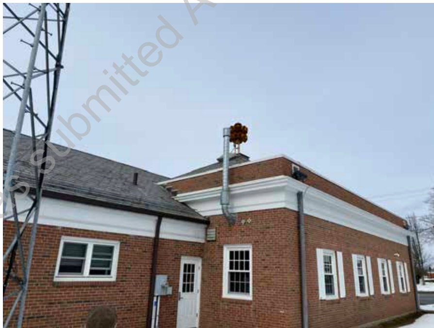
● D2. 6: Community Alert Siren Mounted on Roof
