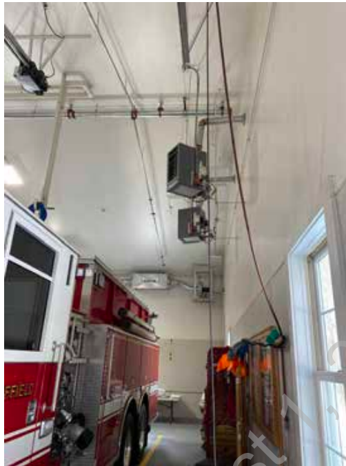
● D2. 25: Propane Fired Unit Heaters in App Bay
