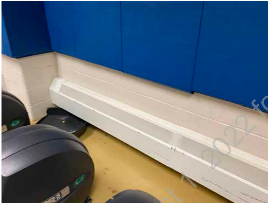
● D2. 57: Workout Room Fin Tube in Poor Condition
