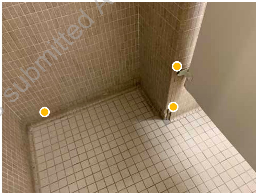
● D1. 36: Detail view of typical bathroom depicting missing and/or broken floor and wall tiles along with retrofit or painted toilet partitions.
