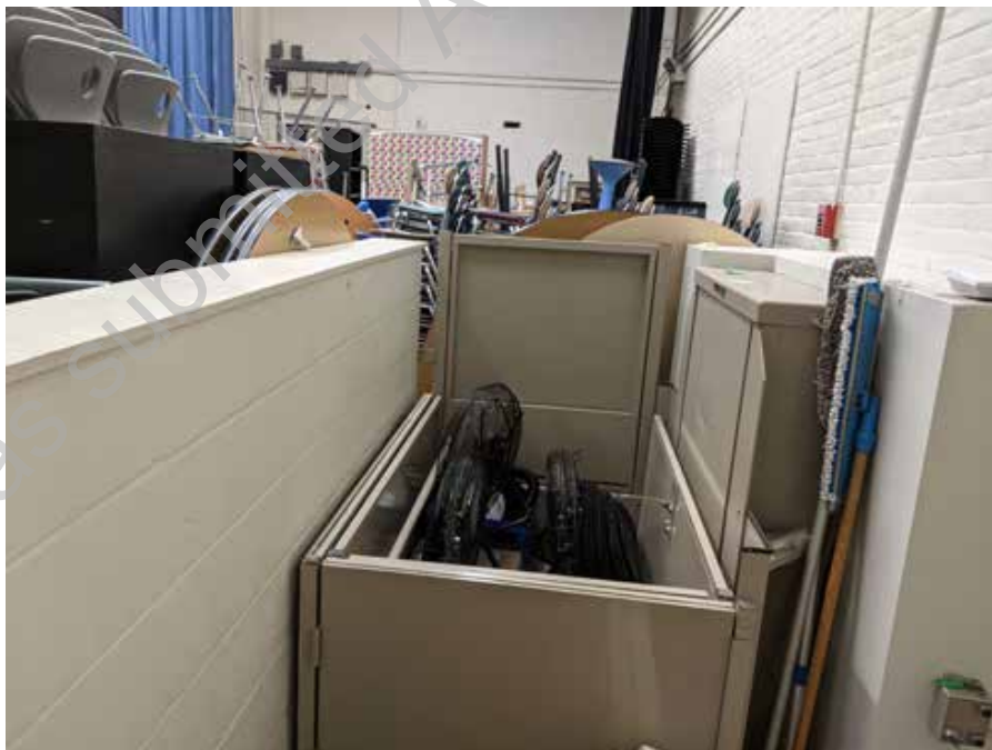
● D1. 30: View of accessibility lift to stage. Note, this equipment did not function at time of walkthrough, no ADA access is provided.
