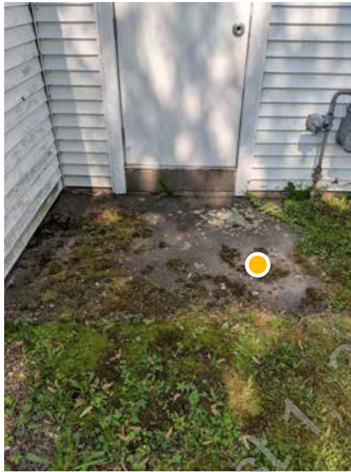
● D1. 21: Organic growth at concrete pad; Vinyl siding damaged at base
