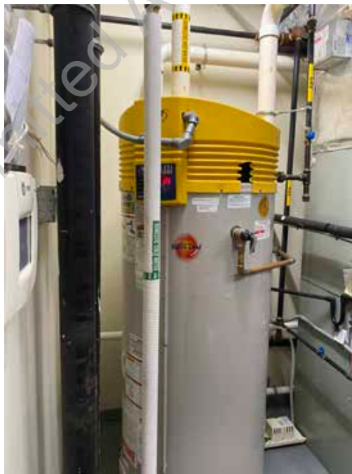
● D2. 26: Propane Fueled Domestic Hot Water Heater
