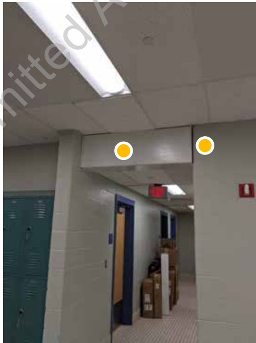
● D1. 82: Detail view of soffit repair in locker room areas, damaged due to use.
