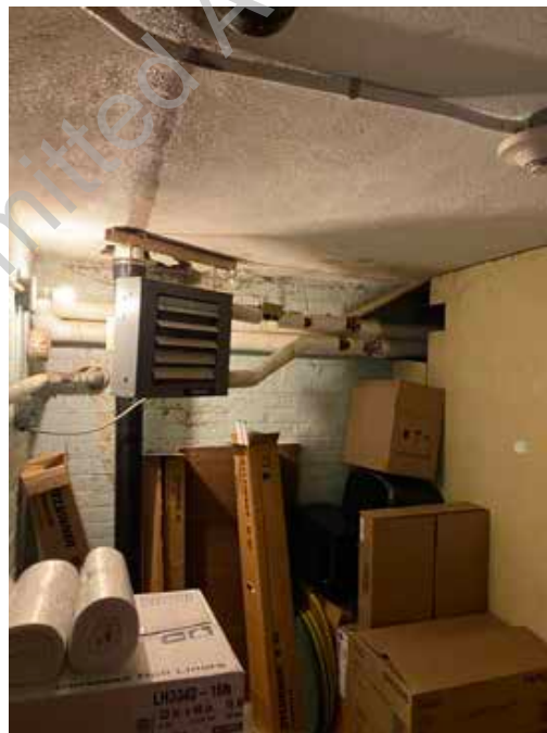
● D2. 20: Hot Water Unit Heater in Poor Condition.
