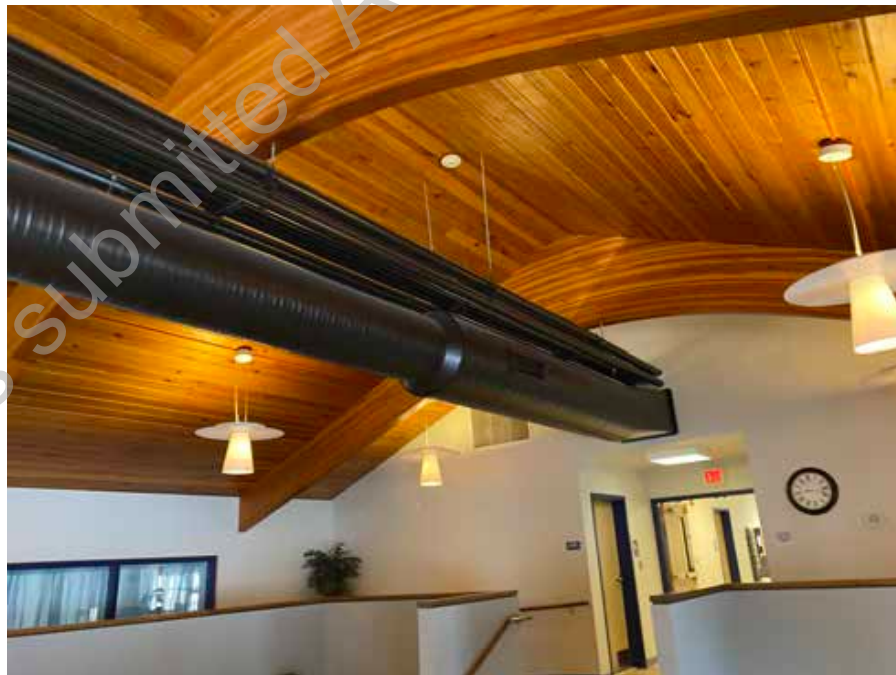
● D2. 6: Ductwork From Fan Coil Unit in Good Condition
