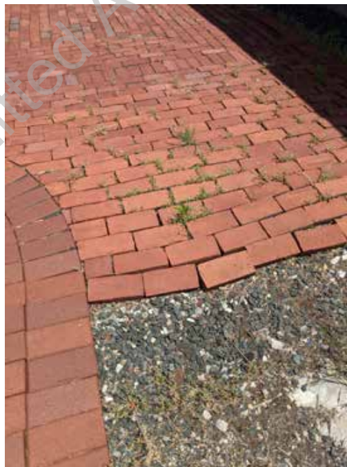
● D3. 8: Bricks at rear courtyard have begun to heave and create unsafe conditions
