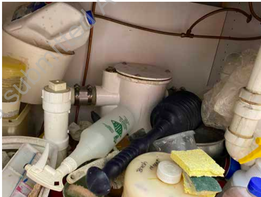
● D2. 44: Detail view of clay trap and PVC plumbing in fair to poor condition with indication of previous leaks via the staining
