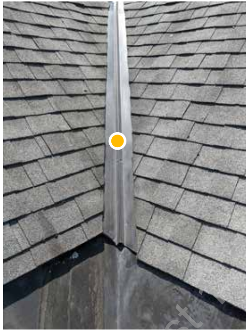
● D1. 5: Typical valley flashing at asphalt shingle roof in fair to good condition overall
