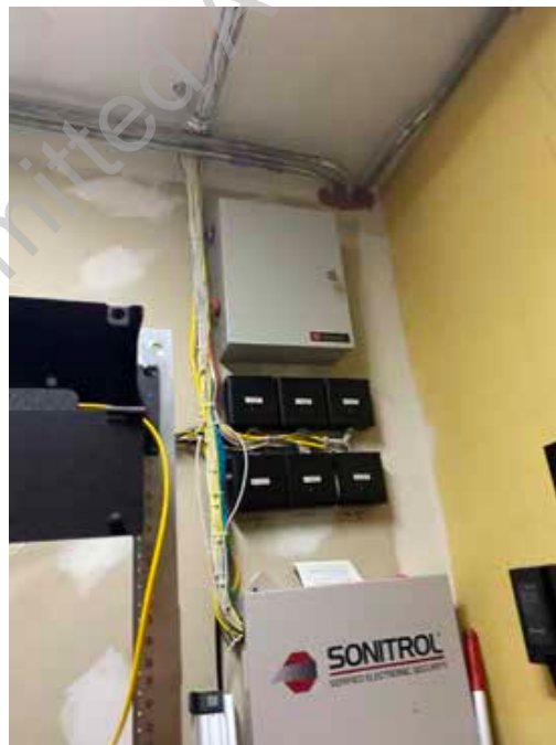
● D2. 2: Access Control System Head End.
