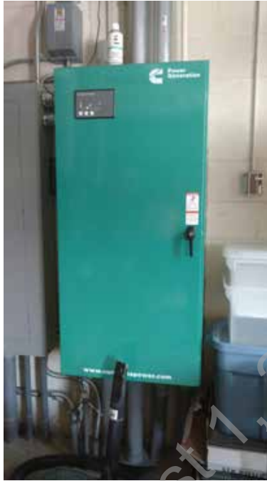
● D2. 1: Automatic Transfer Switch
