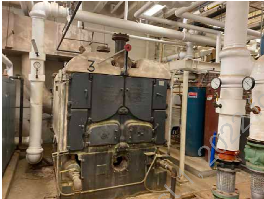
● D2. 1: Abandoned Old Cast Iron Boiler in Mechanical Room.
