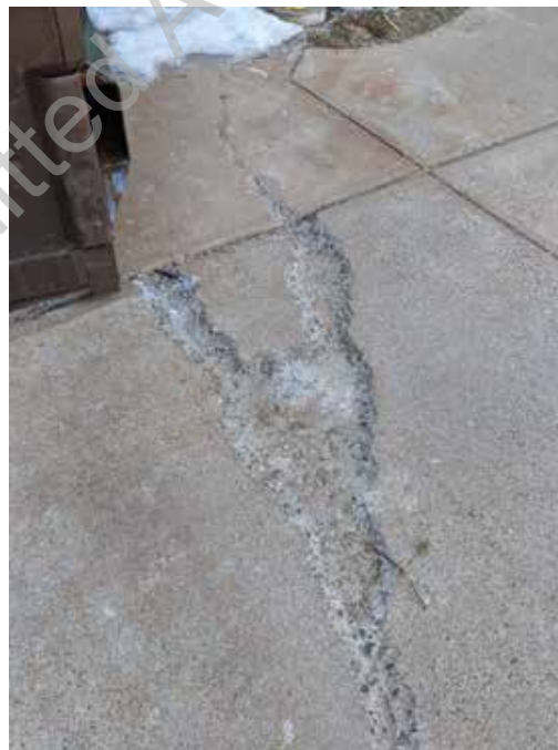
● D3. 6: Typical condition of concrete sidewalks adjacent to service area, note severe cracking likely caused by settlement and moisture infiltration.
