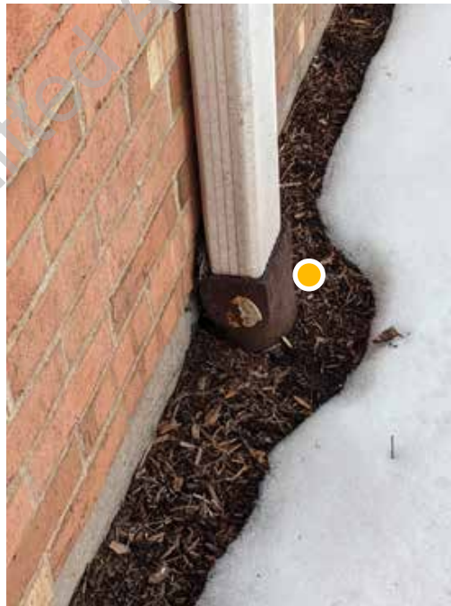
● D1. 4: Rusty boot connecting downspout to sub-surface drainage system
