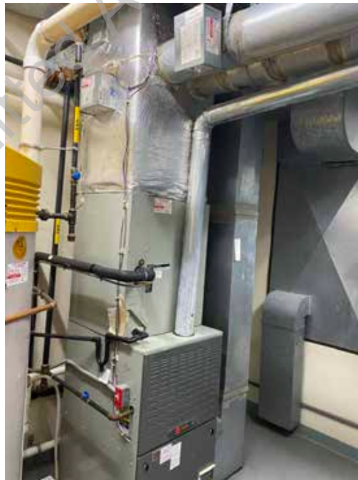
● D2. 24: Propane Fired Furnace and Connecting Ductwork
