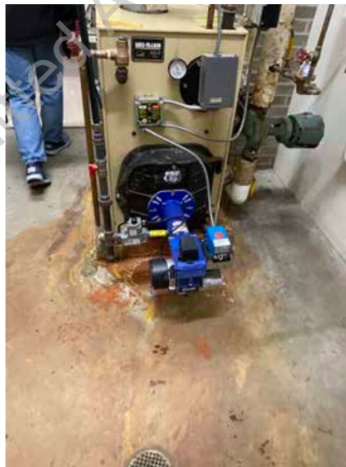
● D2. 30: Weil McLain Propane Fired Hot Water Boiler
