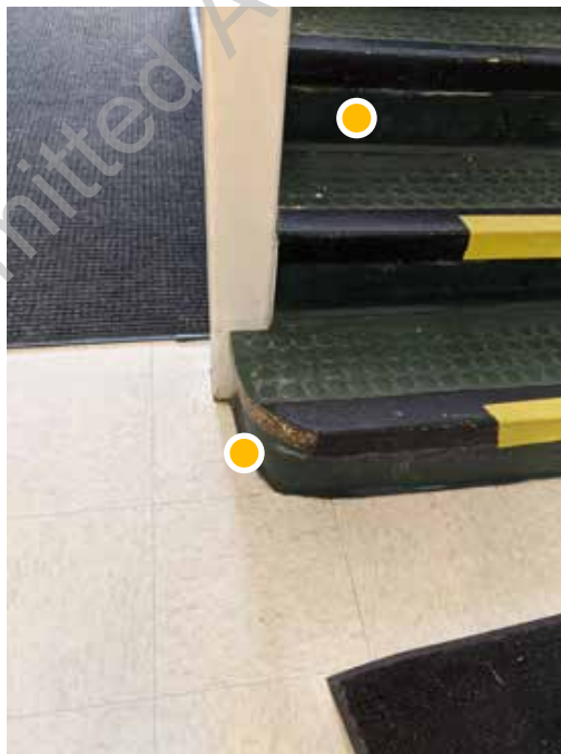
● D1. 58: Detail view of typical poor condition of the rubber treads and risers at the stairs.
