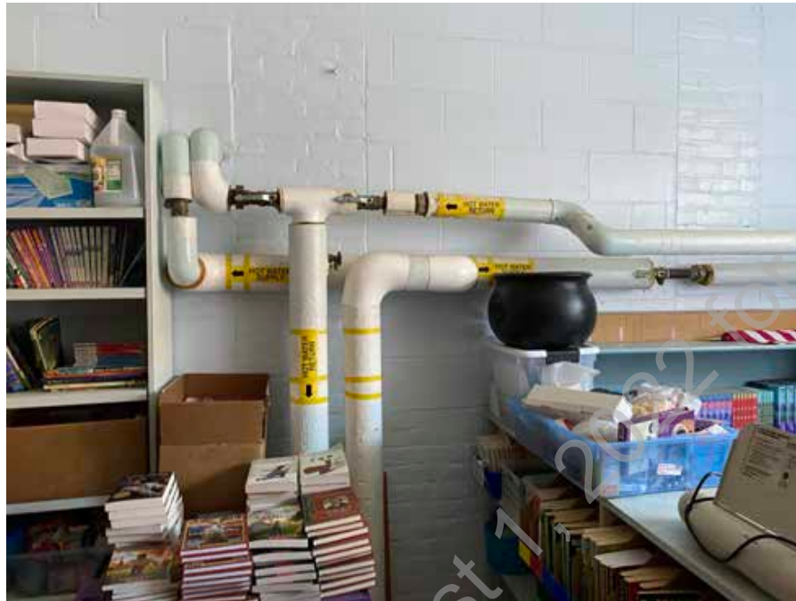
● D2. 21: Detail view of exposed piping retrofits within an existing educational space.
