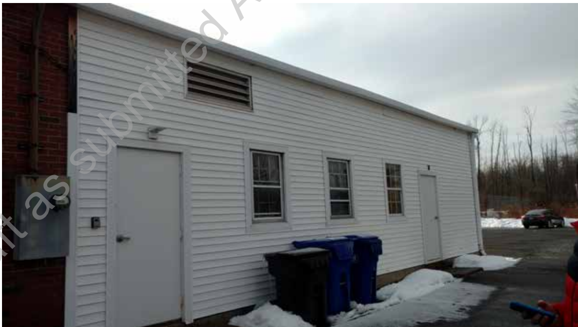
● D2. 32: Sidewall Exhaust Louver Serving Furnace
