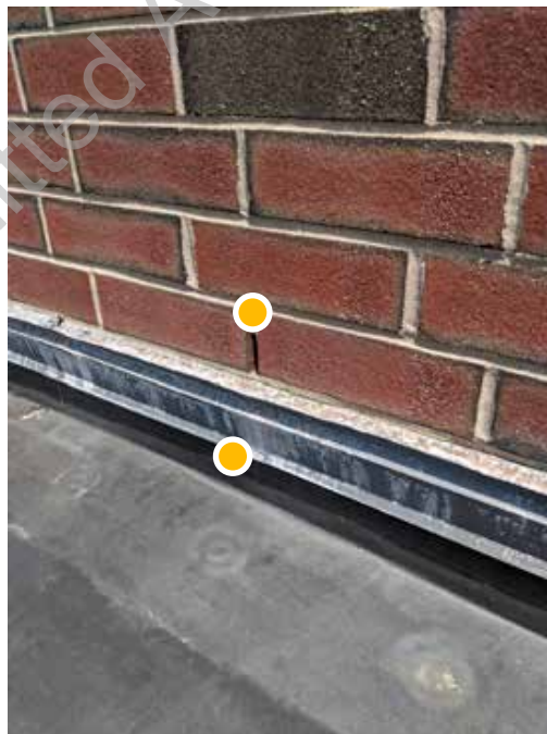
● D1. 4: Detail view of masonry wall weep holes and roof to wall counter flashing, in good condition overall
