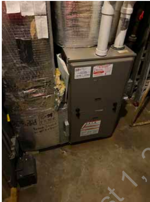
● D2. 25: Natural Gas Fired Furnace Located in Mechanical Room
