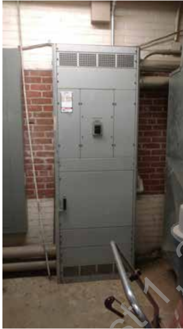
● D2. 11: Electric Service Main Switch.
