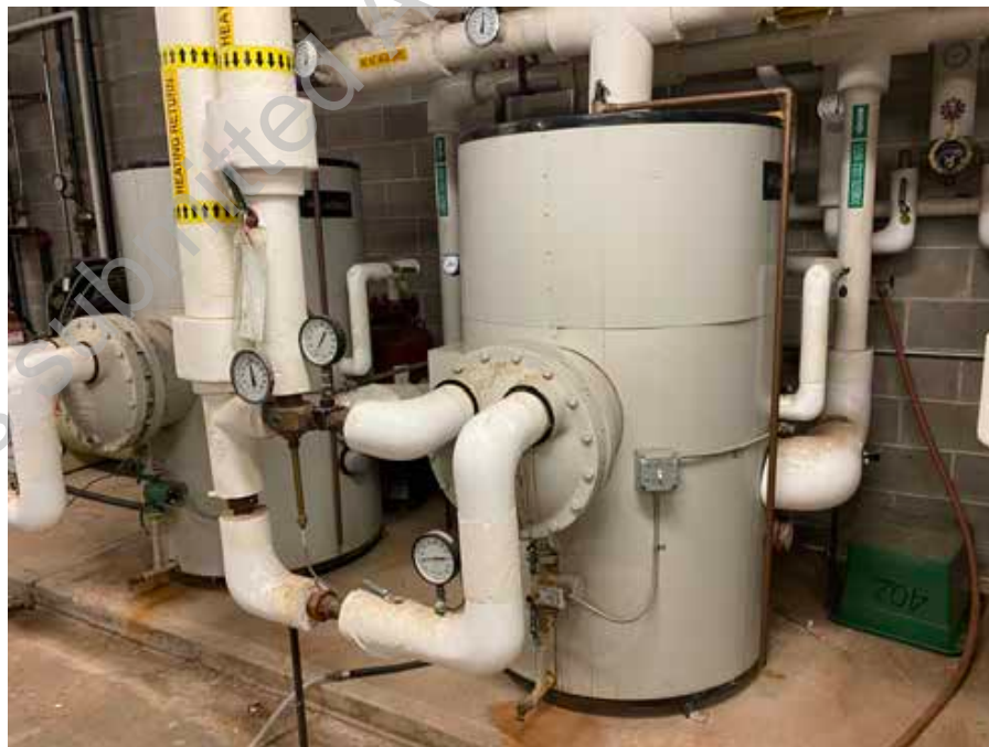
● D2. 36: Lochinvar Domestic Water Heaters in Mechanical Room
