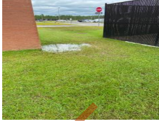
Area on southeast corner holding water
