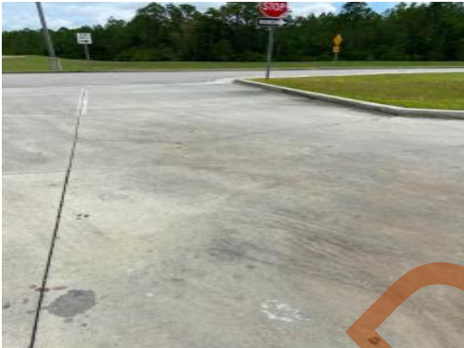
Concrete drive in southeast corner
