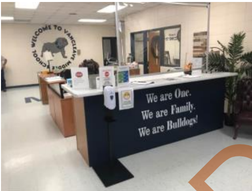
Office counter not ADA compliant
