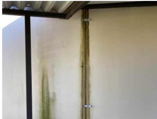
Missing downspout
