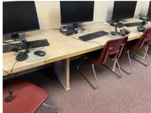
Peeling veneer in computer lab
