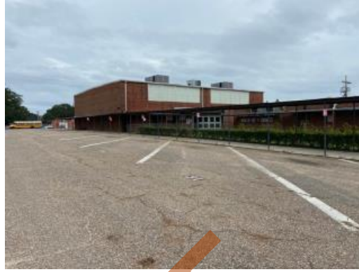
Asphalt and striping north of Bldg A
