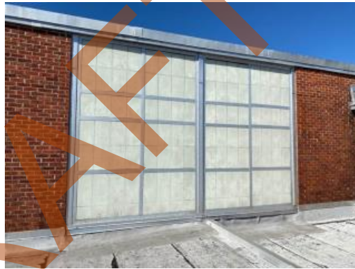
Original aluminum window system at gym
