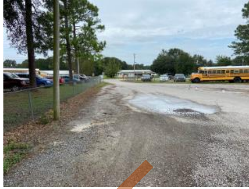
Failing asphalt
