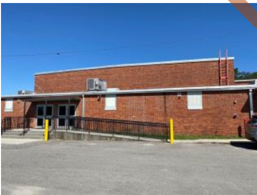
Overall building photo
