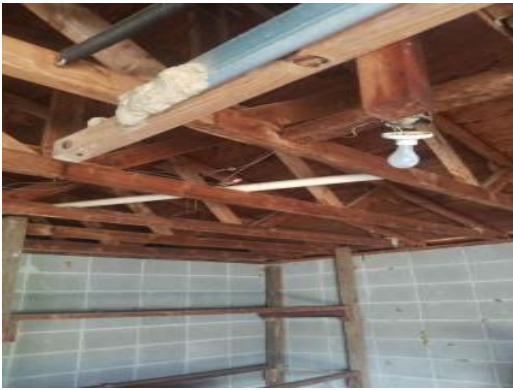
Exposed wiring
