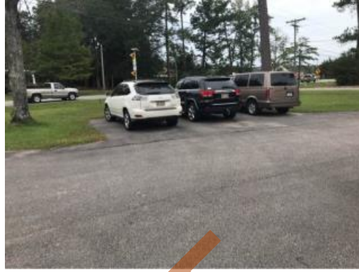
No ADA parking identified, no parking lot striping
