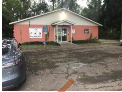
ADA signage and parking space Restripe
