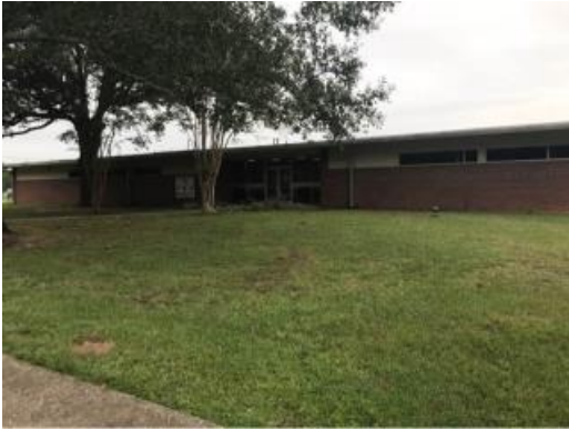
South Elevation Main Entrance
