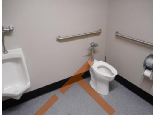
Fab Lab restroom fixtures and finishes
