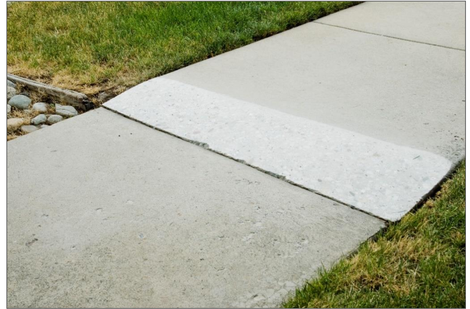
Using our Patented Saw-Cutting Technology the same panel is now compliant with Americans with Disability Act.
