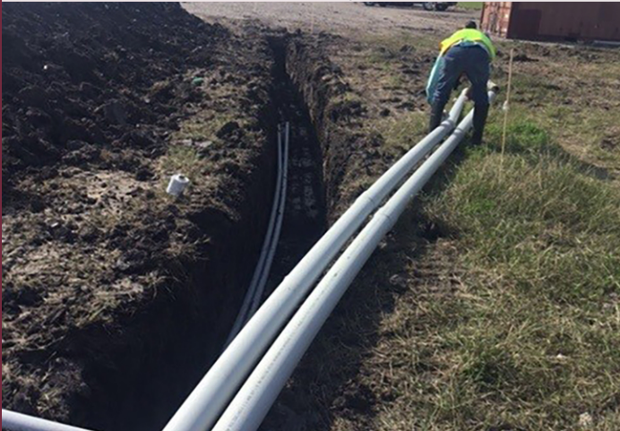
Photo 03 - Installation of data/power conduit along loop road
