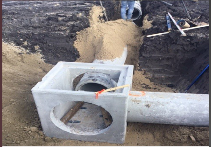
Photo 02 - Installation of new storm drainage piping
