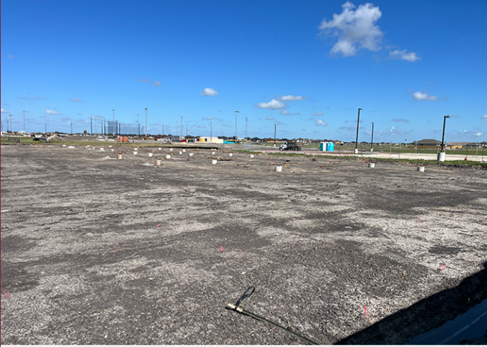
Photo 01 - Classroom wing addition foundation piers in place
