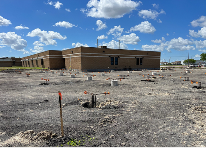
Photo 01 - Classroom wing addition foundation piers in place
