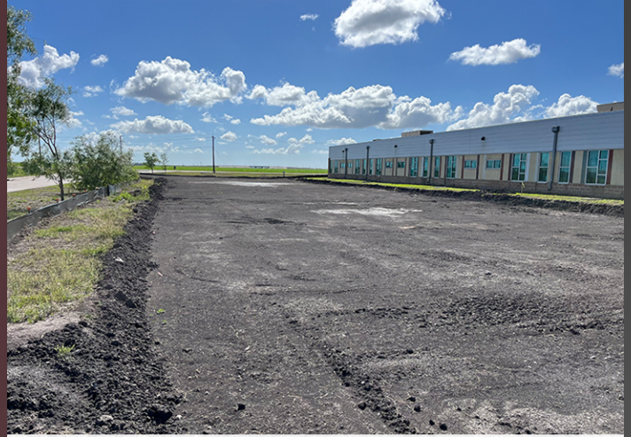
Photo 02 - Parking lot addition subgrade improvements complete
