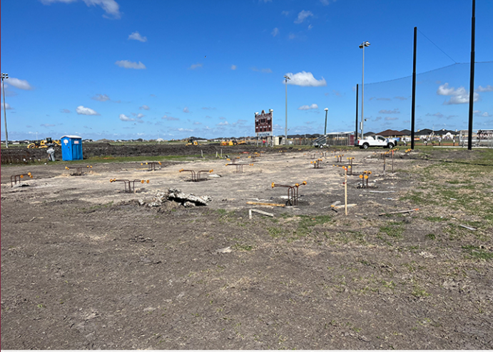
Photo 01 - View west at concessions, foundation piers complete
