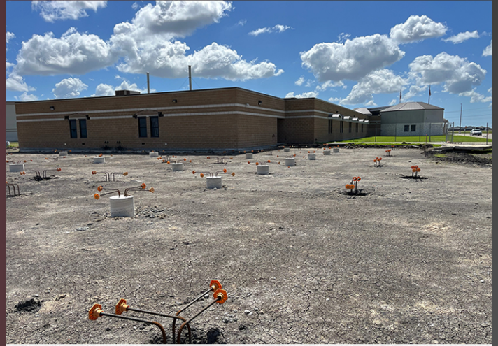
Photo 02 - Classroom wing addition foundation piers in place
