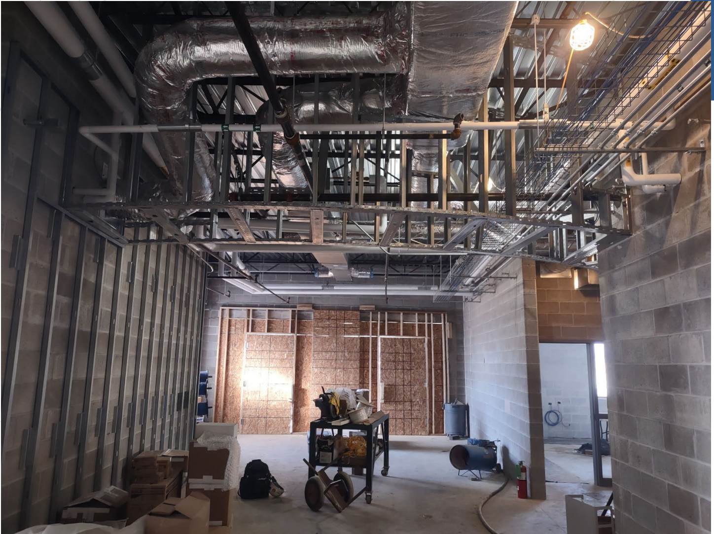
Classroom Addition Learning Commons with bulkhead framing installed. Temporary plywood enclosure will be replaced with aluminum storefront system.
