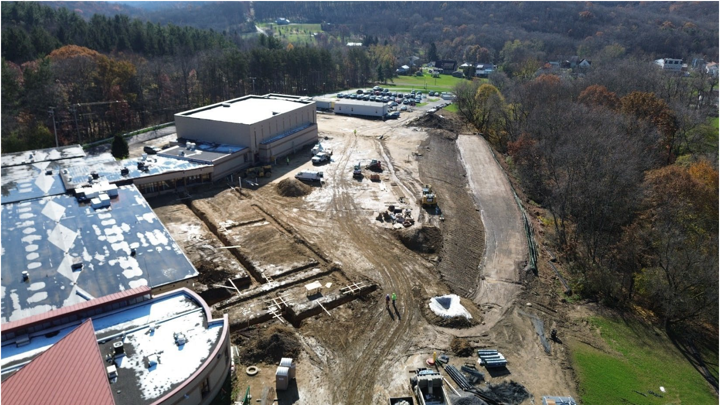
Foundations begun for classroom/administrative addition, Mechanically-Stabilized Earth Retaining Wall is underway on the right edge.
