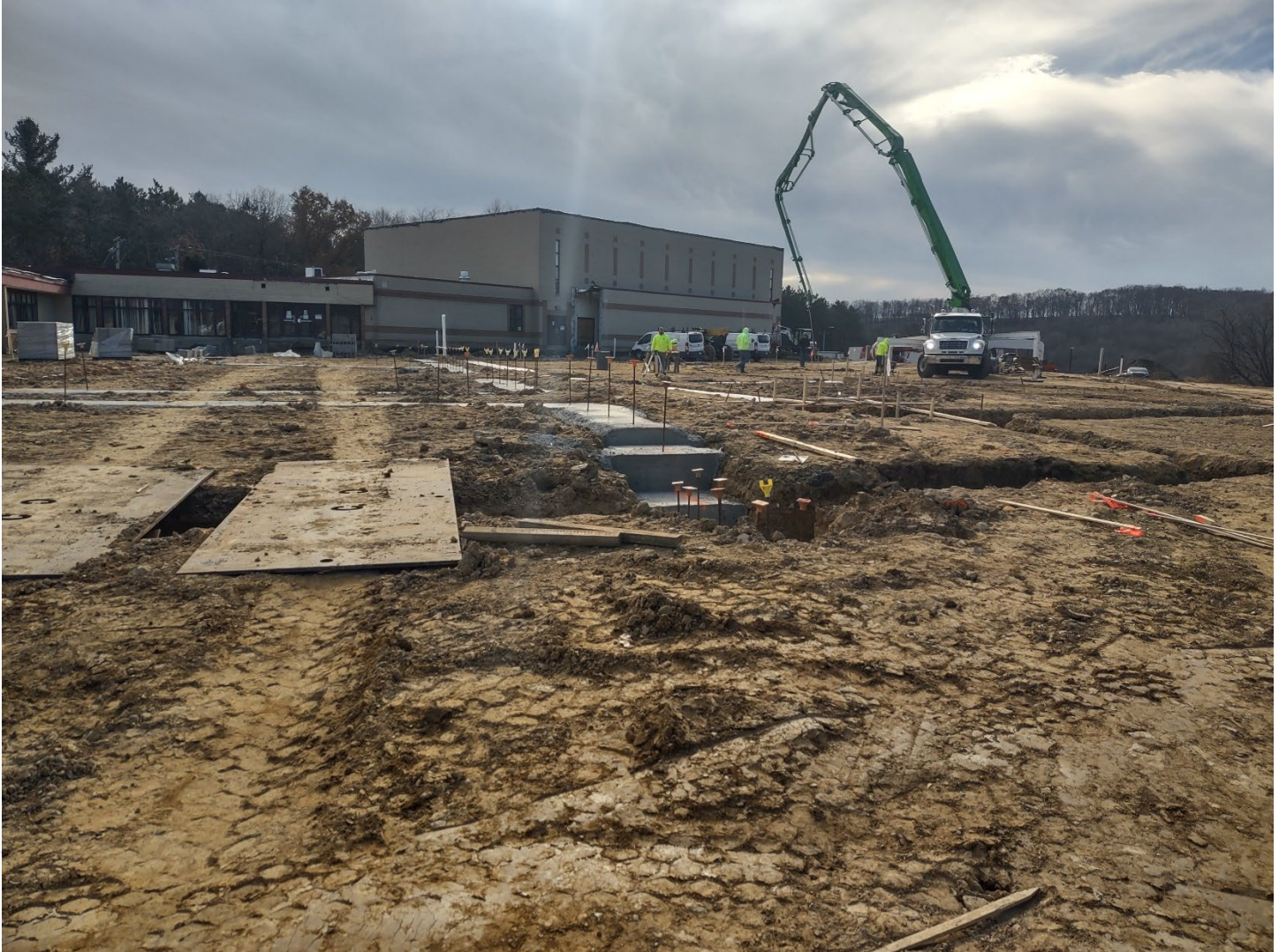
Area C Classroom Admin Area, and Entry Corridor foundation concrete being placed.
