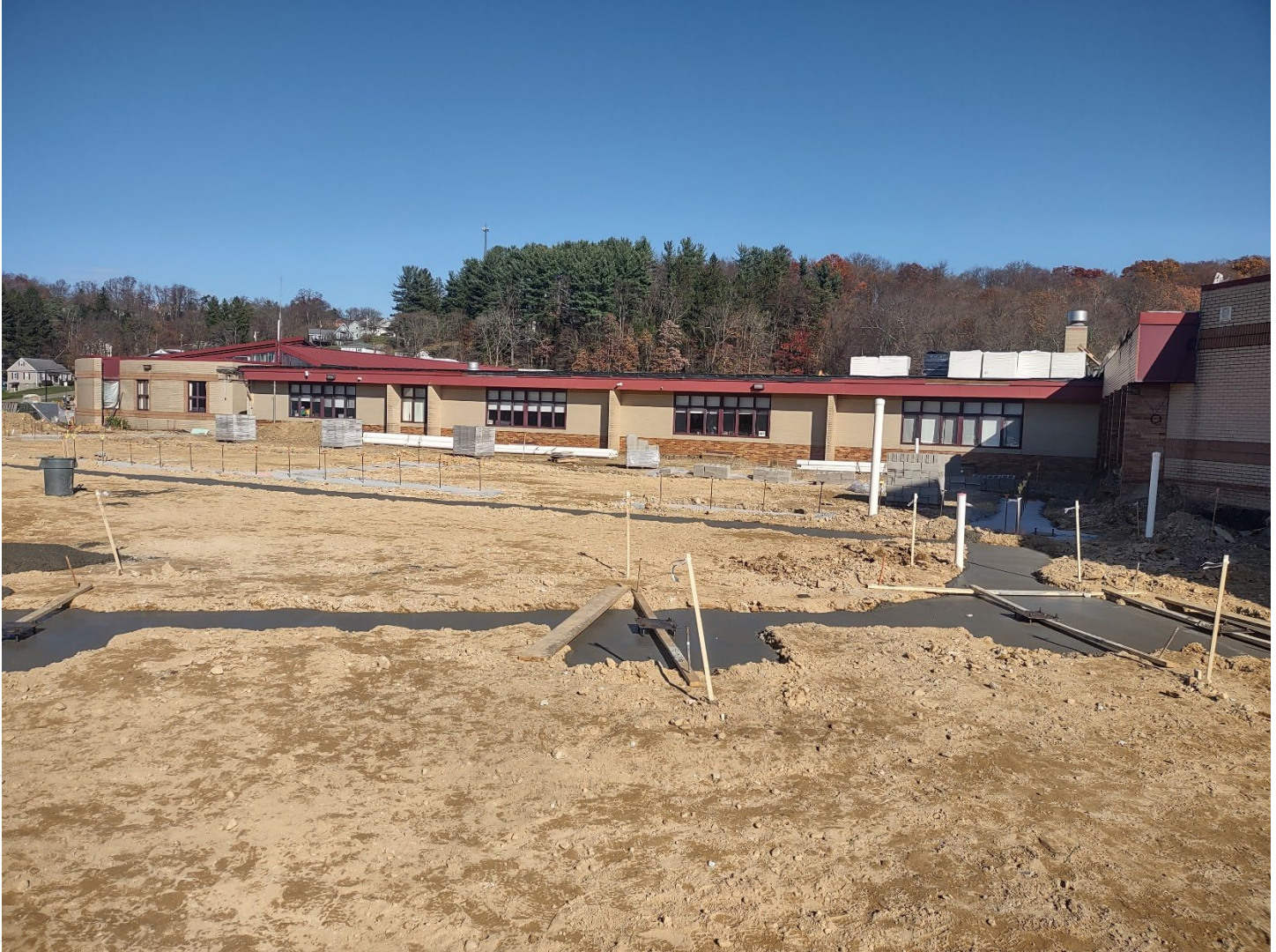
Footings and pier foundations installed for Administrative area. New classroom foundations are in background, with concrete block staged to be installed.
