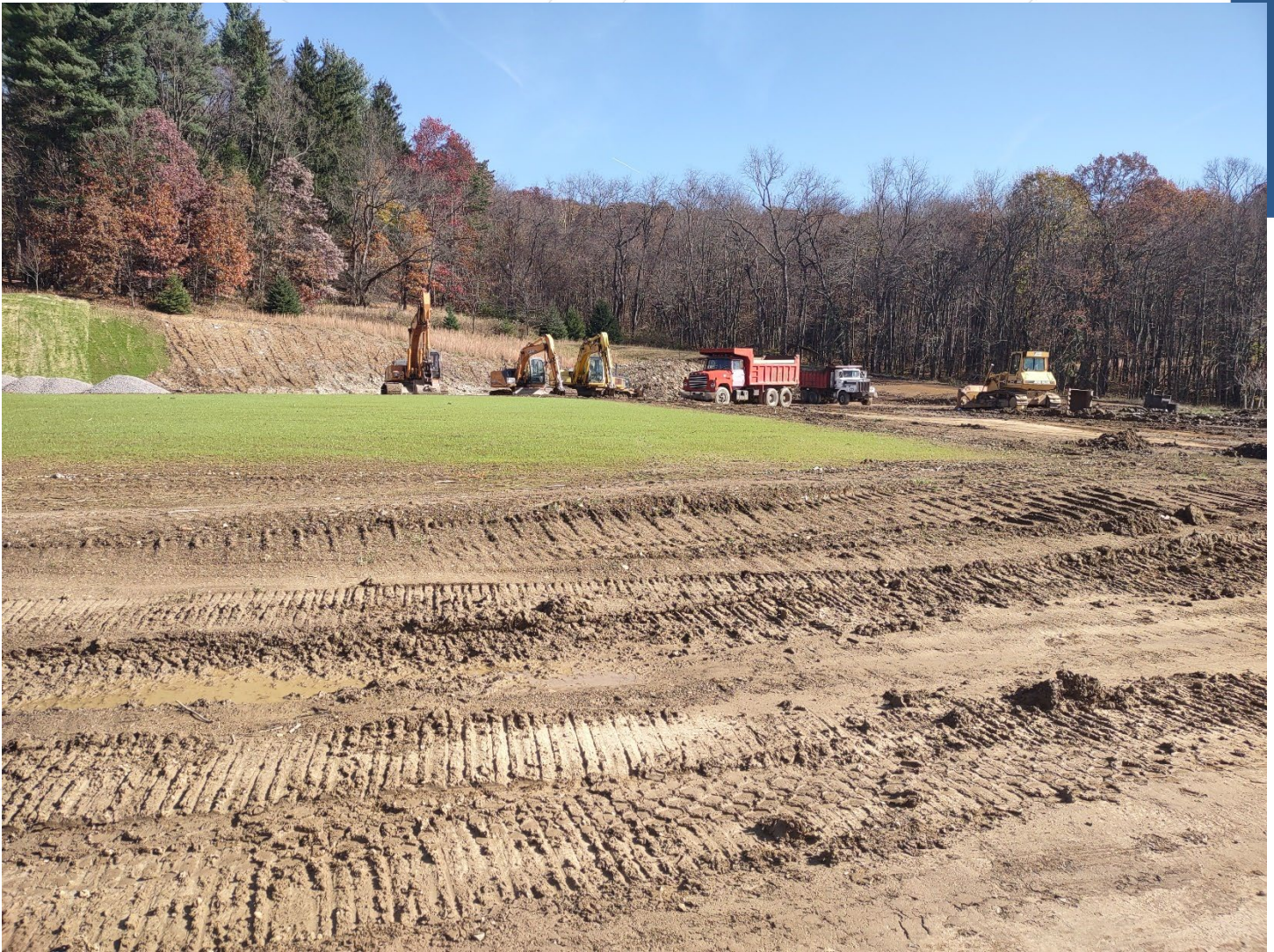
Earth moving equipment excavating the athletic field to subgrade before spreading rest of topsoil.
