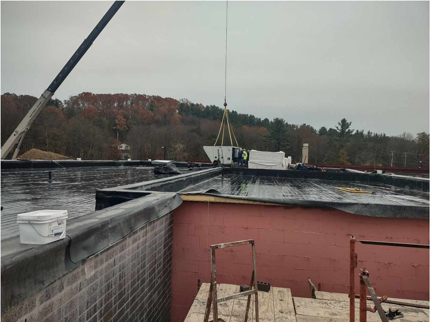
Classroom Addition and Area “B” Rooftop Units being lifted onto roof.
