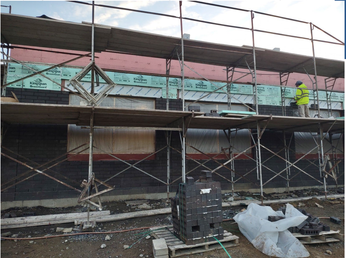
Brick Veneer being installed on Classroom addition.
