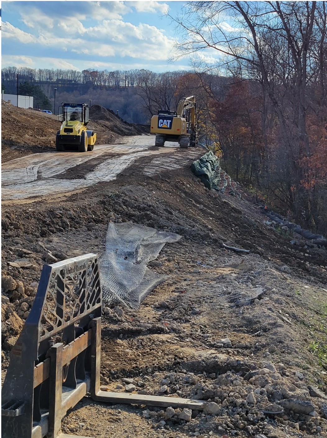
Mechanically Stabilized Earth retaining wall, soil being compacted.
