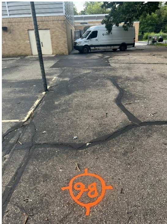
Photograph No. 12: Looking south. Pavement is flush to building. Previous patch and crack sealing visible.
