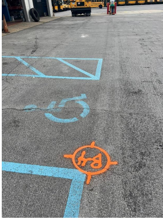
Photograph No. 7: Low severity block cracking near building.
