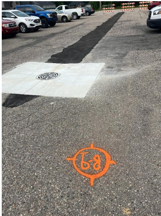
Photograph No. 18: Previous bituminous patch and new concrete collar around basin looking west.
