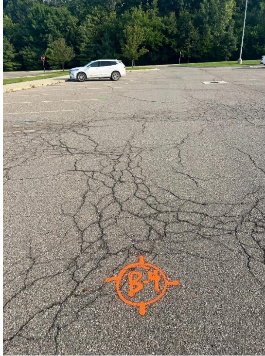
Photograph No. 7: Moderate to high severity fatigue cracking looking north toward B-4. Note concrete collar around catch basin.
