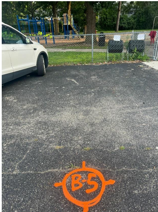
Photograph No. 10: Low severity fatigue cracking looking north playground. New concrete to the east adjacent to the school.
