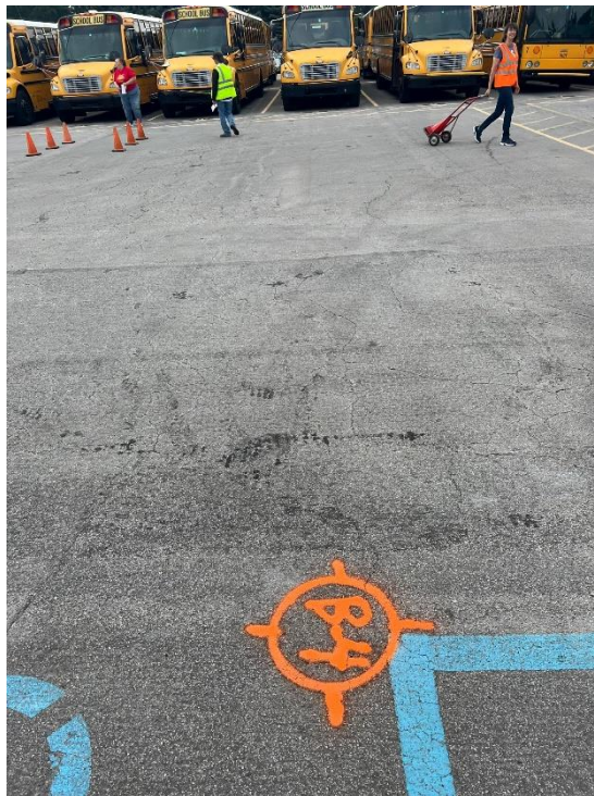
Photograph No. 8: Moderate severity fatigue cracking near bus garage.
