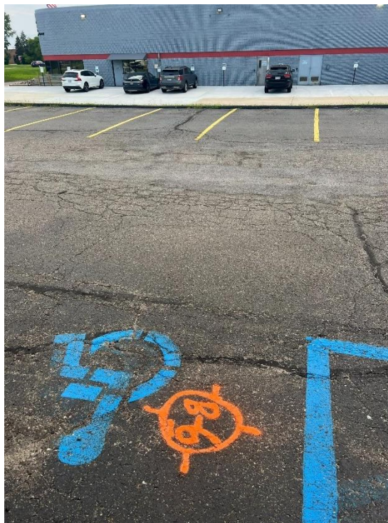
Photograph No. 14: High severity fatigue cracking and settlement evident. Previous patch constructed.
