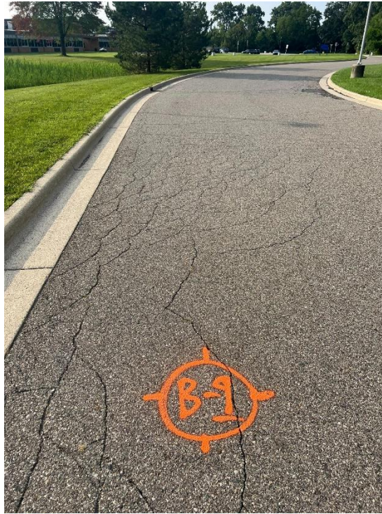
Photograph No. 15: Low to moderate severity edge cracking propagating outward. Note transverse cracking and previous patch along west side of drive. Drainage structure in gutter on east side of drive. Looking south.
