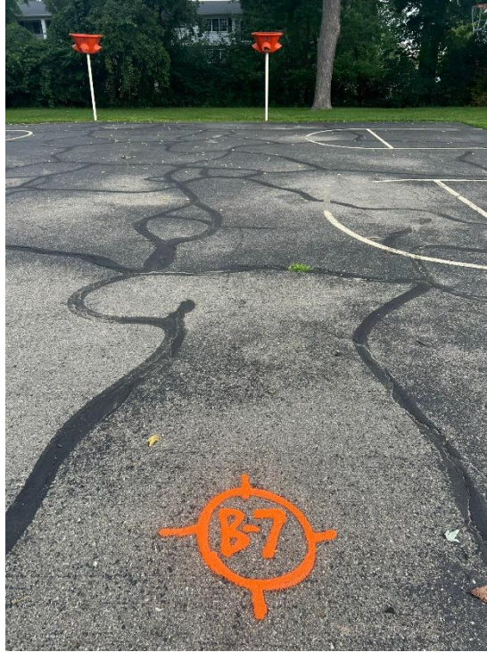
Photograph No. 13: Moderate severity cracking with previous crack sealing.
