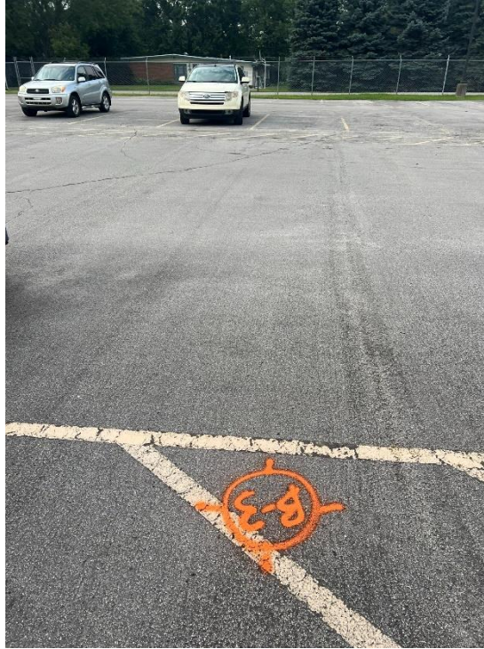
Photograph No. 5: Moderate severity cracking.
