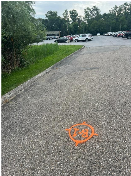
Photograph No. 2: Moderate severity edge cracking and previous patching along bituminous curb. Looking east.
