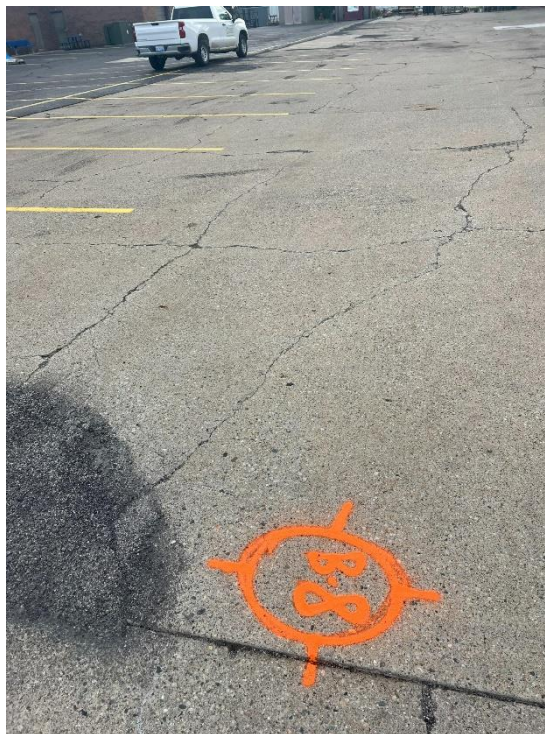
Photograph No. 18: Moderate to high severity longitudinal and transverse cracking, looking east along concrete lot.
