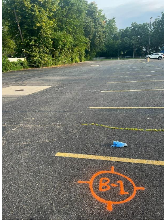
Photograph No. 1: Looking north, low to moderate severity block, joint, and fatigue cracking. Concrete collar around basin.
