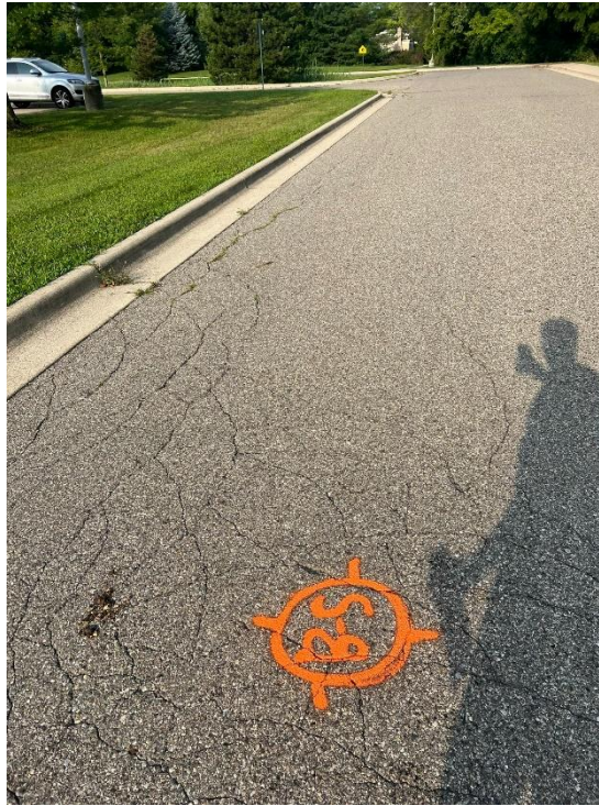
Photograph No. 9: Low to moderate severity edge fatigue cracking looking west toward B-5.
