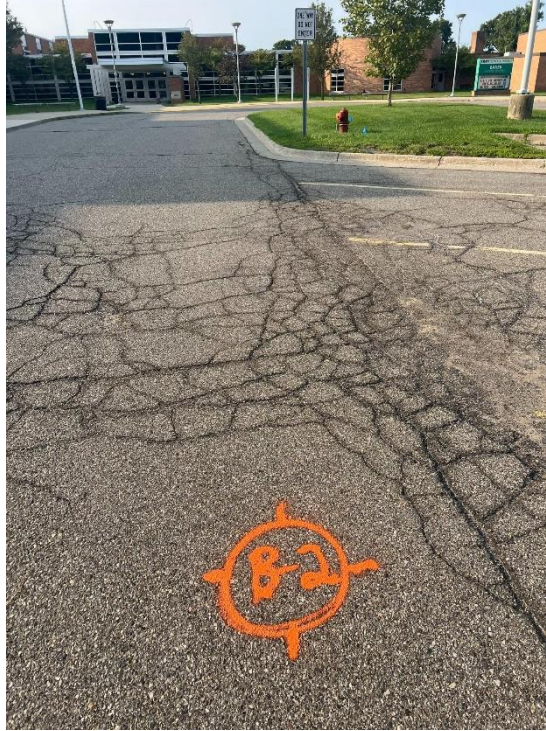
Photograph No. 3: Looking south at B-2. High severity fatigue and joint cracking.
