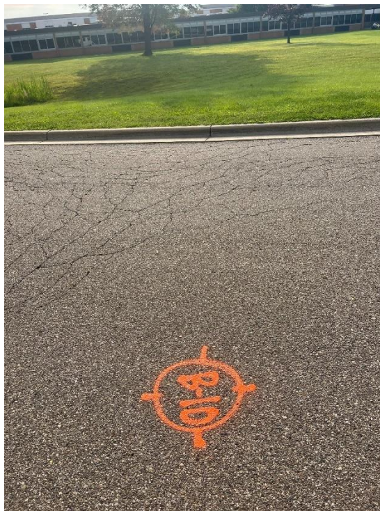
Photograph No. 18: Moderate severity transverse, fatigue, and edge cracking looking east toward B-10.
