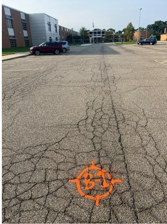
Photograph No. 1: Looking south toward B-1. High severity fatigue and joint cracking.
