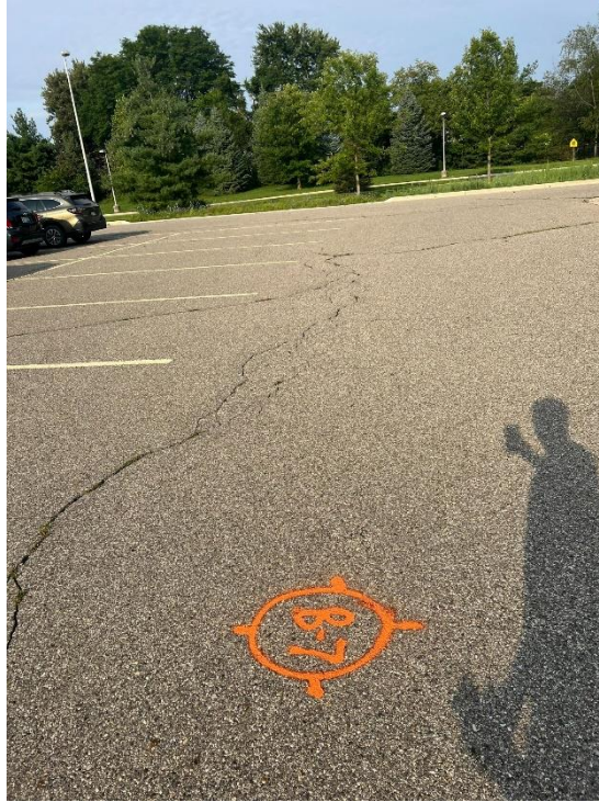
Photograph No. 13: Low to moderate severity block and fatigue cracking. Note drainage path in curb on west side of lot to drainage swale.
