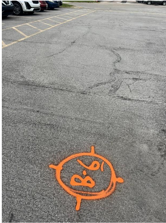
Photograph No. 11: Moderate severity block and fatigue cracking looking west toward west entrance.
