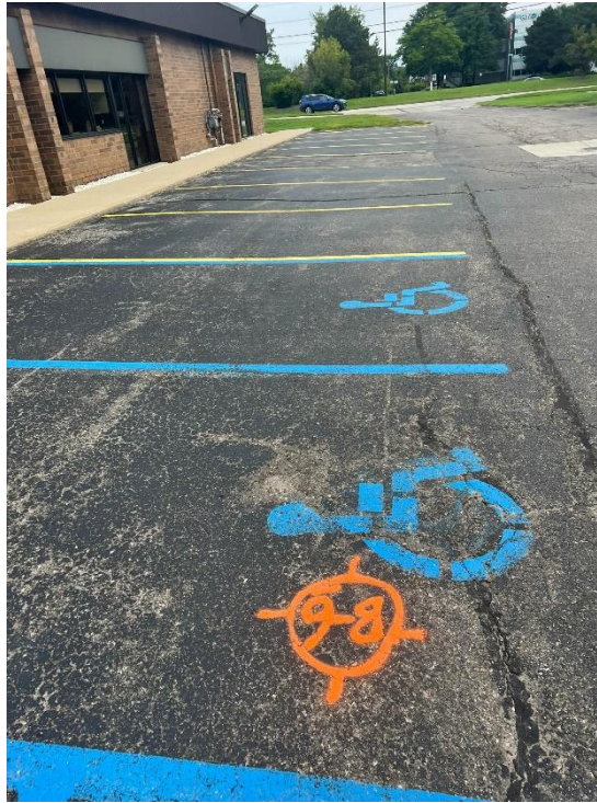
Photograph No. 13: Moderate to high severity block and joint cracking with secondary fatigue cracking looking north toward drive entrance.
