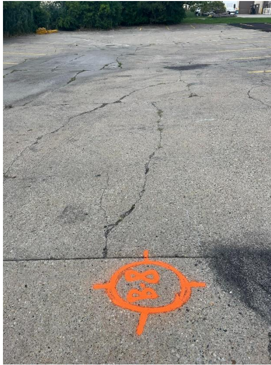
Photograph No. 17: Moderate to high severity longitudinal and transverse cracking, looking west along concrete lot.
