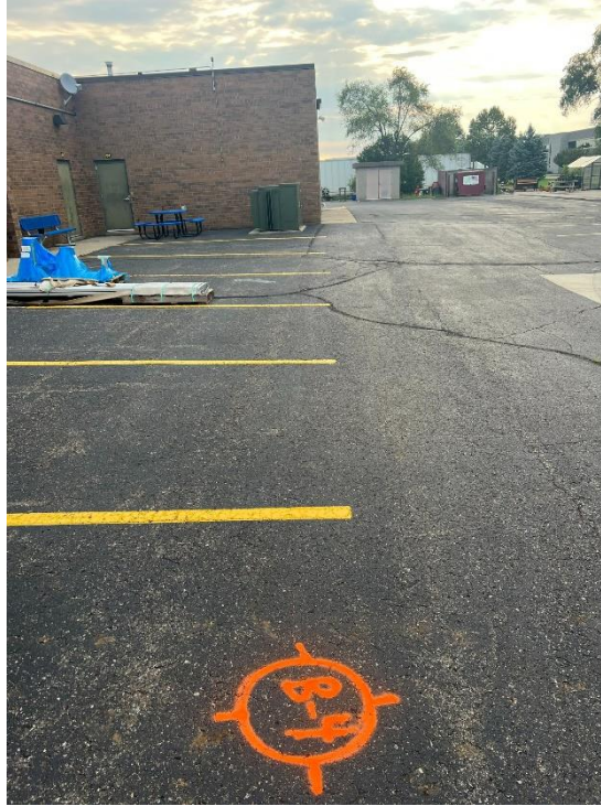
Photograph No. 9: Moderate severity block and fatigue cracking looking east. Concrete color around catch basin. Pavement flush with building.
