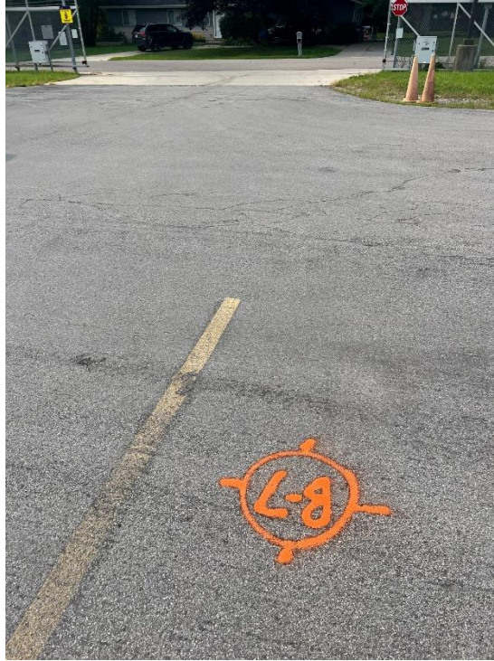
Photograph No. 13: Moderate severity block and fatigue cracking looking south at east entrance.
