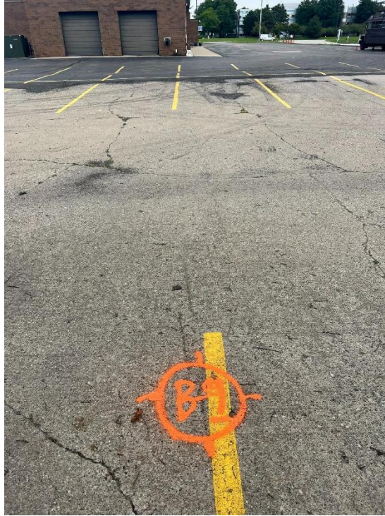
Photograph No. 19: Moderate to high severity longitudinal and transverse cracking, looking north along concrete lot.
