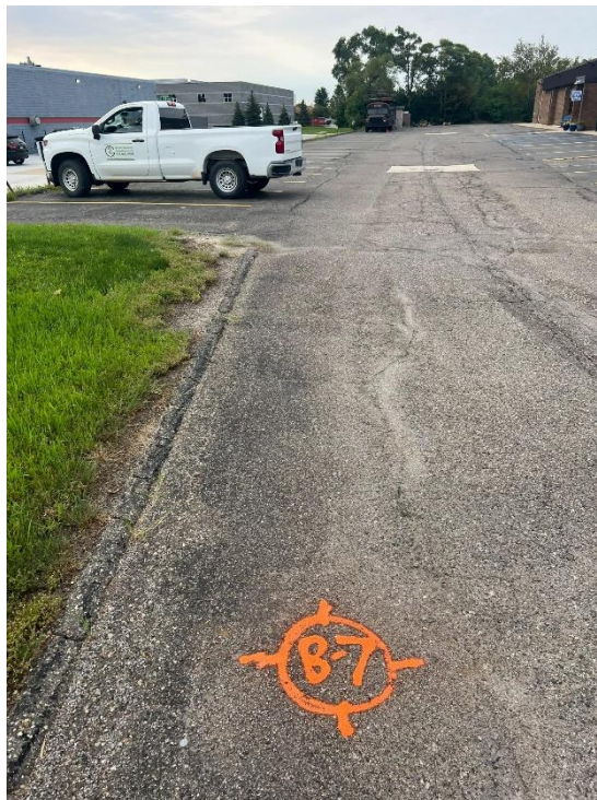
Photograph No. 16: High severity fatigue cracking at center of lot looking south from access drive.
