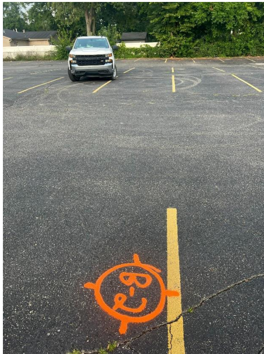
Photograph No. 4: Low to moderate severity block and fatigue cracking.
