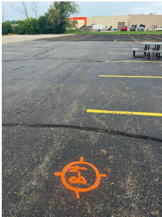
Photograph No. 8: Looking west, note the concrete pavement on the south side of the lot and newer pavement on west lot. Moderate to high severity block cracking.
