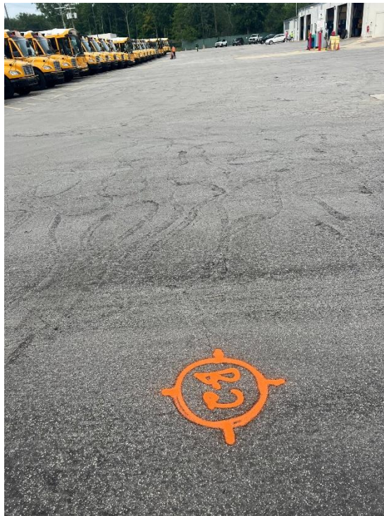
Photograph No. 4: Moderate severity fatigue cracking looking west toward B-2.
