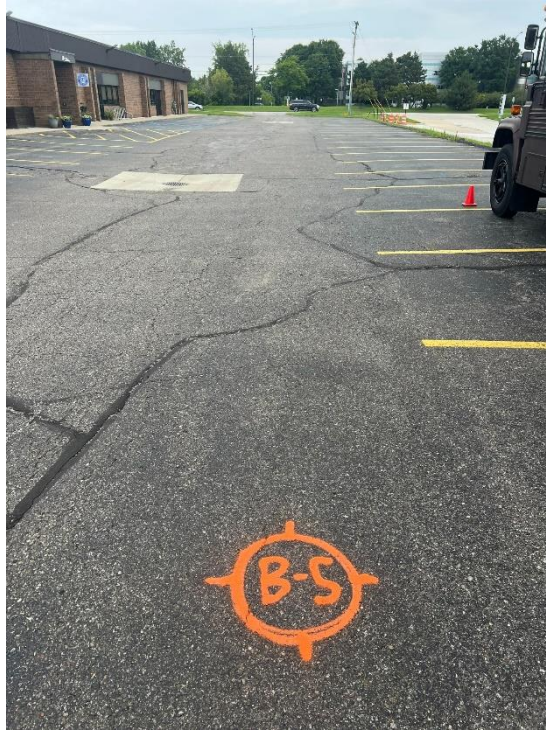
Photograph No. 11: Moderate severity block cracking with moderate to high severity fatigue cracking propagating outward, looking north along east lot.
