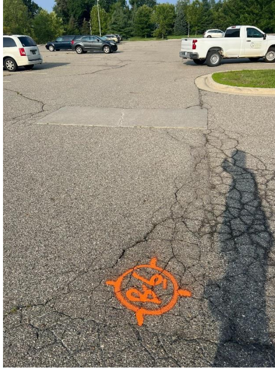
Photograph No. 11: Moderate to high severity fatigue and block cracking looking west toward B-6. Note previous concrete patch.
