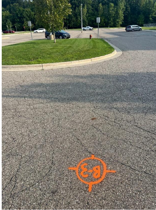
Photograph No. 5: Looking north toward B-3. Low to moderate severity fatigue and cracking.
