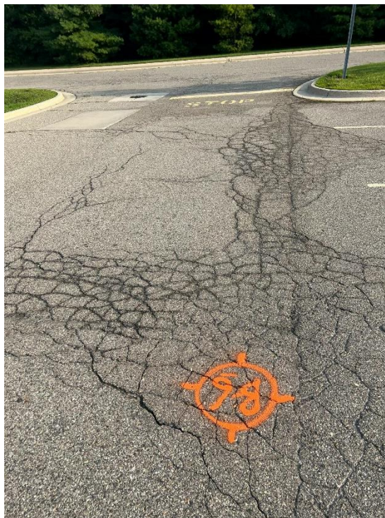
Photograph No. 10: High severity fatigue and joint cracking looking north toward B-6. Note concrete collar around basin and patch south of basin.
