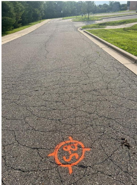
Photograph No. 8: Moderate severity fatigue and edge cracking, looking east toward B-5.
