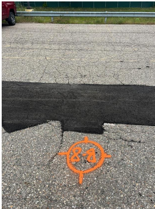
Photograph No. 16: High severity fatigue cracking In parking stalls.
