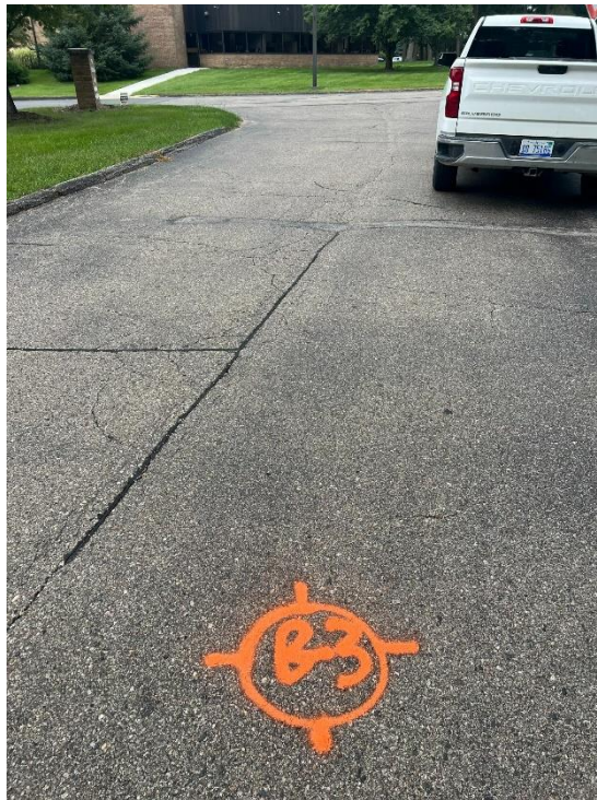
Photograph No. 6: Moderate severity block, joint, and fatigue cracking looking west toward drive entrance.
