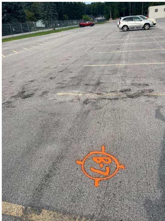
Photograph No. 14: Low to moderate severity joint and fatigue cracking looking west along south side of lot.
