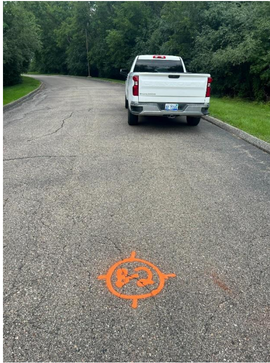
Photograph No. 3: Looking west. Low to moderate severity fatigue and edge cracking. Evidence of ponding along south curb line.
