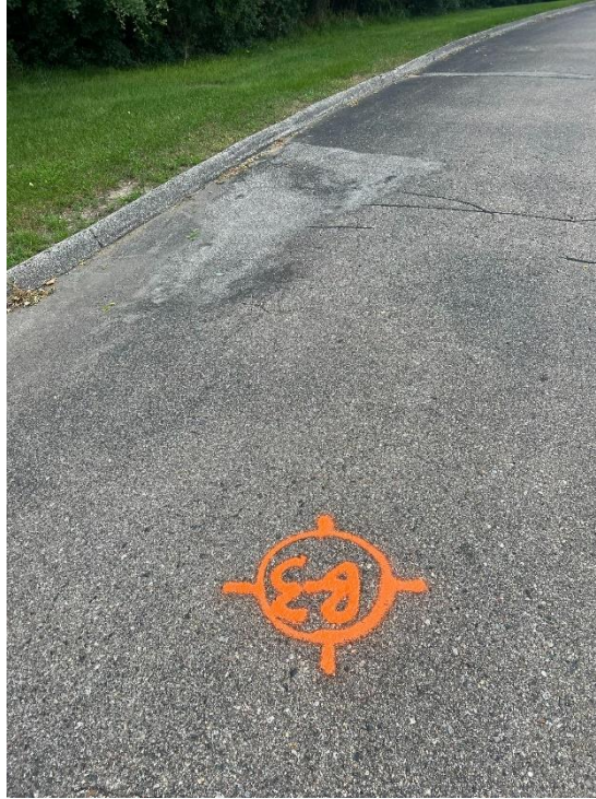
Photograph No. 5: Moderate severity fatigue cracking and patch along north curb line, looking east toward B-3.
