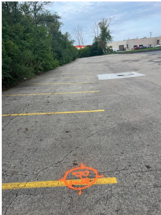
Photograph No. 20: Moderate to high severity longitudinal and transverse cracking, looking west along concrete lot.
