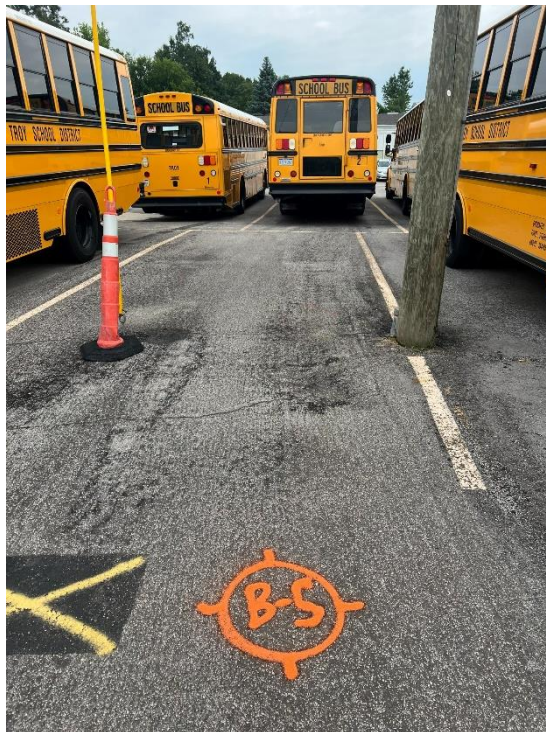
Photograph No. 10: Low severity transverse cracking.
