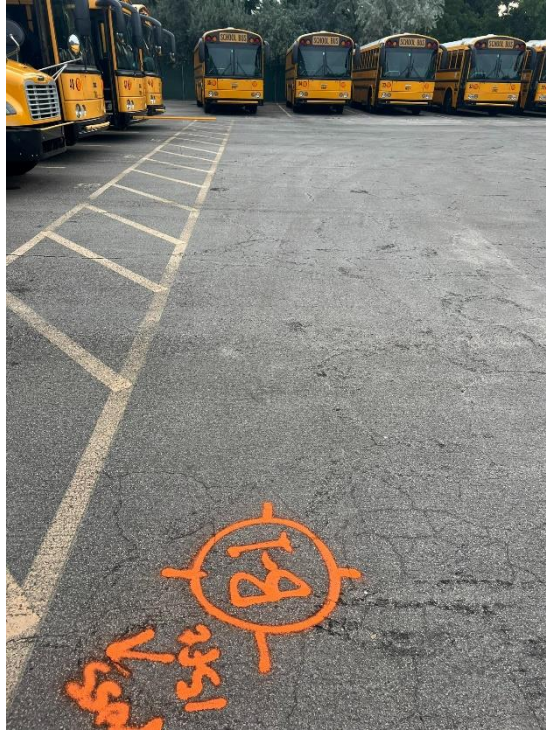
Photograph No. 1: Moderate severity fatigue and block cracking looking east.
