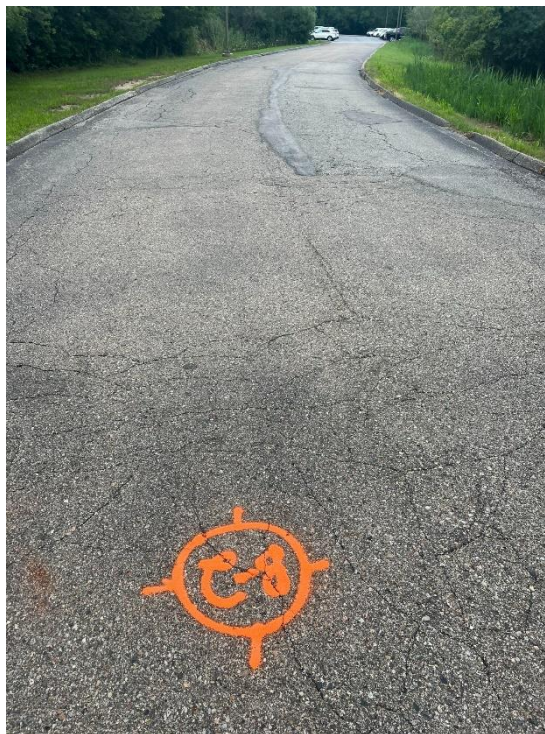
Photograph No. 4: Moderate severity fatigue cracking looking east toward B-2. Previous patching along curb line and center.
