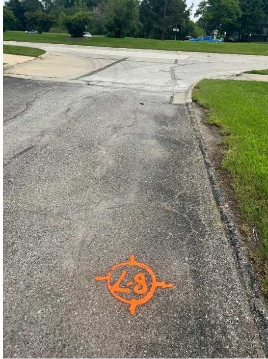
Photograph No. 15: Moderate fatigue cracking at east entrance. Note asphalt curb.
