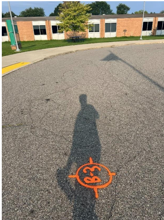
Photograph No. 4: Looking west at B-3. Low severity fatigue Cracking at access loop.
