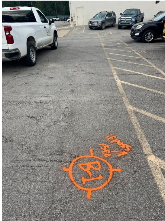
Photograph No. 2: Moderate severity fatigue cracking looking west. Pavement surface showing weathering.
