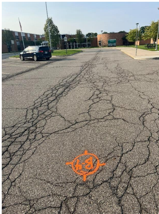
Photograph No. 6: Look south at B-4. High severity joint and fatigue cracking.
