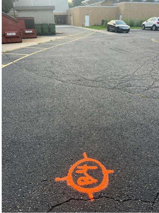
Photograph No. 7: Moderate severity fatigue cracking looking east.
