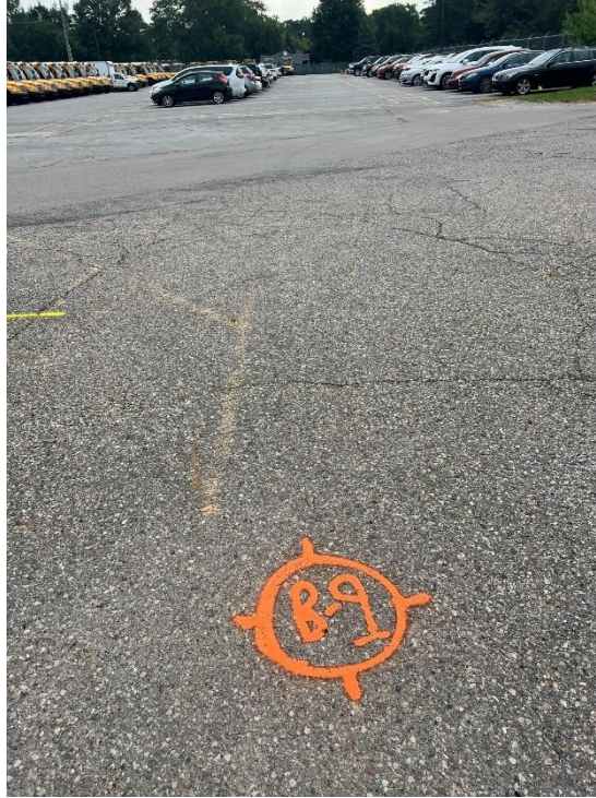
Photograph No. 17: Low severity fatigue cracking looking east along south side of the property. Previous patch crossing west entrance drive.
