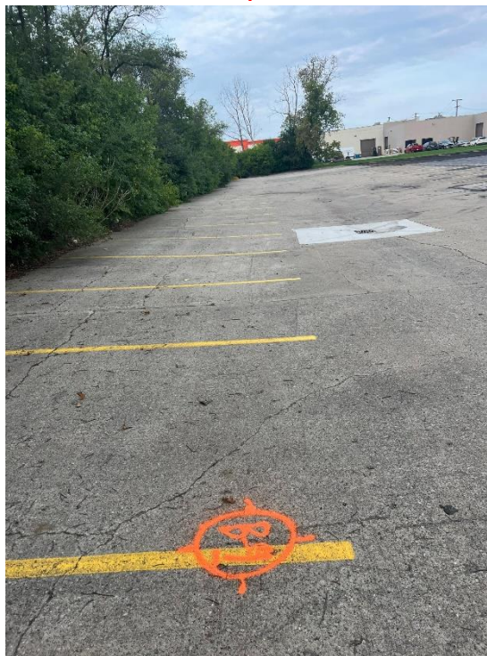
Photograph No. 10: Concrete pavement at south side of lot. Moderate severity fatigue cracking.
