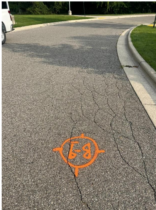
Photograph No. 16: Low to moderate severity edge cracking propagating outward. Looking north.
