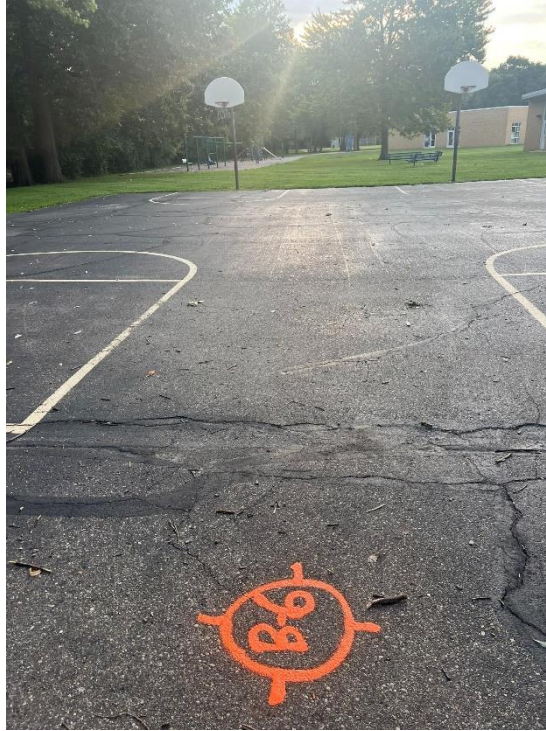
Photograph No. 11: Moderate to high severity fatigue cracking and settlement evident.
