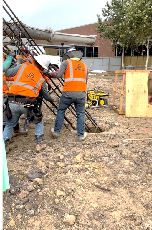
Concrete pier installation
