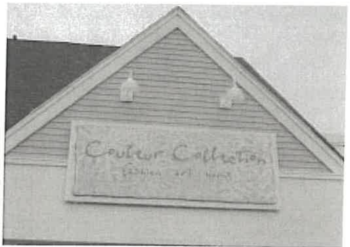
These facade-mounted lighting fixtures are visually compatible with the form and color of the building.
