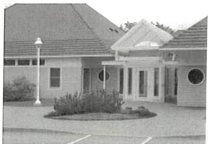
The color, form, and line of this fixture reflect the contemporary design of this office building. Its height and placement contribute to the human scale of the entrance.
