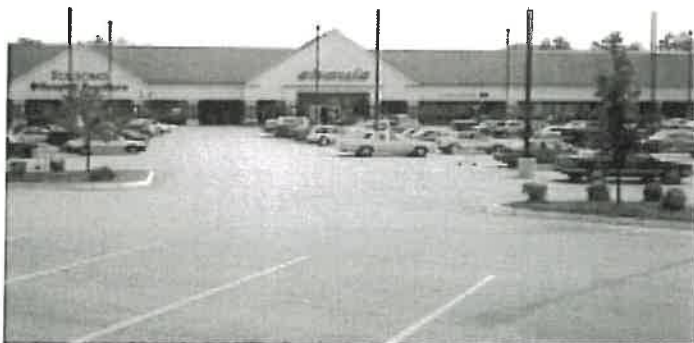
An example of lighting fixtures which are taller than the main building and out of scale with the site.
