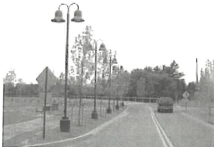
Driveway lighting effectively used to add character to a new road and illuminate the adjacent sidewalk
