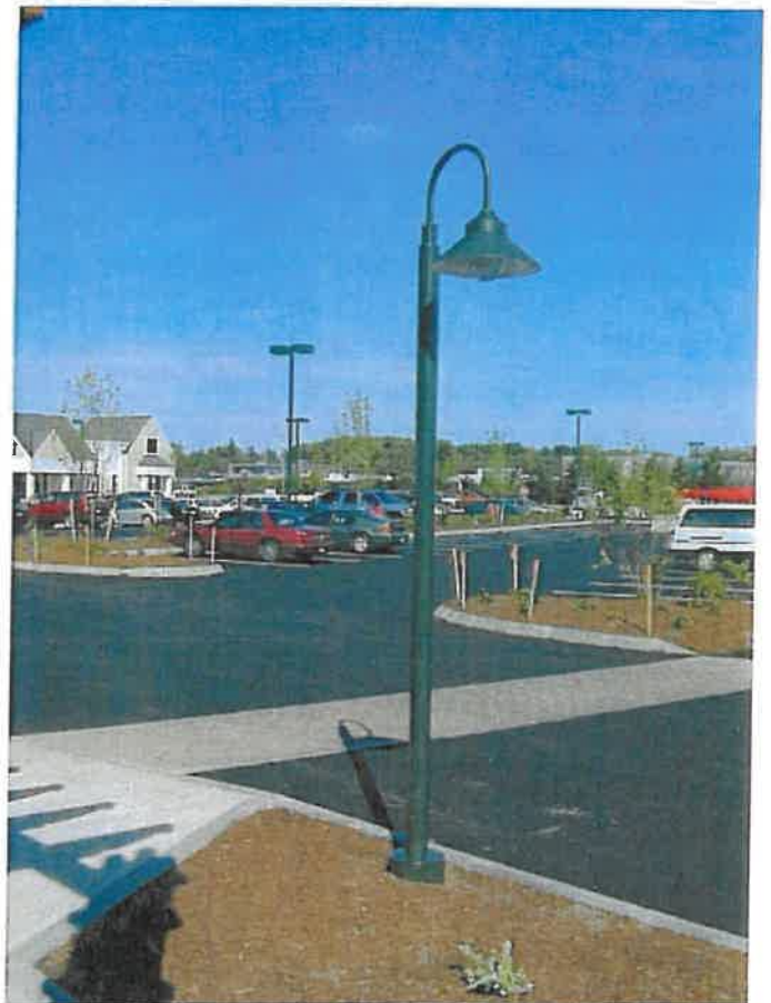
This light fixture at a crosswalk in a parking is scaled to the pedestrian.
