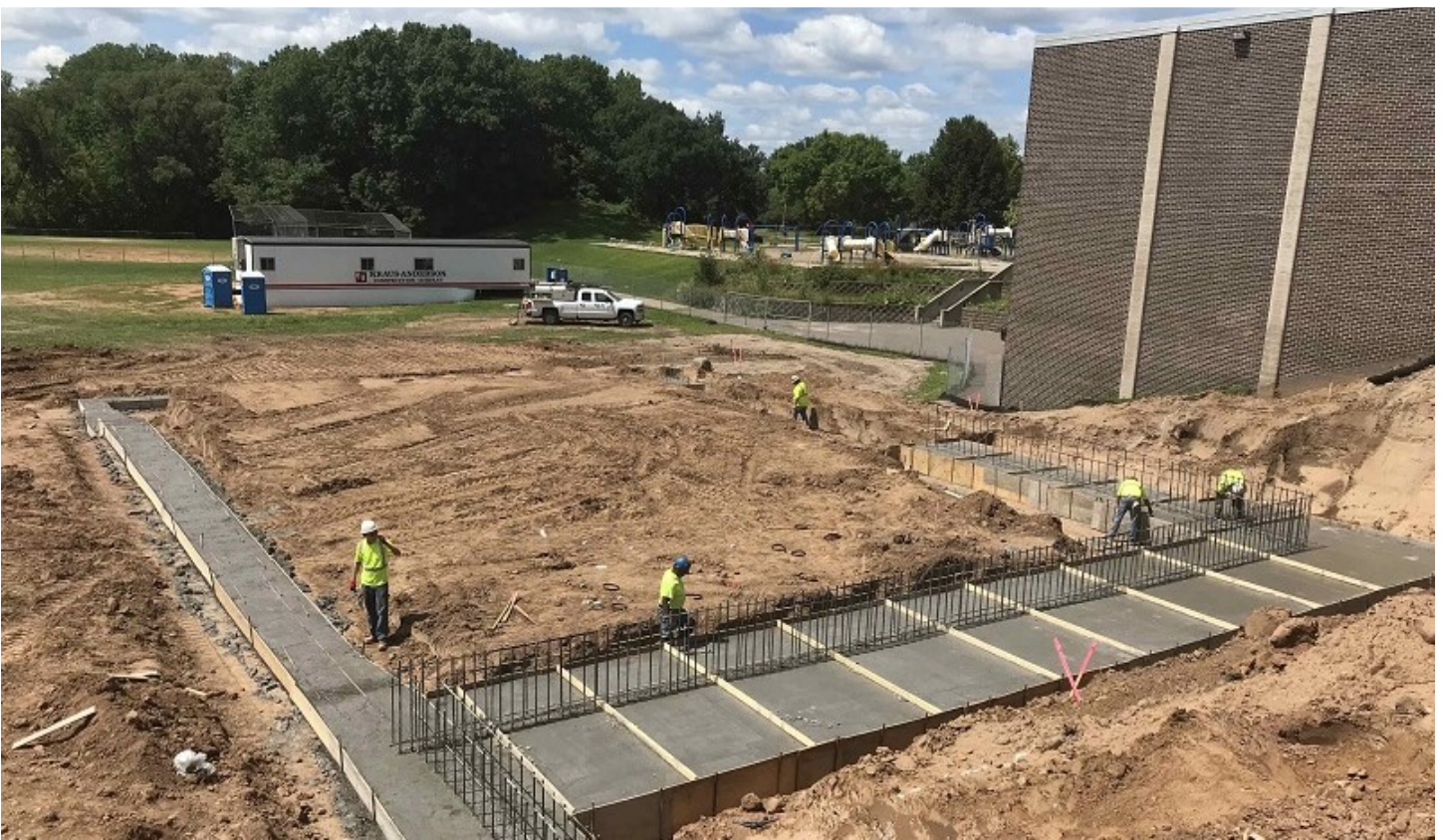
From top to bottom: Formwork placed for concrete footings; concrete footings poured for new building addition. (July 2020)
