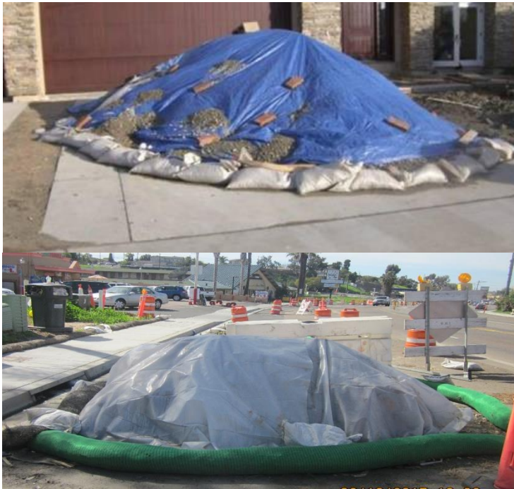
Cover and containment for stockpile
