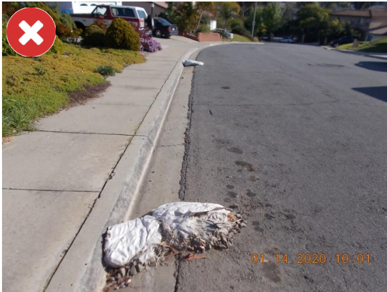
Damaged check dams, wrong orientation
