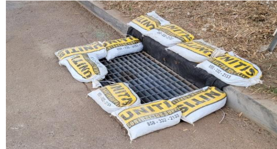
Gravel bag berm and filter fabric
