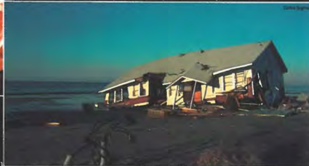
▲ The rain from Hurricane Floyd caused the worst flooding in North Carolina in recent memory. Water from the Tar and Neuse rivers covered 66 counties, destroying over 4,000 homes and killing 51 people.
