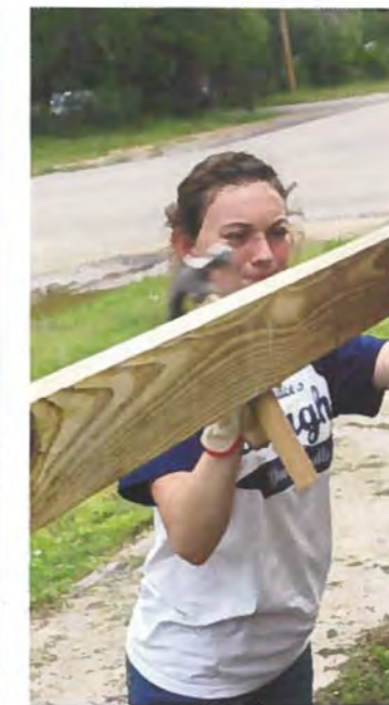
Left: Working hard to finish her group's project, Sophomore Genevieve Devlin helps her team to level and hammer in the first board of the fence they are building.
