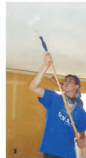
Left: After helping tear down and rebuild a ceiling almost from scratch, Junior J.L. Bronold proudly paints the finished product, intent on seeing the project through to the end.
