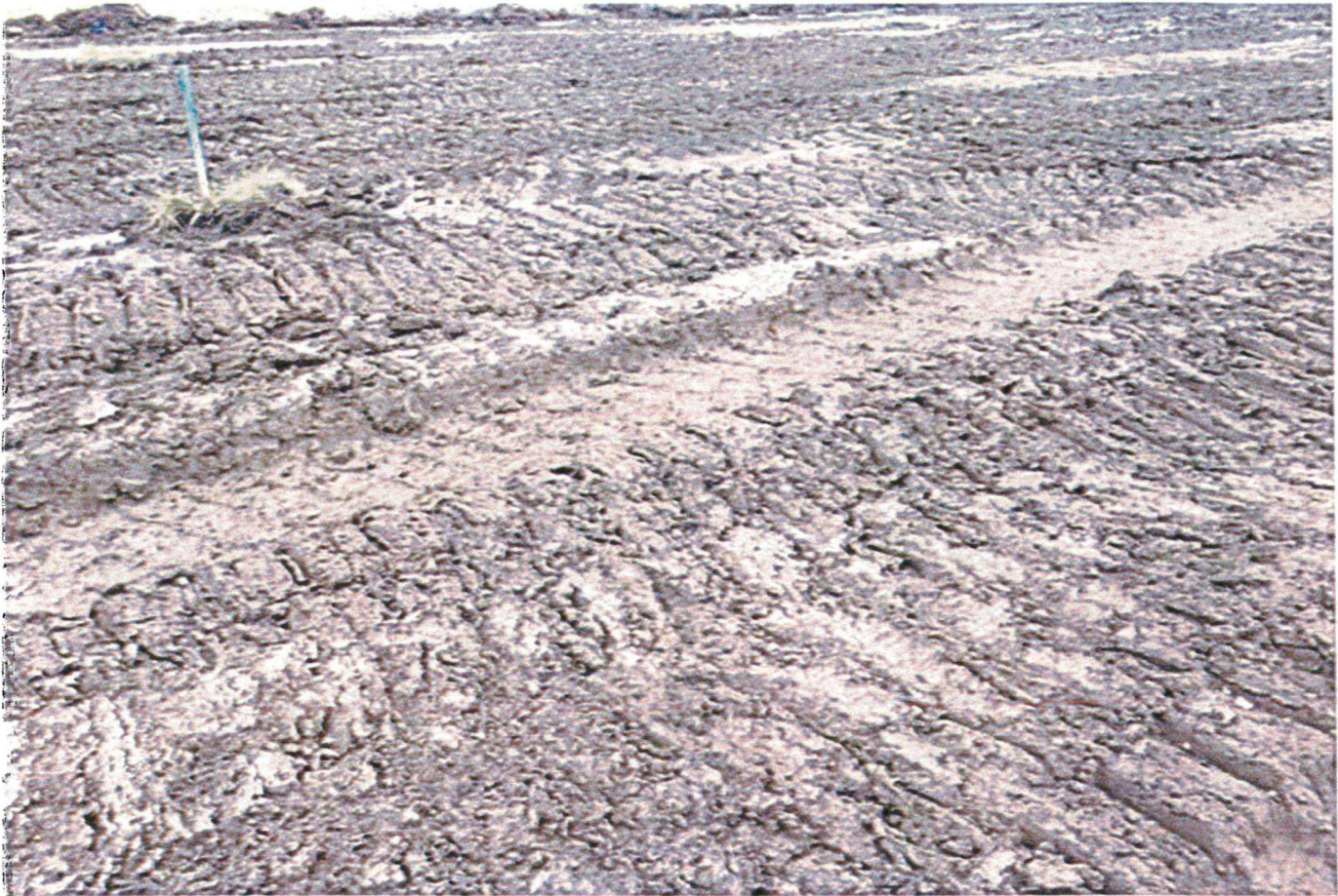
View of existing sub grade soils.
