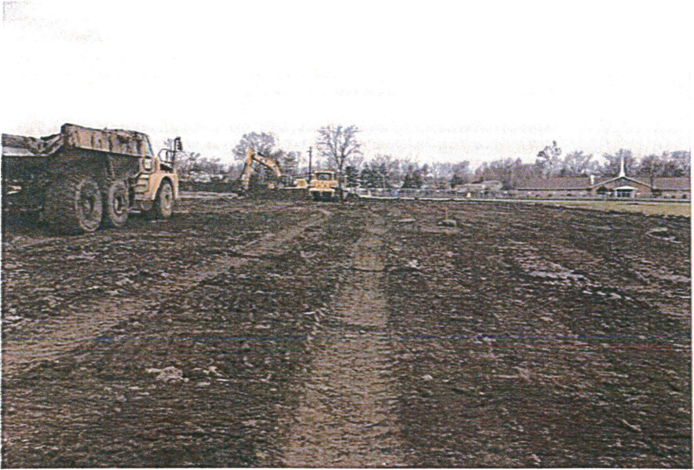
View of proof roll area looking west.
