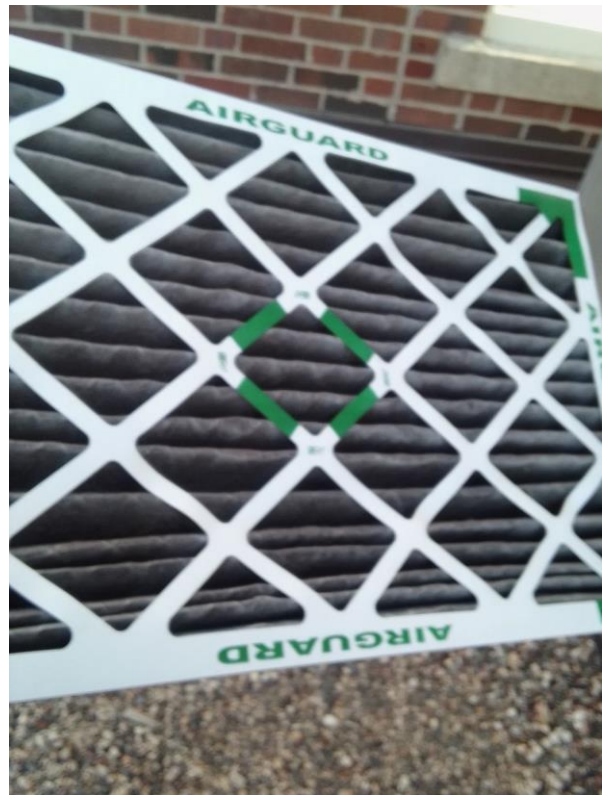
RTU-01 Mixed Main Filter Cleanliness
