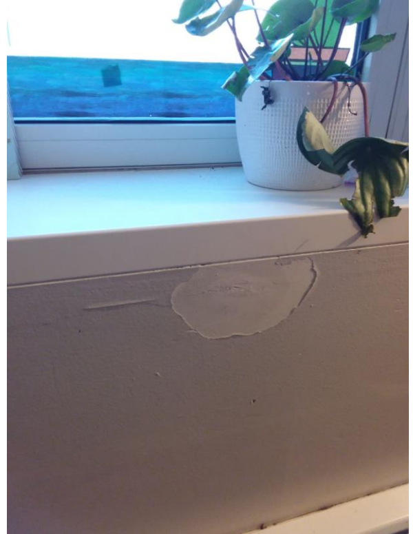
Bubbling/Peeling Paint
