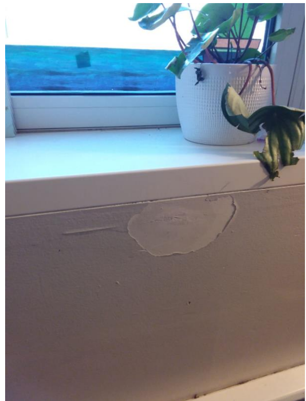
Bubbling/Peeling Paint
