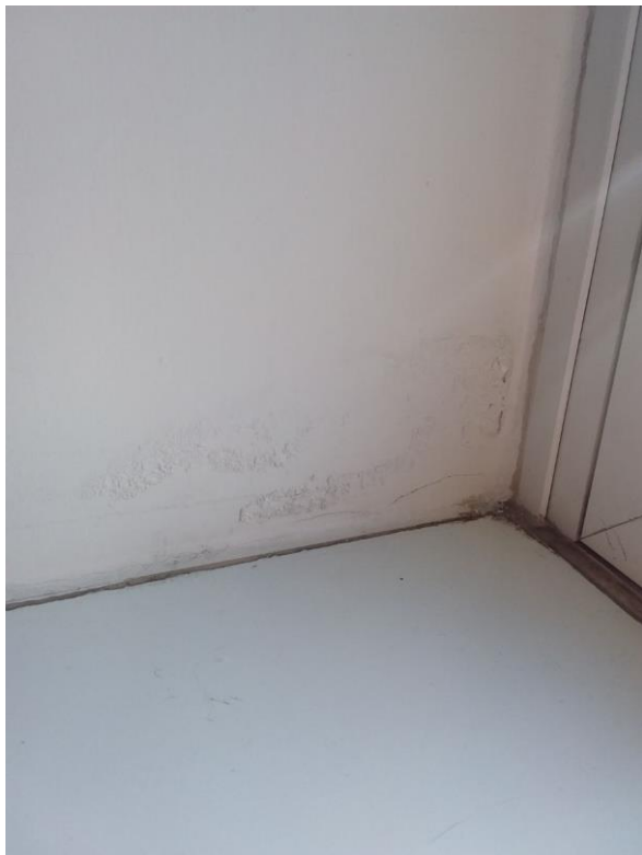
4110 Bubbling/Peeling Paint
