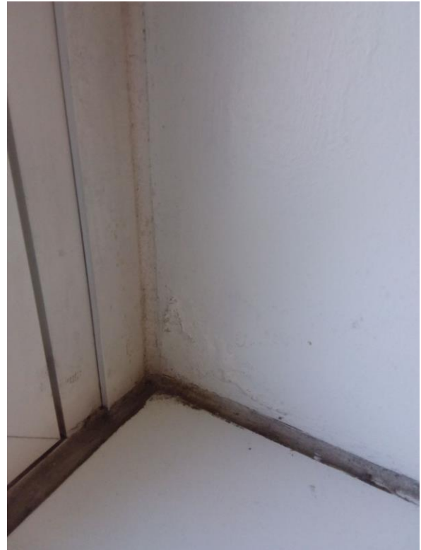
Bubbling/Peeling Paint
