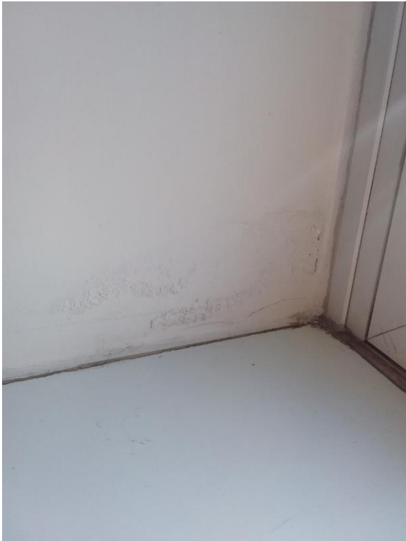
4110 Bubbling/Peeling Paint
