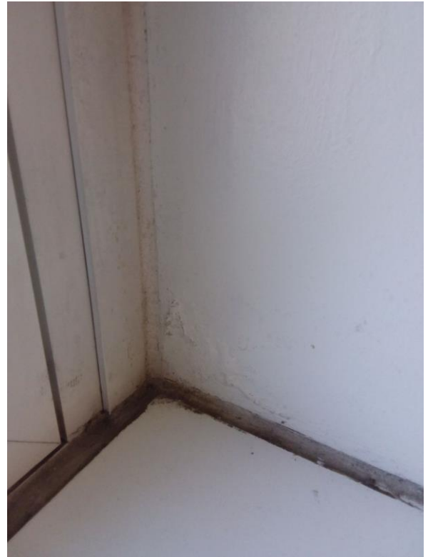
Bubbling/Peeling Paint
