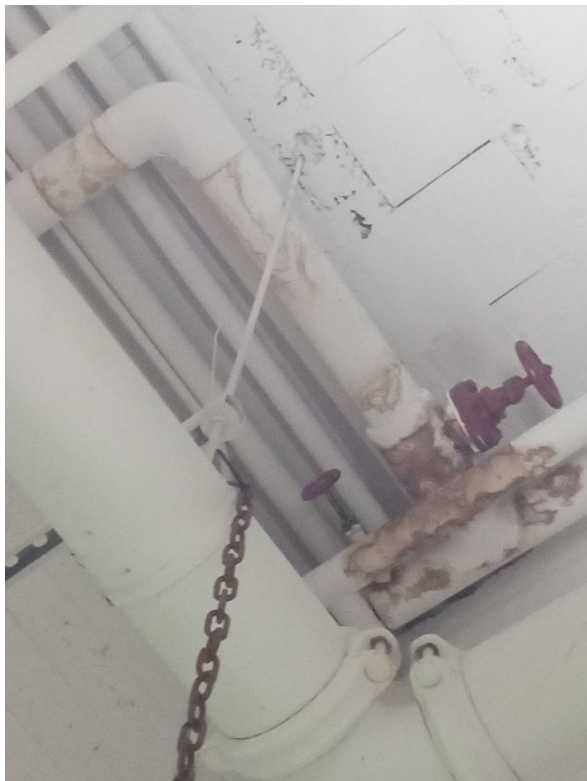
CUSTODIAL OFFICE Moisture Impacted Materials
