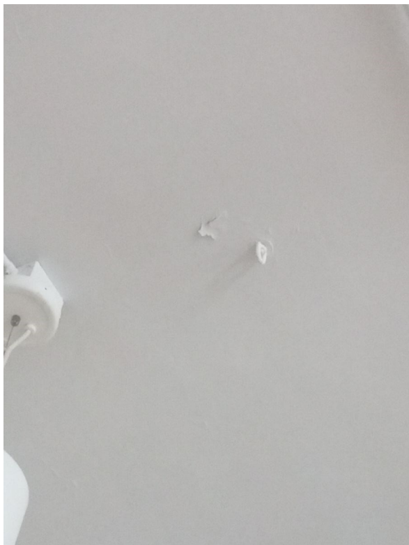
1112 Bubbling/Peeling Paint
