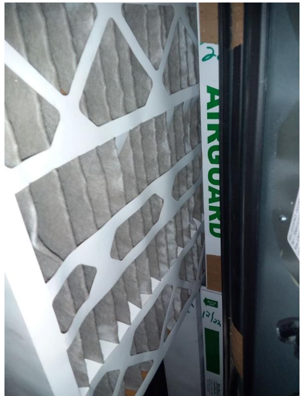
AHU-13 Mixed Main Filter Cleanliness
