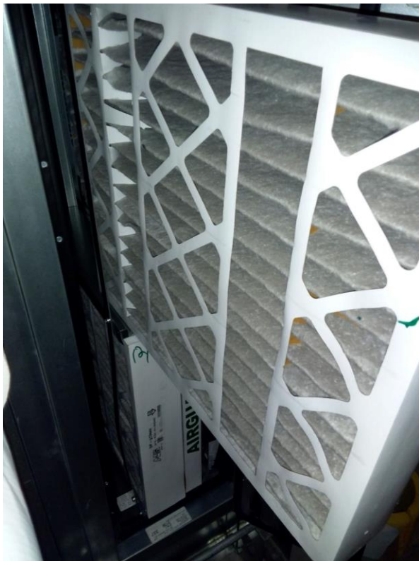
AHU-12 Mixed Main Filter Cleanliness
