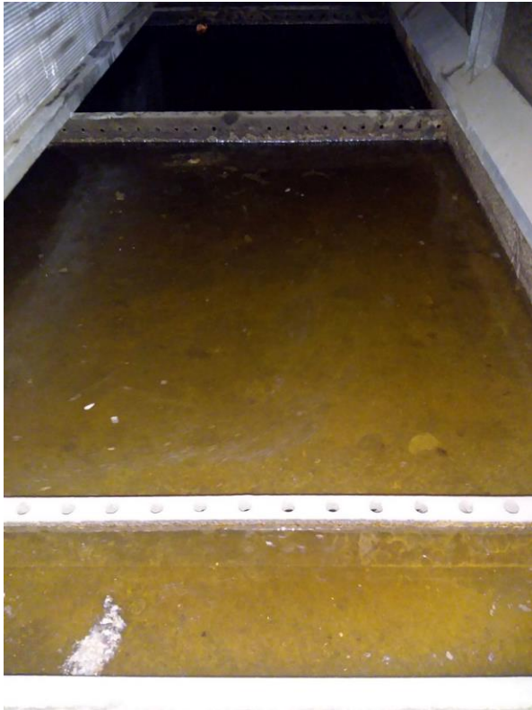
AHU-10 Drain Pans
