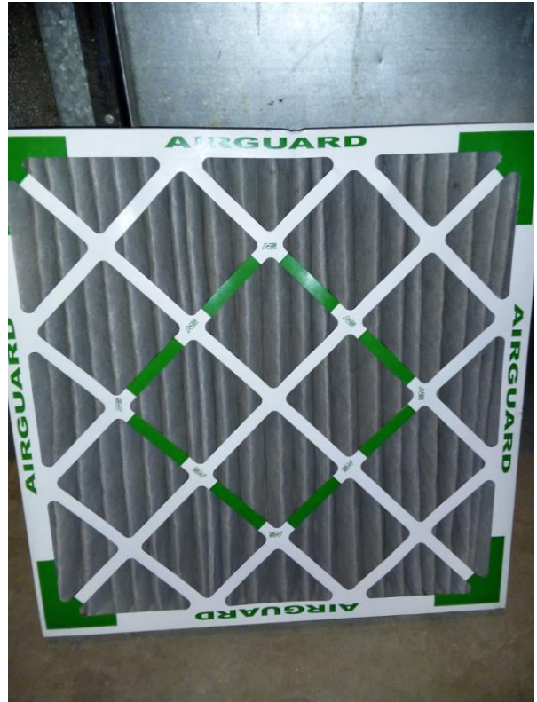
AHU-11 Mixed Main Filter Cleanliness
