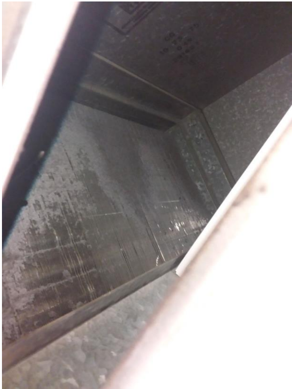
HVU_03 Heating Coils
