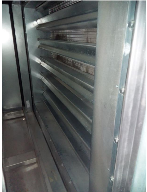
AHU_16 Heating Coils
