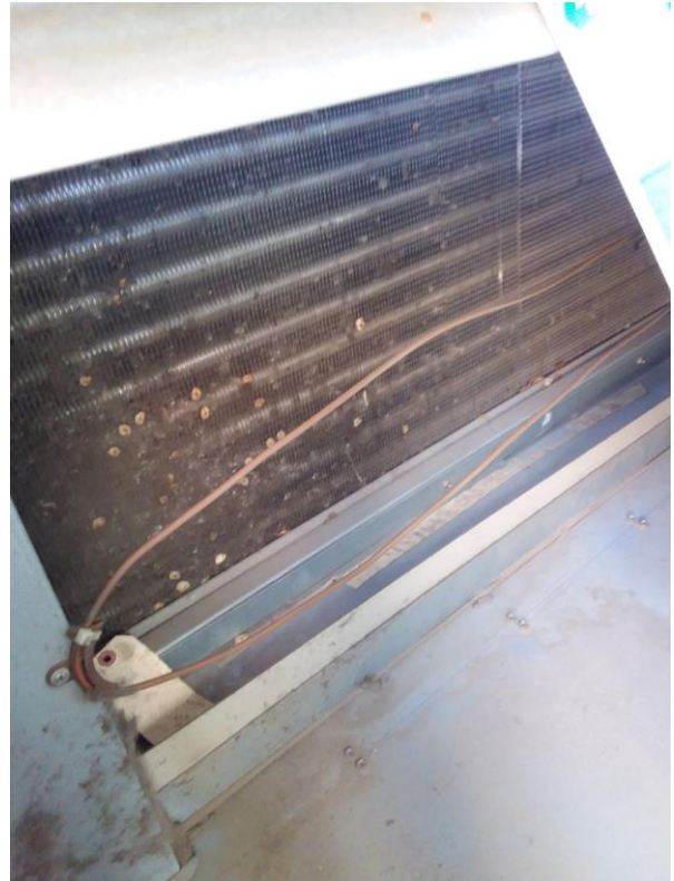
RTU_02 Heating Coils
