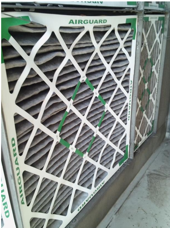
RTU_03 Mixed Main Filter Cleanliness
