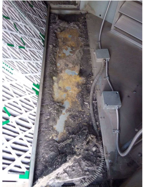
RTU_B1 General Condition
