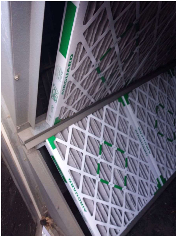
RTU_B3 Mixed Main Filter Fit
