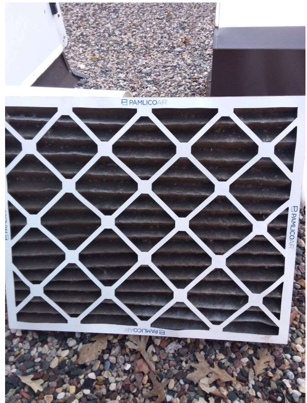
ERU_B1 (ERV-1) Outdoor Main Filter Cleanliness
