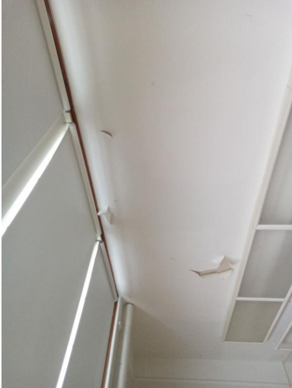
2303 Bubbling/Peeling Paint
