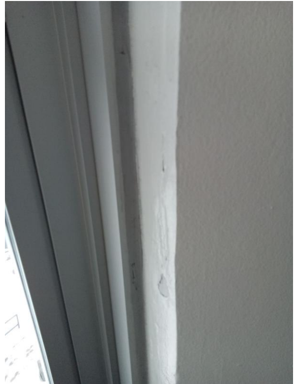
2111 Bubbling/Peeling Paint
