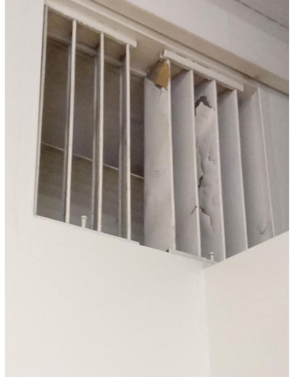
2301 Bubbling/Peeling Paint
