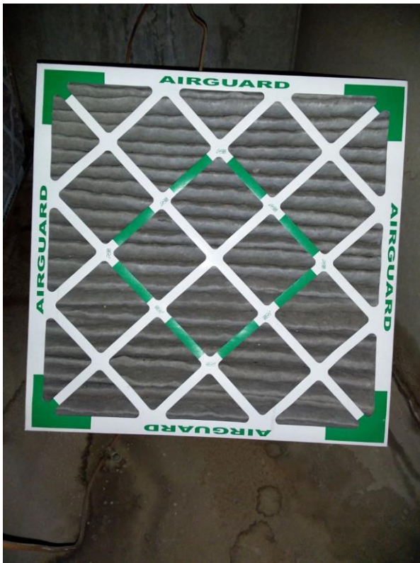
AHU 08 Mixed Main Filter Cleanliness
