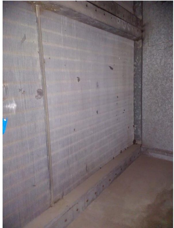
AHU 12 Heating Coils
