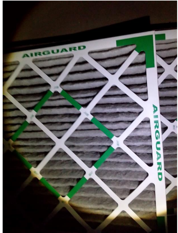
AHU 07 Mixed Main Filter Cleanliness
