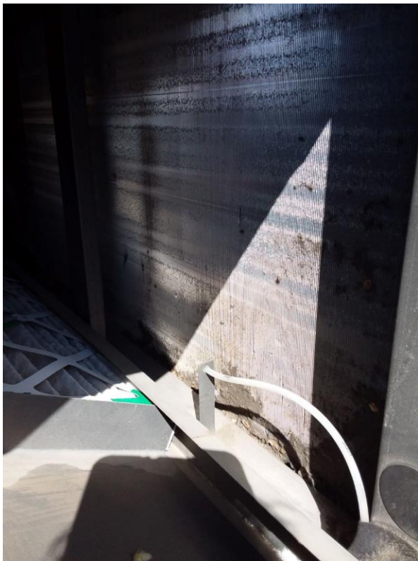
RTU 03 Heating Coils
