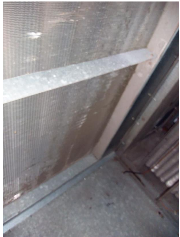
AHU-7 Heating Coils
