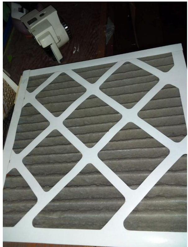
AHU-11 Mixed Main Filter Cleanliness
