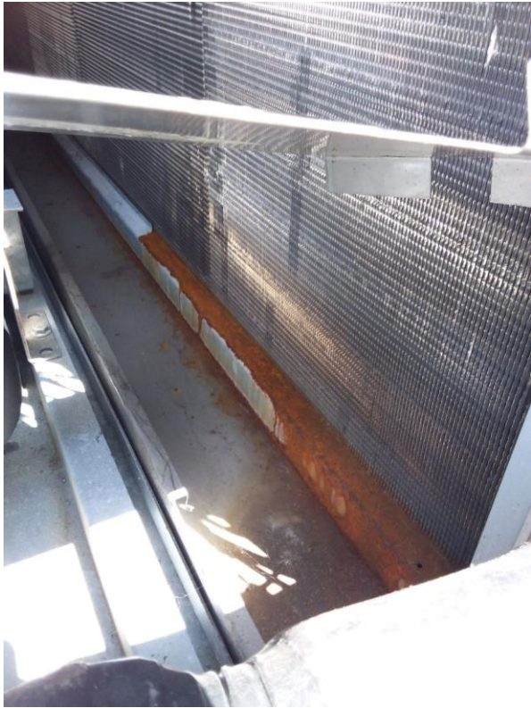
RTU-04 Drain Pans
