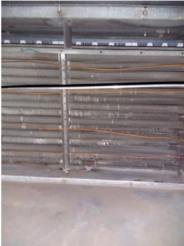
AHU-7 Heating Coils
