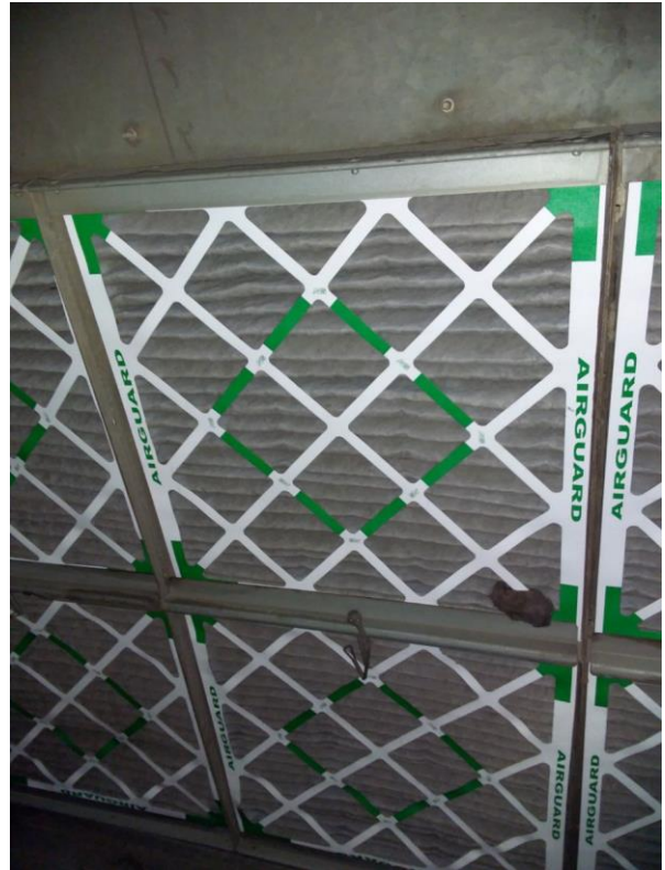
AHU-4B Mixed Main Filter Cleanliness
