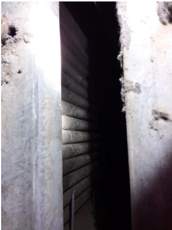
AHU-10 (100% RA) Heating Coils
