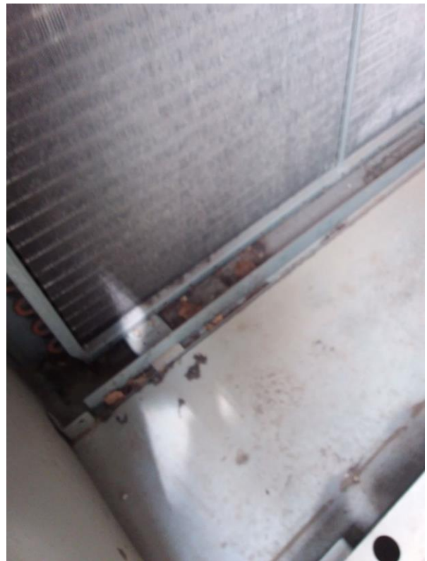
RTU-01 Drain Pans
