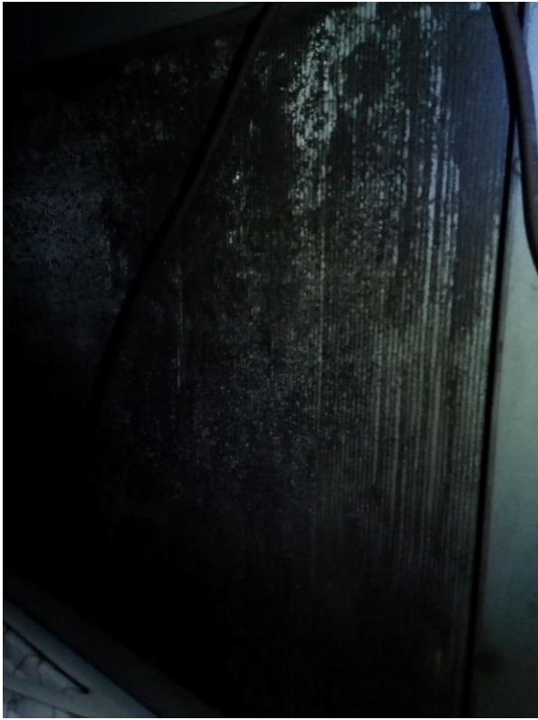
HVU 01 Heating Coils
