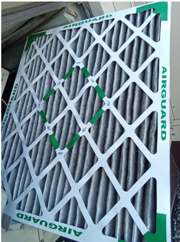
RTU 04 (100% OA) Outdoor Main Filter Cleanliness
