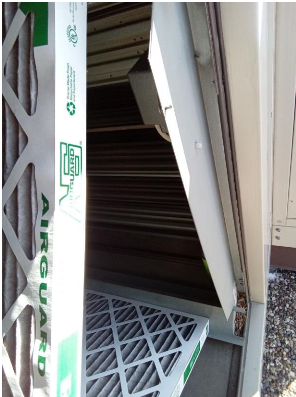
RTU 05 (100% OA) Outdoor Main Filter Fit
