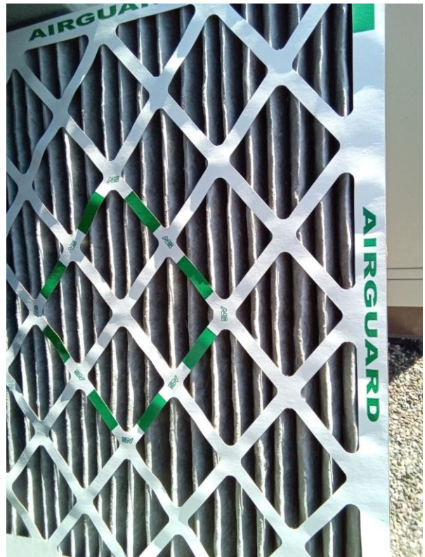
RTU 05 (100% OA) Outdoor Main Filter Cleanliness
