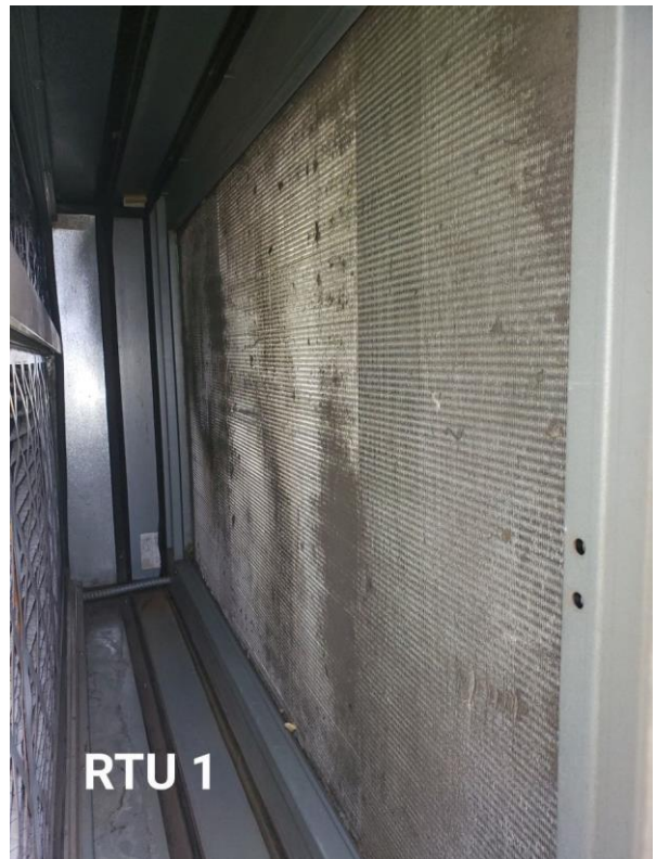
RTU_01 Heating Coils
