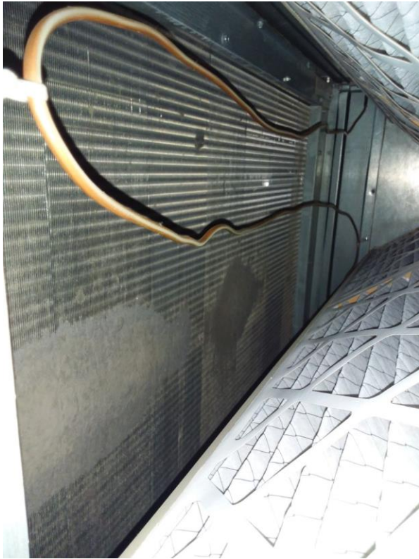
AHU-02 Cooling Coils
