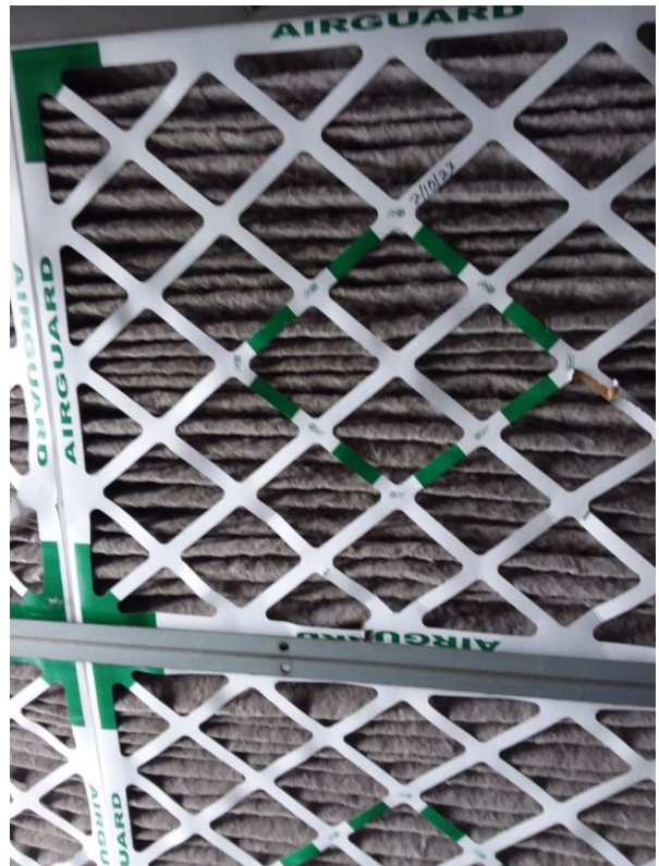
RTU-01 Mixed Main Filter Cleanliness
