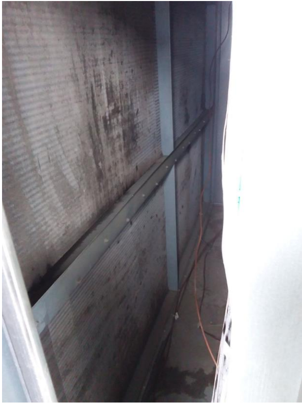
RTU-01 Heating Coils
