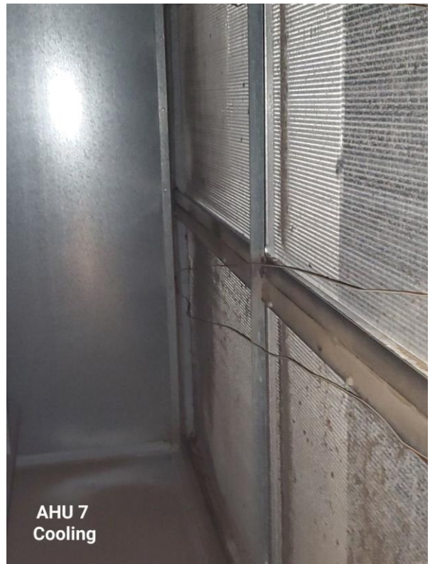
AHU-7 Cooling Coils
