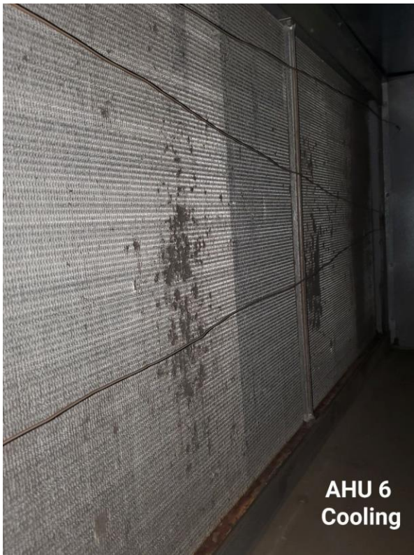
AHU-6 Cooling Coils
